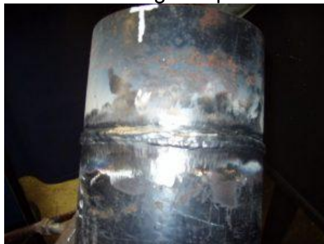
Last stringer filler bead before the completion of the weld.
