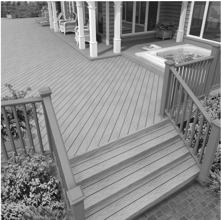
12.6 Decking application in North America (courtesy of Composatron).
