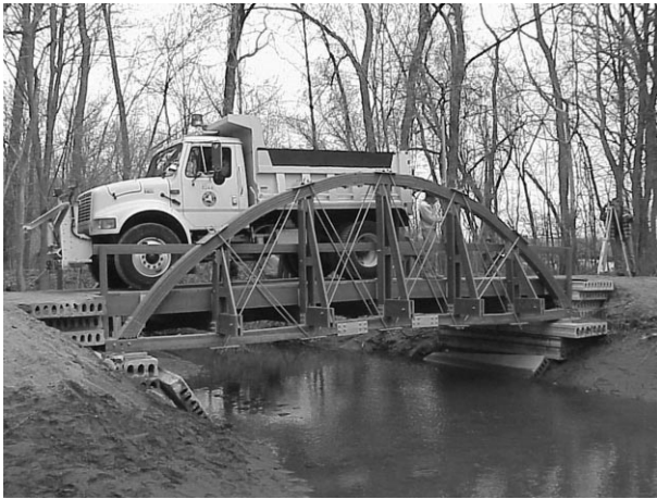
12.10 Reinforced plastic lumber bridge.
