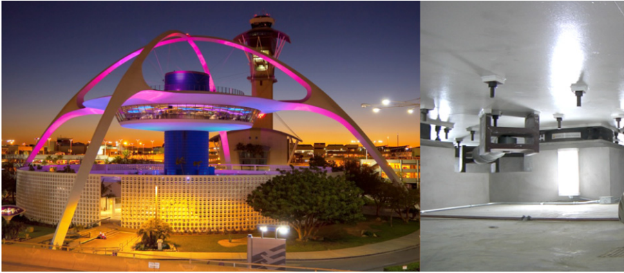
Figure 14.2 The LAX Theme Building (left), implemented damper and isolator (right).
