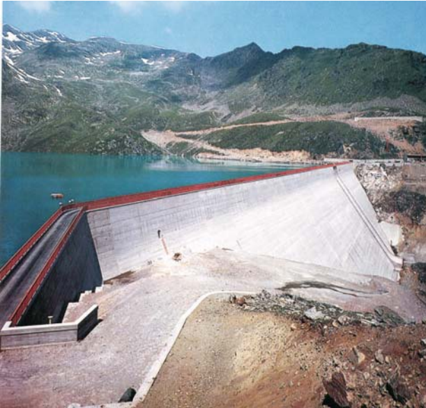
Fig. 35. The QUAIRA DELLA MINIERA dam near Bolzano, Italy [63]
