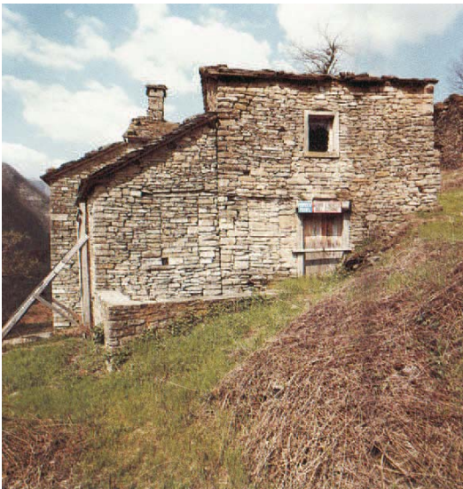
Fig. 115. Restoration of dry masonry farmhouses promoted by “Consorzio Acque per le Provincie di Forlì e Ravenna” (The Water Cooperate for the Provinces of Forlì and Ravenna) in the area of RIDRACOLI dam [54]
