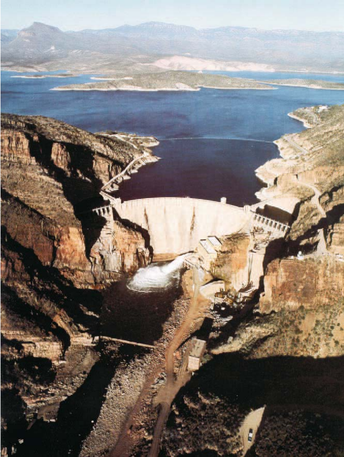
Fig. 5. The ROOSEVELT dam on the Salt River, Colorado, U.S.A. [136]
