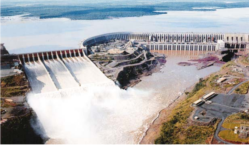
Fig. 121. The ITAIPU dam (earth: 17 \cdot 10^6 m^3 ; concrete: 12 \cdot 10^6 m^3 ) on the upper Paraná River at the Brazil-Paraguay border is the largest hydroelectric powerplant in the world (12,600 MW)
