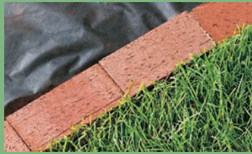
Brick set on faces parallel to the walkway edge
