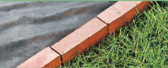
Brick set on faces perpendicular to the walkway edge
