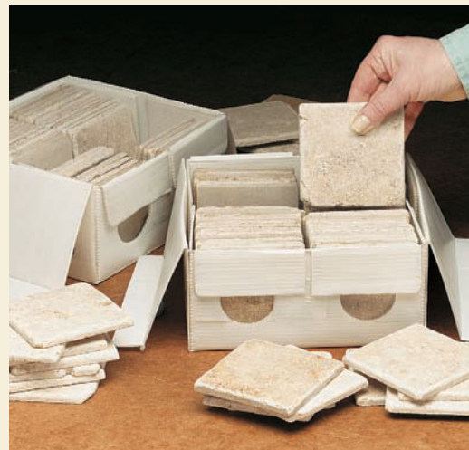
Mix tile from carton to carton. Slight variations in color won't be as noticeable mixed throughout the project as they would be if the color shifts from one area to another.
