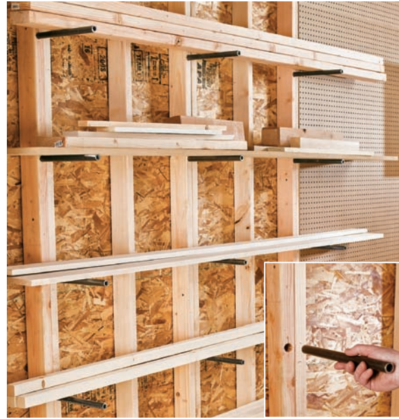
You can build this space-saving lumber rack with a few 2 × 4 studs and some steel pipe: drill matching holes in all of the studs, then fasten one to the side of every other garage-wall stud. Add a plywood shelf or two for storing small pieces. Don't use garage wall studs as the pipe supports; the holes would weaken the studs too much.
