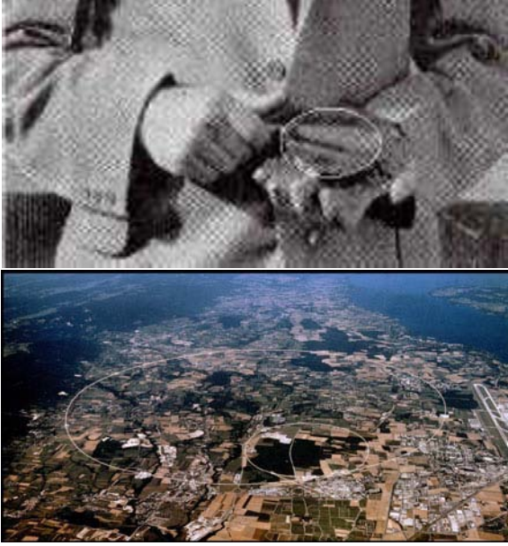
Figure 1. Top: First Cyclotron: 1930 E.O. Lawrence, 11 cm diameter, 1.1 MeV protons. Bottom: The LHC, 2008 9 km diameter, 7 TeV protons, after 80 years, 10^7 times more energy and 10^5 times larger
