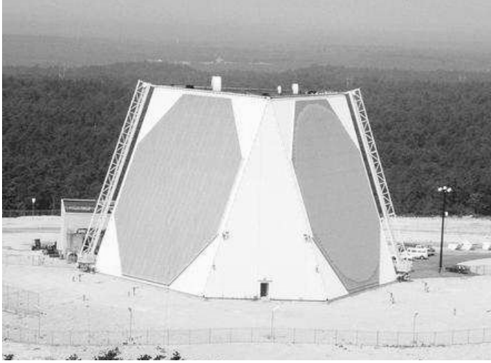
Fig. 2.25. Two-face phased array at Cape Cod, belonging to the US Space Surveillance Network (SSN) Phased Array Warning System (PAWS; source: SSN).
