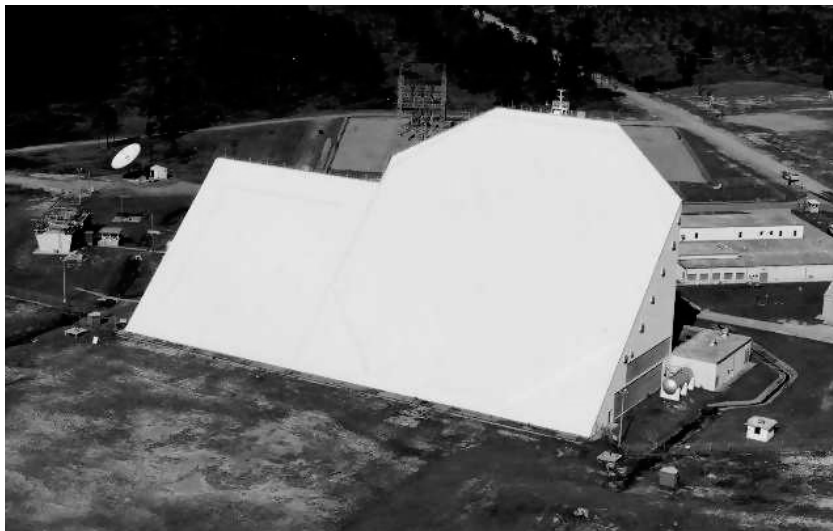
Fig. 2.27. One-face phased array at Eglin, with separate transmitter and receiver sub-arrays, belonging to the US Space Surveillance Network (source: NASA).
