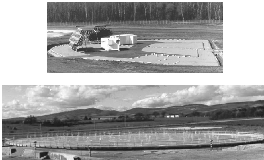
Fig. 2.29. The French electronic fence GRAVES (Grande Réseau Adapté à la Veille Spatial), with a transmitter, consisting of two phased arrays, at Dijon (top), and a receiver array at Apt (bottom; source: ONERA).
