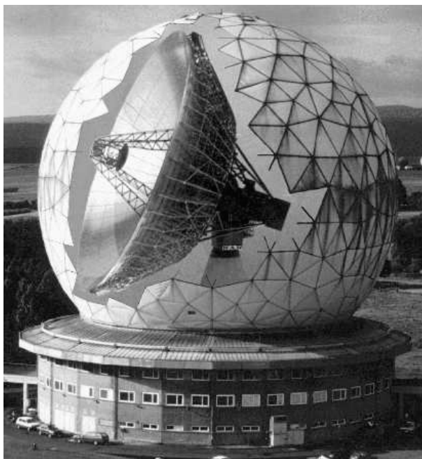
Fig. 2.30. FGAN Tracking and Imaging Radar (TIRA) at Wachtberg/Germany (artist's view, with partially removed radome; source: FGAN).
