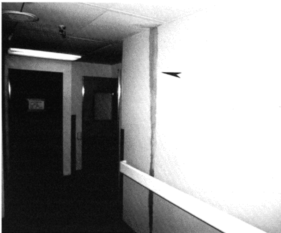
Fig. 3. Water being used for dust control during remediation on an upper floor wets a paper-fibre gypsum board wall, providing an opportunity for new colonization.
