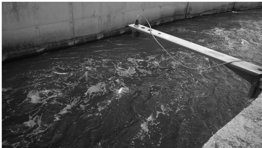
FIGURE 2.2 Discharge measurement at the outlet of the Tatlar WWTP by an ultrasonic displacement meter.
