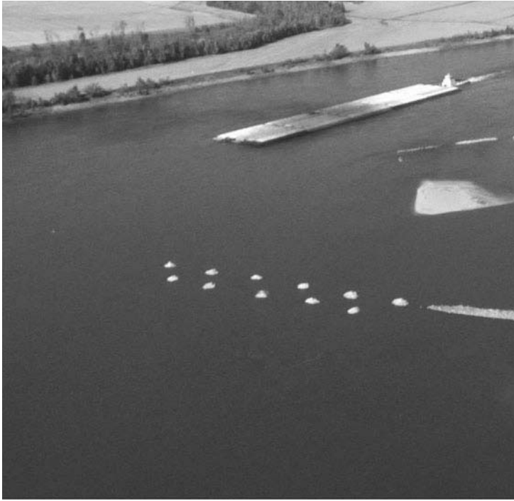
Fig. 10-2. Double row of multiple roundpoint structures on the Mississippi River
