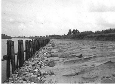
Fig. 6-4. Pile revetment on the Red River in Louisiana immediately after construction (a) and after sediment deposition had occurred (b)
