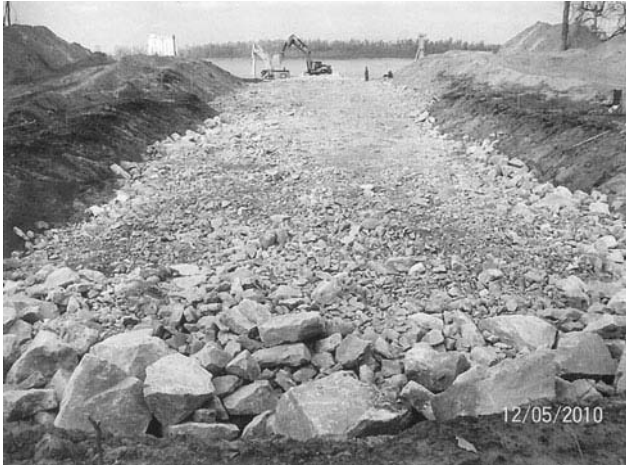
Fig. 5-6. Stone placed in stone root on the Mississippi River Source: USACE Vicksburg District
