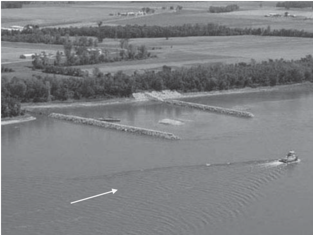
Fig. 5-7. Dike bank paving on the upper Mississippi River Source: USACE St. Louis District
