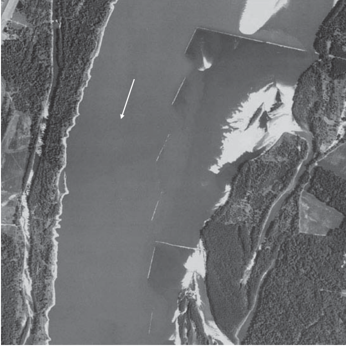
Fig. 5-11. Vane dikes between L-head dikes on the Mississippi River near Providence, Louisiana
