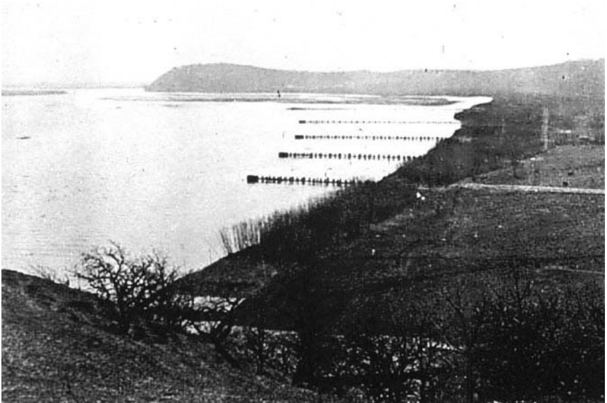
Fig. 5-20. Rock Bluff Bend, Missouri River, with timber-pile dikes, March 1935
