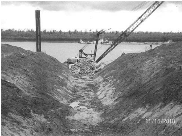
Fig. 5-5. Excavated trench for stone root on the Mississippi River Source: USACE Vicksburg District
