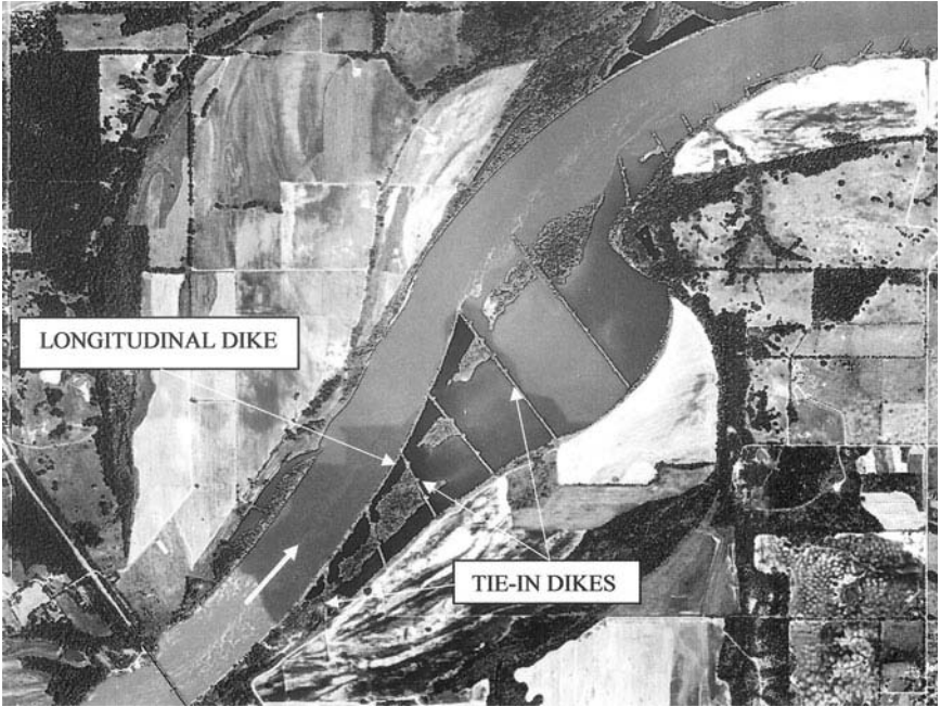
Fig. 5-9. Longitudinal dike on the Arkansas River Source: USACE Little Rock District
