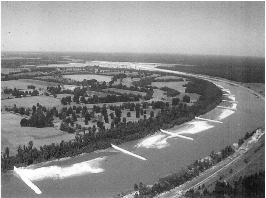
Fig. 4-3. Additional contraction structures Source: USACE Vicksburg District
