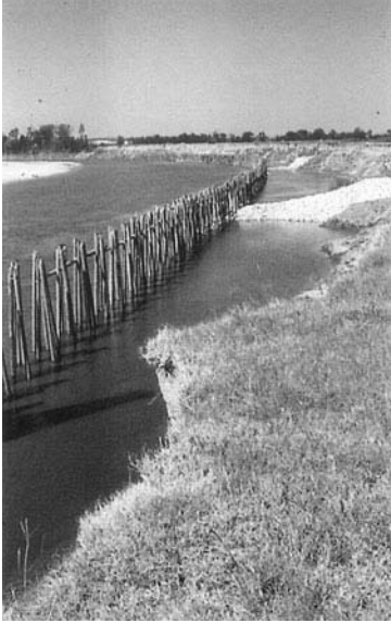
Fig. 6-4. Pile revetment on the Red River in Louisiana immediately after construction (a) and after sediment deposition had occurred (b)
