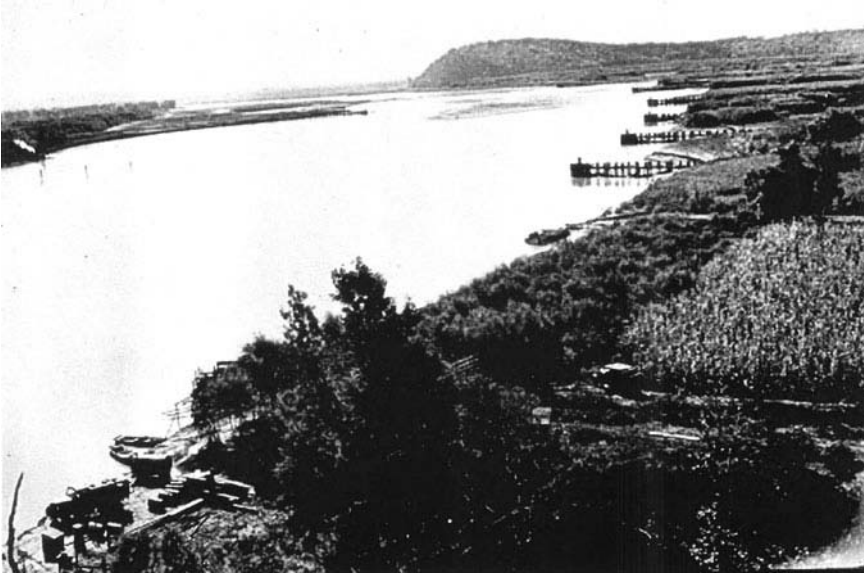
Fig. 5-21. Rock Bluff Bend, Missouri River, showing deposition in timber-pile dike field, October 1939
