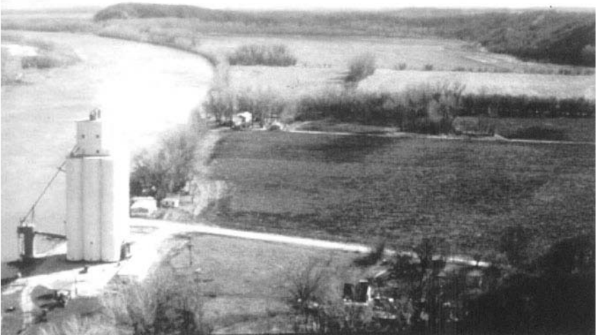
Fig. 5-24. Conditions at Rock Bluff Bend, Missouri River, March 1983 Source: USACE Omaha District
