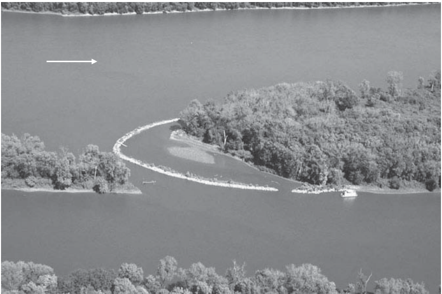
Fig. 7-4. Bullnose structure on the Mississippi River Source: USACE St. Louis District
