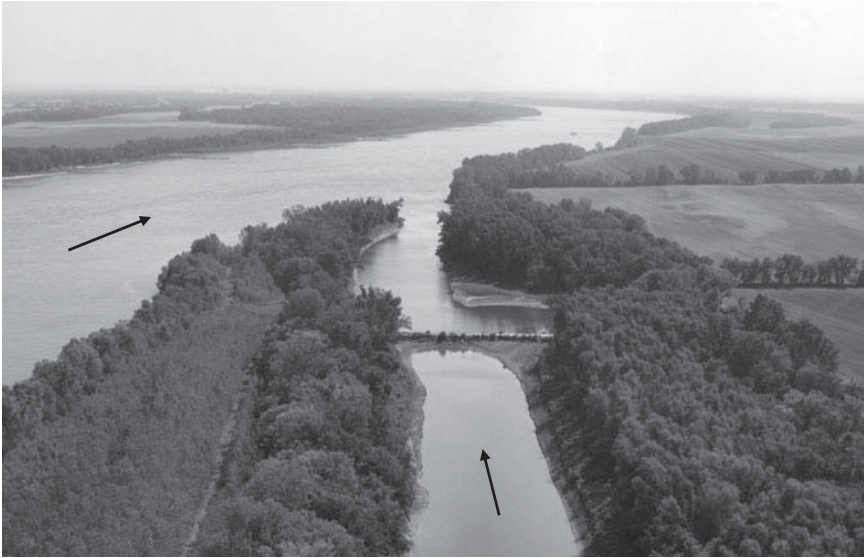
Fig. 5-13. Looking downstream at a closure dike on a secondary channel on the Mississippi River. Note the widened bankline just below the dike caused by the plunge pool when the dike is overtopped Source: USACE St. Louis District
