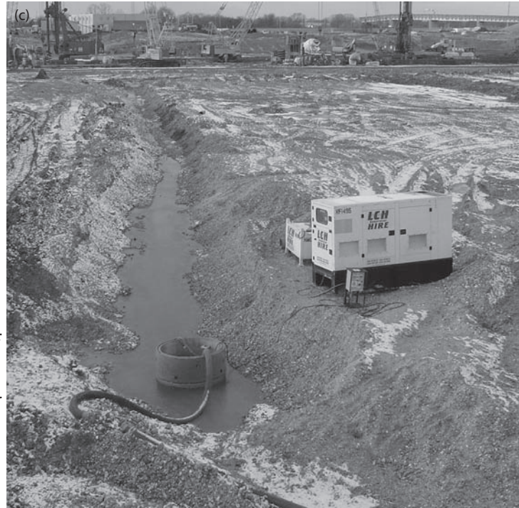
Figure 8.2 Typical forms of sump construction. (a) Small sump formed using perforated oil drums. (b) Large sump formed using concrete manhole rings. (c) Concrete manhole ring sump fed by a drainage ditch. (Courtesy of WJ Groundwater Limited, Bushey, U.K.)
