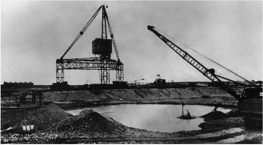
Figure 4.10 Perched water table. The groundwater level monitored in observation wells was several meters below the standing water visible in the photograph. When the clay layers below this level were punctured by excavating, the perched water drained away. (Courtesy of ESG Soil Mechanics, Burton on Trent, U.K.)
