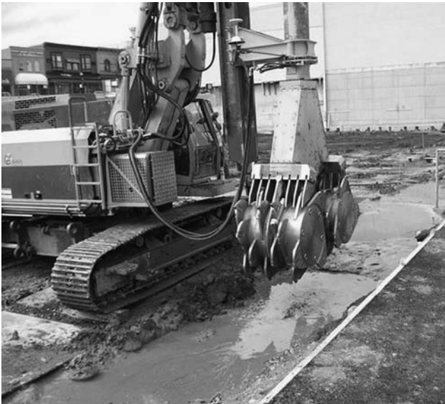
Figure 12.20 CSM unit. (Courtesy of Golder Associates, Toronto, ON, Canada.)
