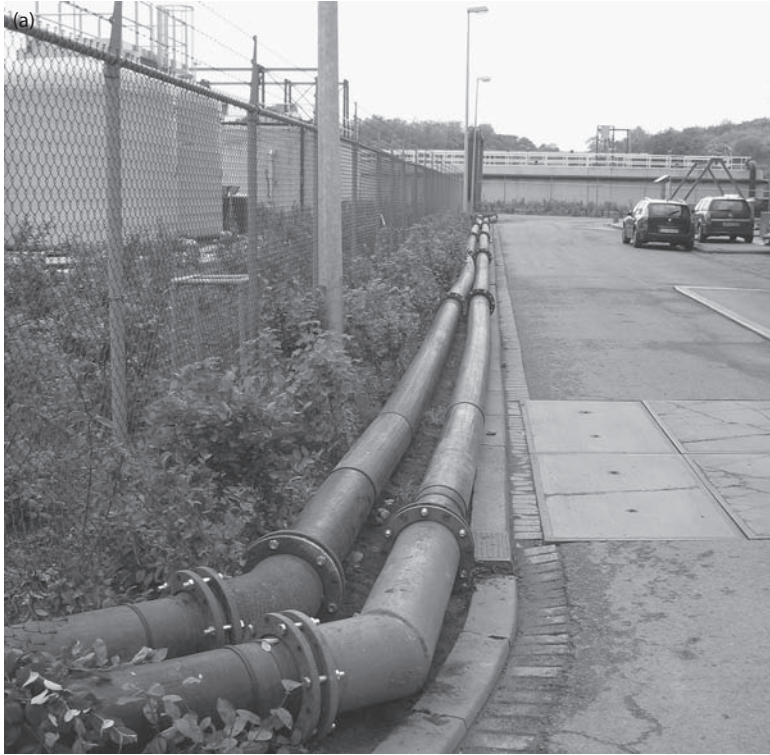
Figure 13.10 Pipework used for dewatering discharges. (a) Sectional pipework used for dewatering discharge systems. (b) Pipe bridge used to carry dewatering discharge over access road. (Courtesy of Theo van Velzen BV, Heiloo, The Netherlands.)
