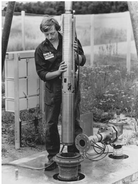
Figure 13.6 Lowering borehole electro-submersible pump and riser into the well. (Courtesy of Grundfos A/S, Bjerringbro, Denmark.)
