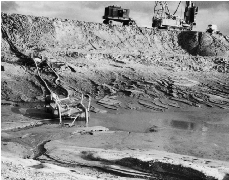
Figure 8.6 Outwash fans due to sump pumping. The suction hoses for the sump pumps were mounted on the crude pontoon shown on the left of the photograph. This helped pumping continue as the water level within the excavation varied with the tide.
