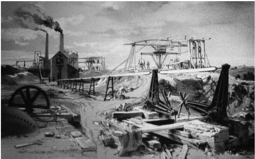
Figure 2.2 Pumps for draining the Kilsby Tunnel. A pumping well is shown in the foreground, with the steam pumphouse in the distance. (From Bourne, J.C., Drawings of the London and Birmingham Railway . Collection of the Library of the Institution of Civil Engineers, London. Courtesy of the Institution of Civil Engineers.)
