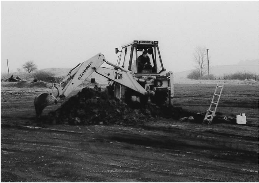
Figure 6.2 Trial pitting using a mechanical excavator.
