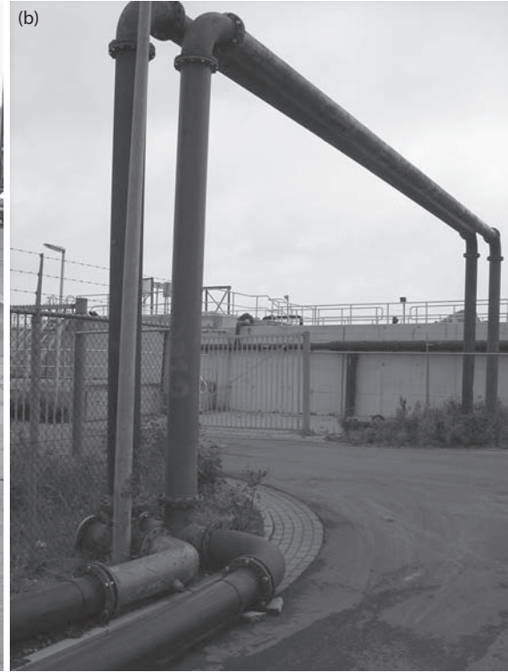
Figure 13.10 Pipework used for dewatering discharges. (a) Sectional pipework used for dewatering discharge systems. (b) Pipe bridge used to carry dewatering discharge over access road. (Courtesy of Theo van Velzen BV, Heiloo, The Netherlands.)
