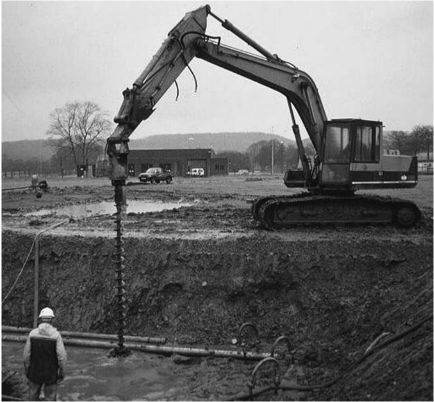
Figure 9.12 Hydraulic auger attachment for preboring through cohesive strata. (Courtesy of WJ Groundwater Limited, Bushey, U.K.)
