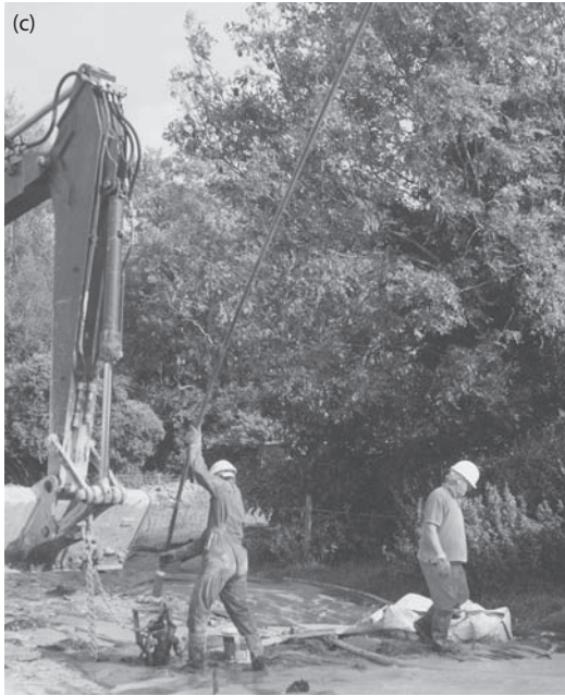
Figure 9.9 (Continued) (c) Plastic disposable wellpoint is installed. (Courtesy of Dewatering Services Limited, Sandbach, U.K.)
