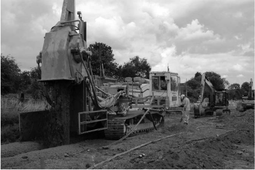
Figure 12.21 Mix-in-place barrier installed by trencher. (Courtesy of Bachy Soletanche, Burscough, U.K.)
