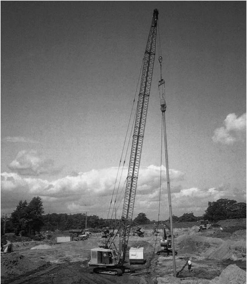
Figure 10.6 Holepuncher used for installation of deep wells. (Courtesy of T.O.L. Roberts.)
