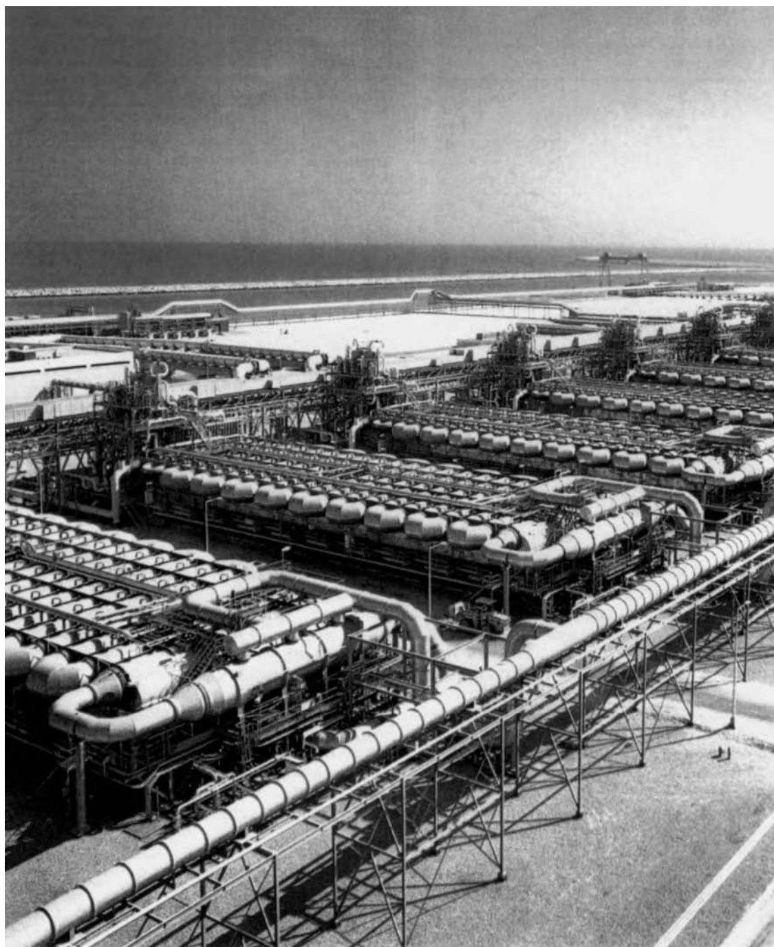
FIGURE 1 Panoramic view of the Al-Jubail Saudi Arabia, phase II, MSF desalination plant. It is up to now the World largest desalination installation totaling a capacity of 947,000 m 3 /d (250 Mgd) fresh water production. Each unit has a capacity of 23,500 m 3 /d (6.2 Mgd). The plant was built for the Saline Water Conversion Corporation, of Saudi Arabia by the Japanese Companies of Sasakura and Mitsubishi. (Courtesy Sasakura Engineering Co., Japan)
