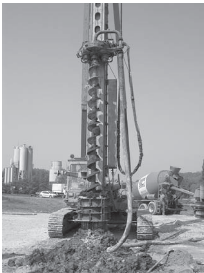
Figure 1. KELLER FOUNDATIONS—Column P1.
