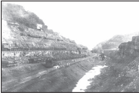
Figure 2. Panama Canal: excavation work using trains in the deep Gaillard Cut, 1911.
