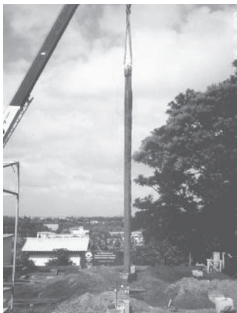
Figure 5. Extracted pile.
