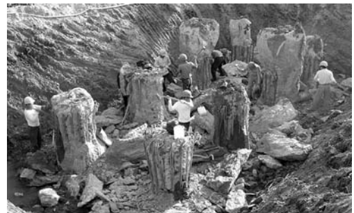
Figure 13. Chipping off the pile heads.
