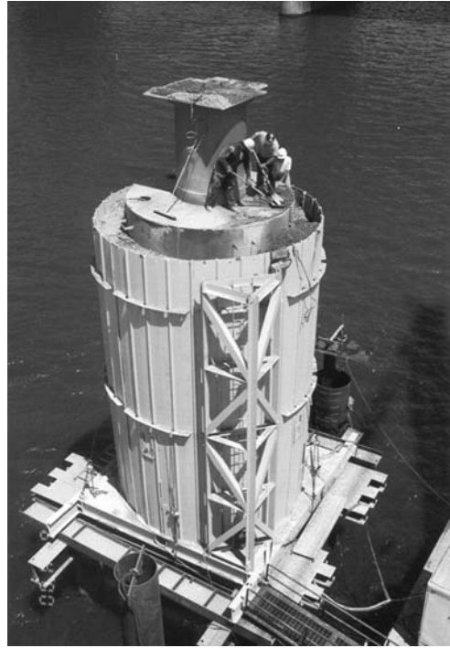
Figure 20. Statnamic axial load test set up.
