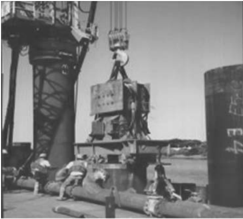
Figure 14. Installation of permanent casing.
