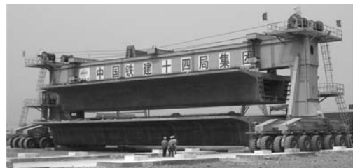
Figure 1. Precast box beam during dismantling from formwork.
