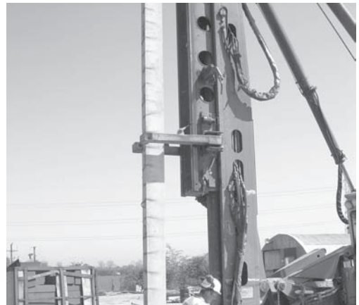
Figure 3. Driving of precast concrete energy piles.
