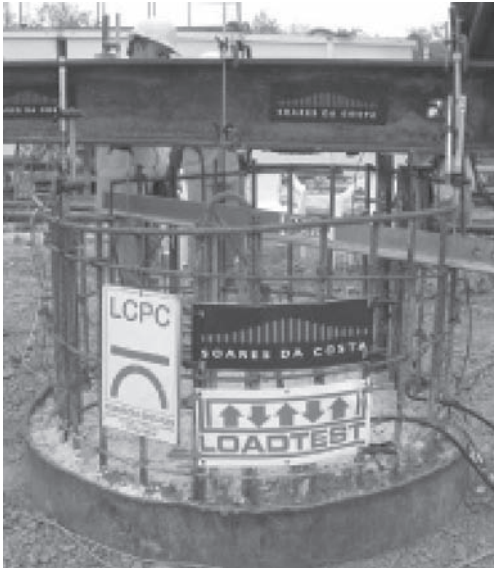
Figure 7. Pile Head with instrumentations.
