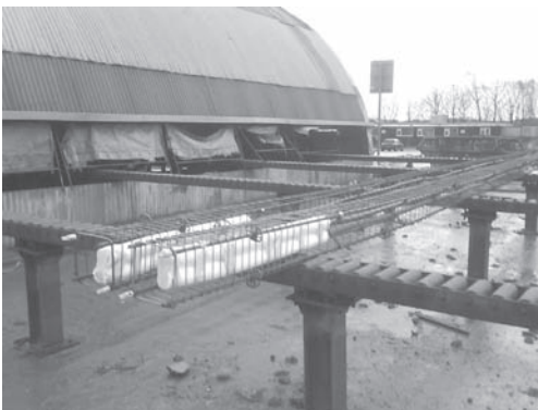
Figure 2. Heads of precast energy piles before casting.
