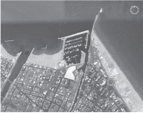
Figure 1. Site location of the new residential and business centre “La prua”, Rimini—aerial view.
