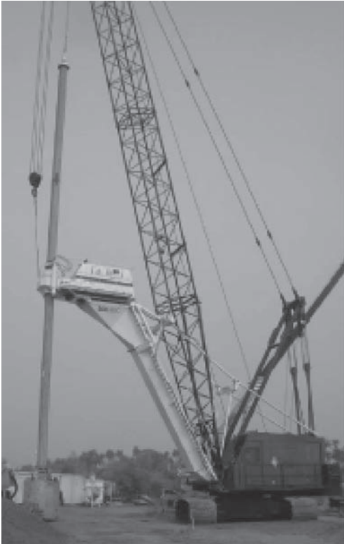
Figure 1. Link Belt LS-418 with Soilmec RT3-ST.
