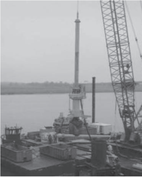
Figure 4. Fly drill operating in Kelly mode, Victory Bridge, New Jersey.
