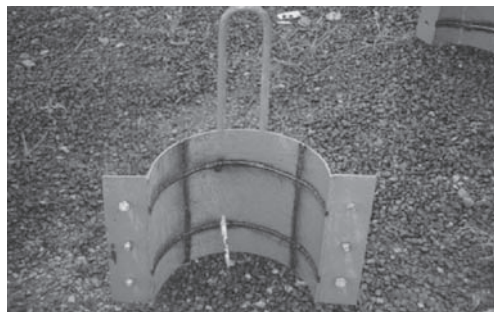
Figure 4. Arrangement to fix the pile.
