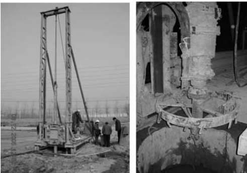
Figure 11. Direct rotary flush drilling with vane cutter \varnothing 1,0 m.
