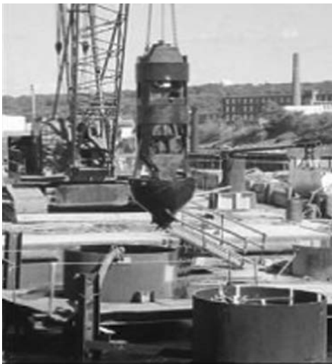
Figure 7. Example of hammergrab.
