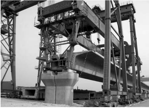
Figure 2. Bridge pier. Installation of box beams.
