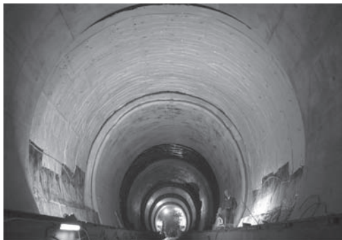
Figure 5. Energy geotextile at lot LT22 of the Lainzer tunnel.
