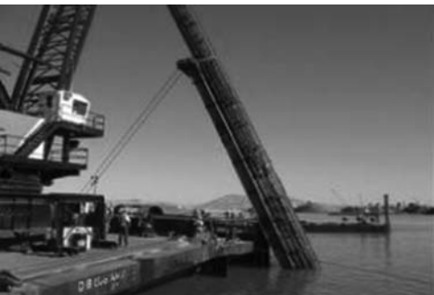
Figure 17. Temporary tipping frame to support reinforcing cage on batter.
