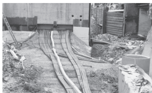
Figure 2. Absorber pipes and measurement cables.
