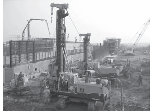
Figure 2. Site set up.
