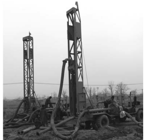
Figure 12. Suction drill rigs.
