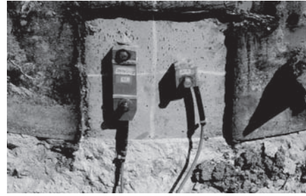
Figure 34. Detail of the dynamic instrumentation (at left: extensometer; at right: accelerometer).
