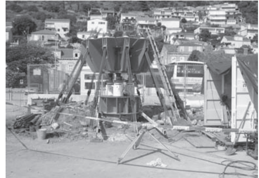
Figure 3. Axial static load test on the pile TP-V1.
