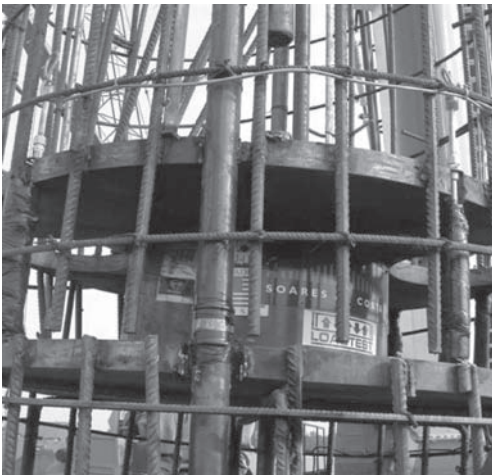
Figure 2. The reinforcing cage with the O-cell.
