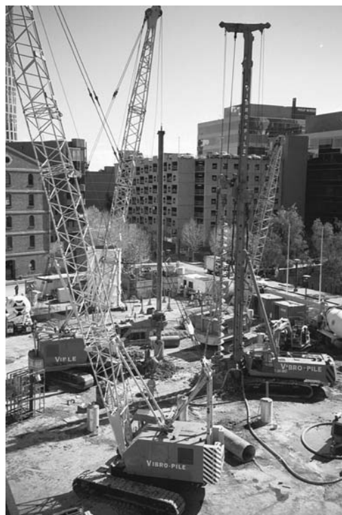
Figure 4. Site congestion was a major concern.
