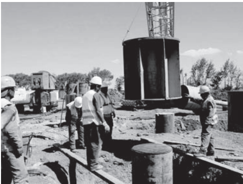
Figure 33. Placement of the reducer over a \phi 800 mm-pile.
