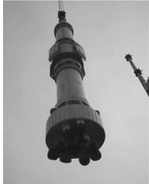
Figure 5. Fly drill in RCD mode, Victory Bridge, New Jersey.
