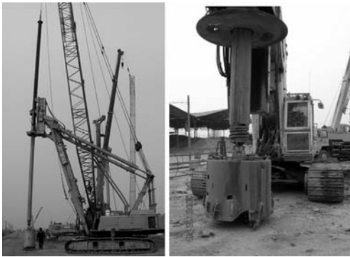
Figure 10. Dry rotary drilling with drill bucket.
