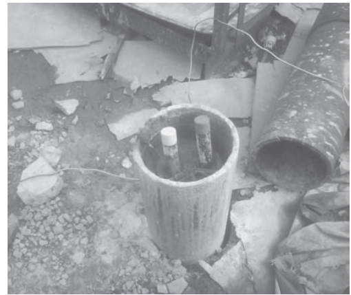
Figure 4. Driven steel energy pile.
