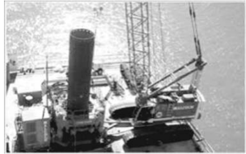
Figure 15. Oscillator equipment installing segmental casing.
