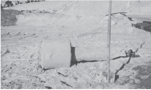
Figure 14. Exhumed enlarged base of bored pile in Perth Sand.
