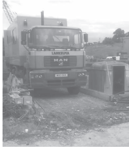
Figure 5. Coaxial pipe being installed.
