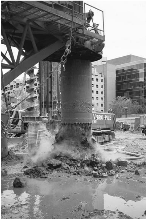
Figure 5. Coring of basalt.
