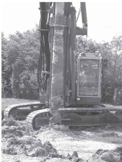
Figure 2. MENARD SOLTRAITEMENT—Column P2.
