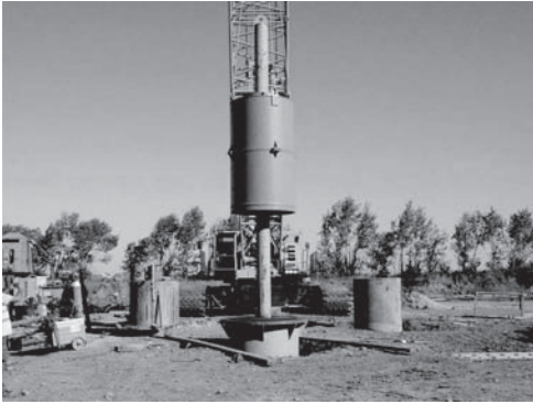
Figure 32. SIPEX—Impact system for experimental piles.
