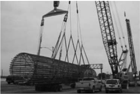
Figure 16. Lifting large reinforcing cage.
