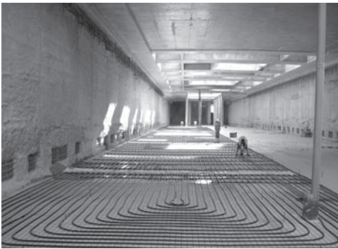
Figure 7. Base slab of station “U2/4 Messe” equipped with absorber pipes.
