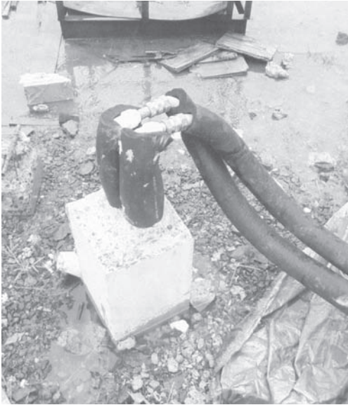
Figure 7. Thermal test on concrete pile.
