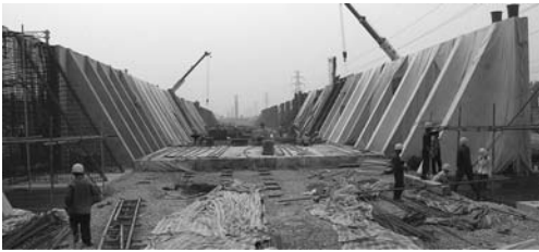
Figure 3. Angular retaining wall (earth structure).
