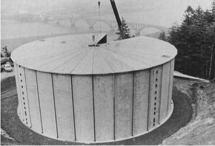
Precast concrete liquid storage tank, Gold Beach, Oregon. (Courtesy Prestressed Concrete Institute, Chicago.)
