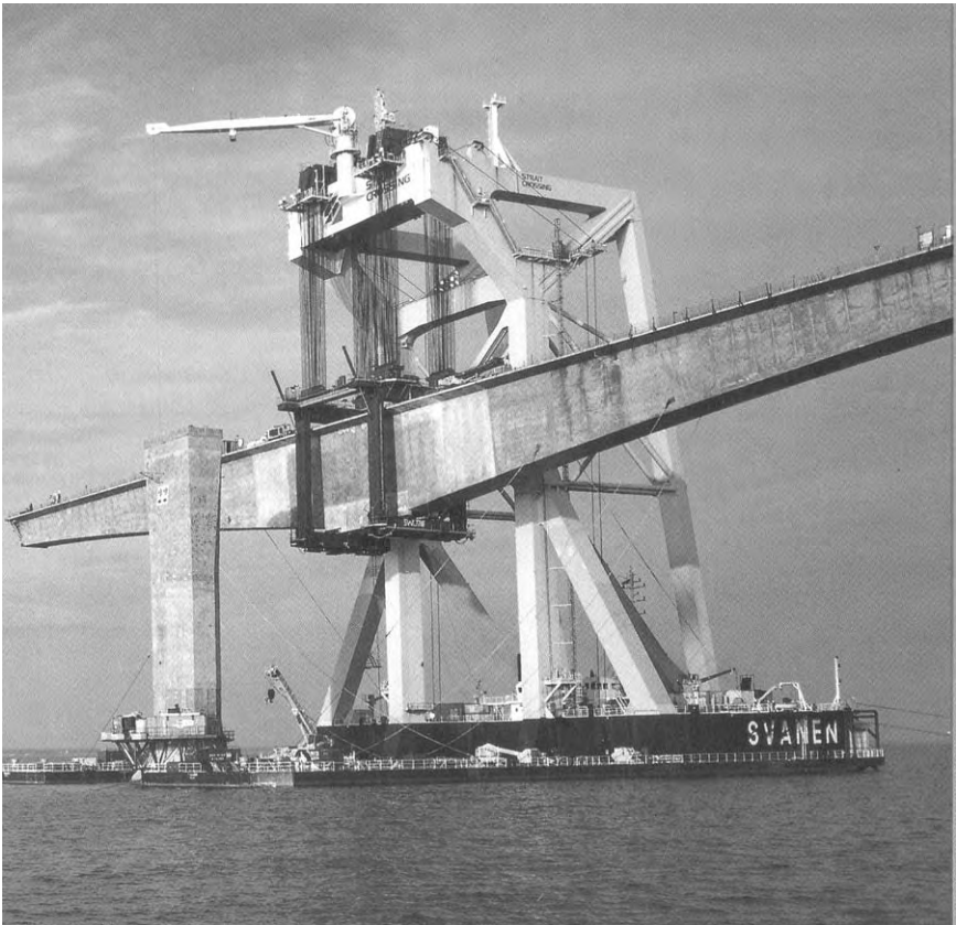
The Confederation Bridge connecting Prince Edward Island and New Brunswick, Canada: Floating crane installing a 190m long segment on a pier
