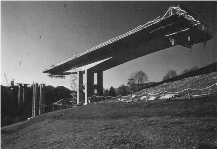
Cast in situ segmental construction of 'Pont de la Fégère', near Lausanne, Switzerland.
