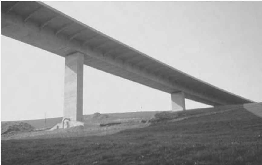
Viaduct at Gruyère, Switzerland
