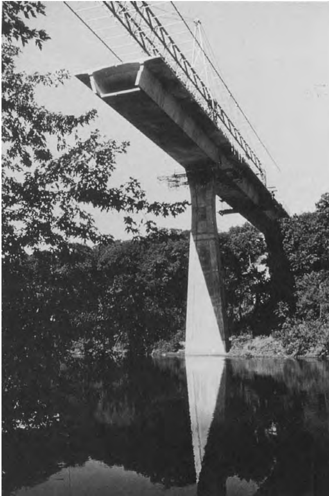
Post-tensioned precast segmental bridge erected by means of a launching truss, Kishwaukee River, Illinois. (Courtesy Prestressed Concrete Institute, Chicago.)
