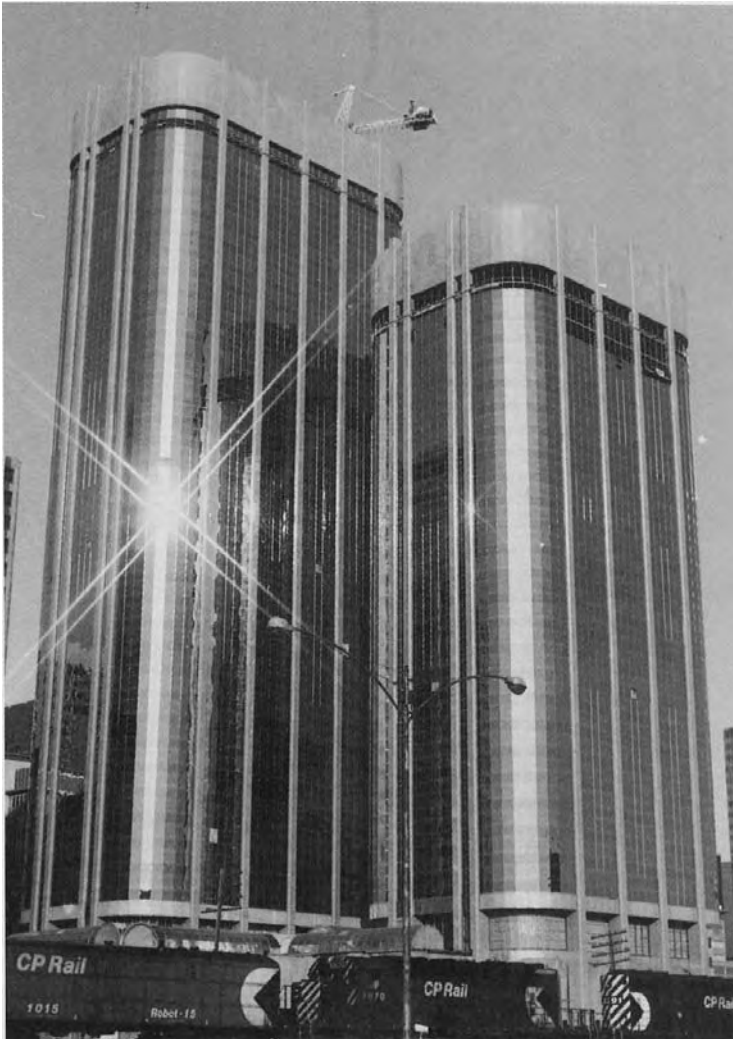
Western Canadian Place, Calgary. Partial prestressing used in all floors. (Courtesy Cohos Evamy & Partners, Calgary.)
