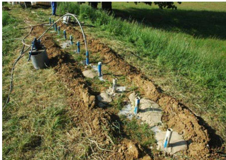
Fig. 3 Pressure filling of the holes using clay mixtures [1]
