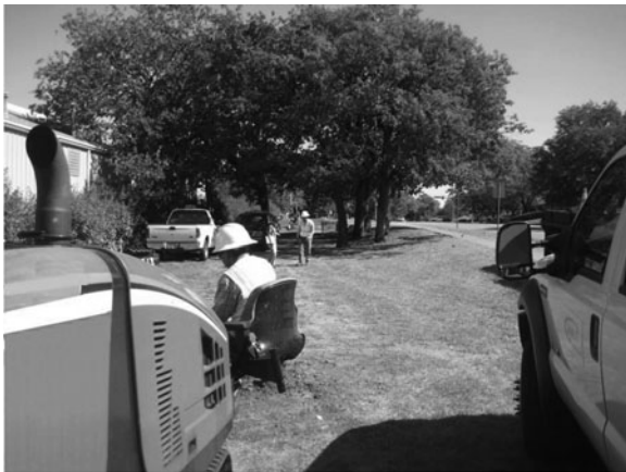
Figure 6-4. Initial Pilot Hole Boring with Mini-HDD Machine.
