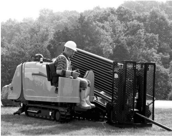
Figure 3-16. Mini-Horizontal Directional Drilling Machine (Courtesy of Astec Industries).
