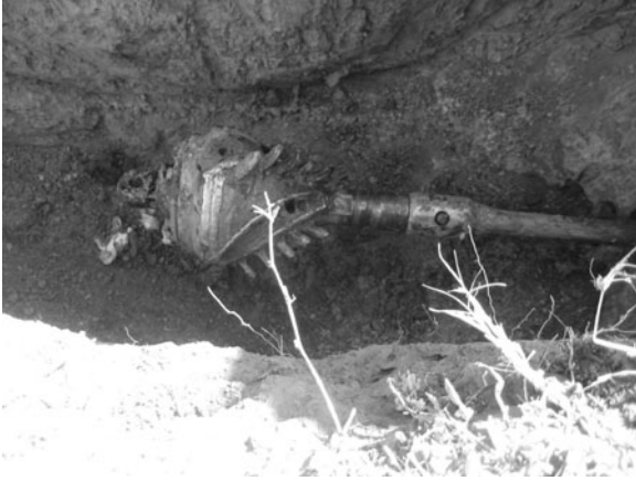
Figure 6-5. Reamer Connected to Drill String.
