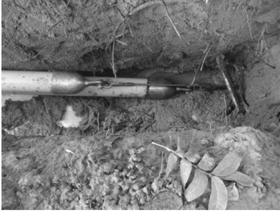
Figure 6-7. Pullback of Two BCN Conduits.
