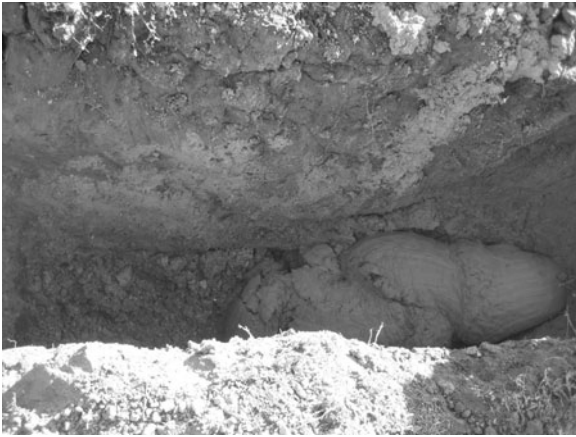
Figure 6-6. Purging Expanded Borehole of Cuttings.
