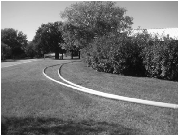
Figure 6-2. Completed Length of Field-Fused PVC Pipe.
