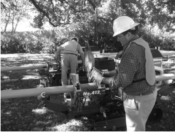
Figure 6-1. Field Assembly Operation for Field-Fused PVC Pipe.
