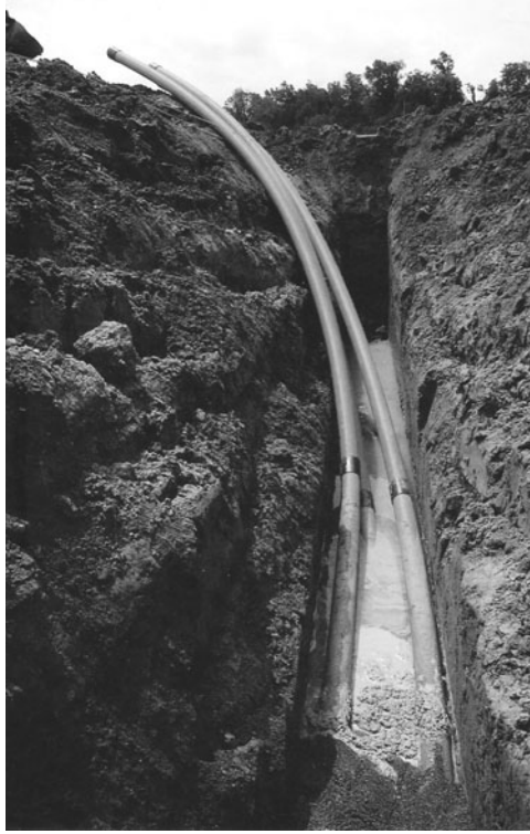
Figure 2-8. HDPE Corrugated Exterior, Smooth-Wall Interior Conduit (Courtesy of A-D Technologies).
