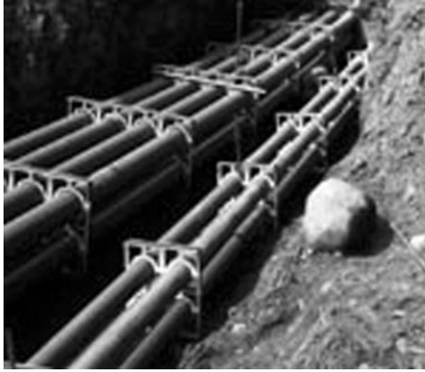
Figure 2-1. Underground PVC Conduit System (Courtesy of Prime Conduit).
