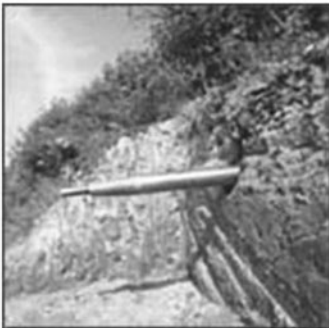
Figure 3-14. Use of a Pneumatic Piercing Tool (Courtesy of Allied Construction Products, LLC).
