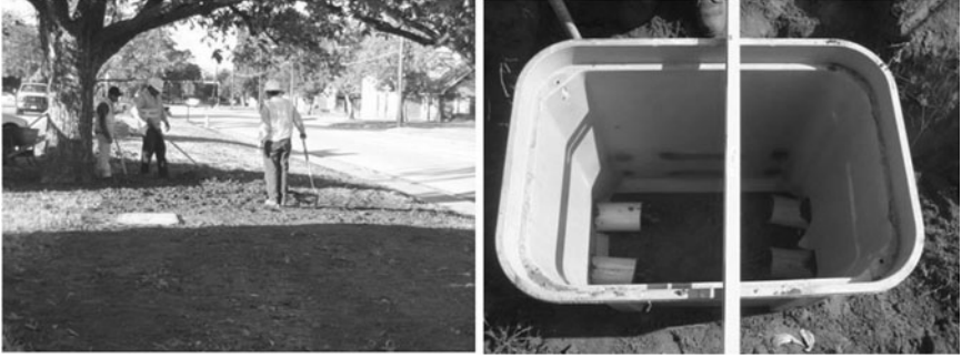
Figure 6-15. Installed Handhole (With and Without Cover), South Davis Drive.
