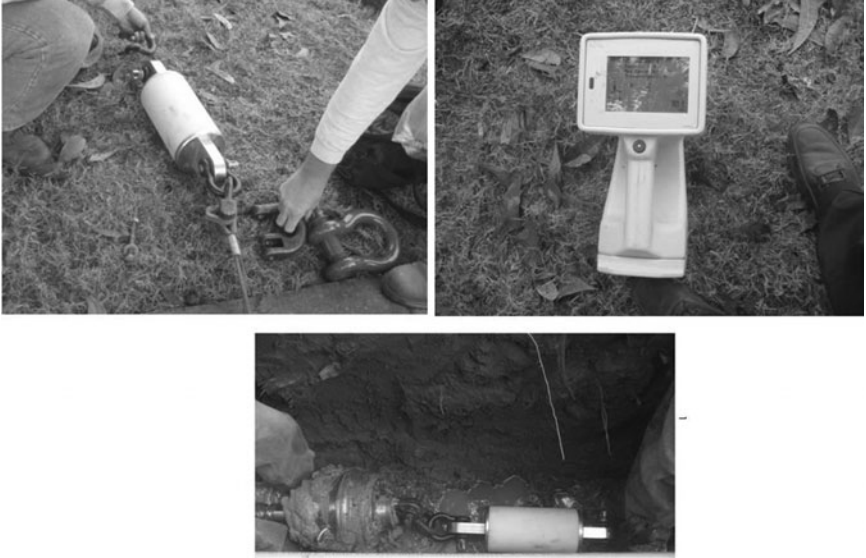
Figure 6-9. Tension and Pressure Monitoring System for HDD Operation.
