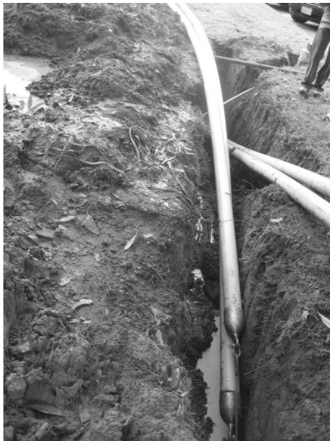
Figure 6-8. Overlapping Conduits from Adjacent Pullbacks.
