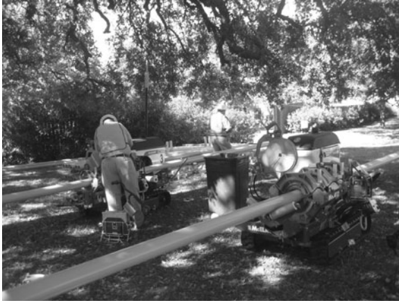
Figure 2-6. Field-Fused PVC.
