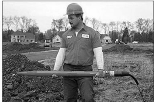
Figure 3-14. Use of a Pneumatic Piercing Tool (Courtesy of Allied Construction Products, LLC).
