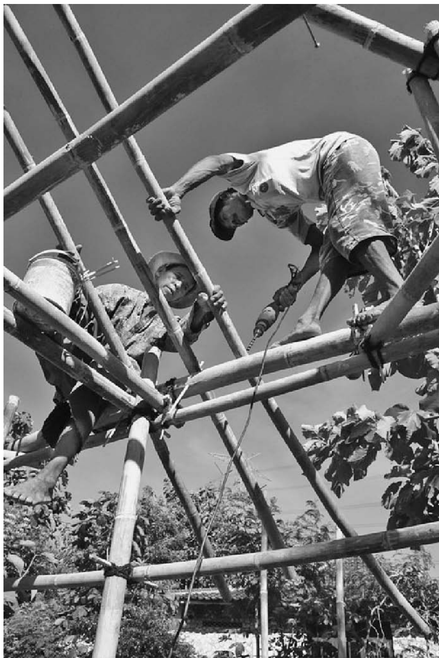
The post earthquake community construction of a house in South Jogyakarta. (Photo credit, Rikki Zulkernaen.)
