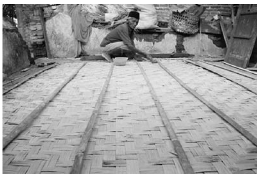
Preparing a bamboo thatch wall. (Photo credit, Eko Bhirwo.)
