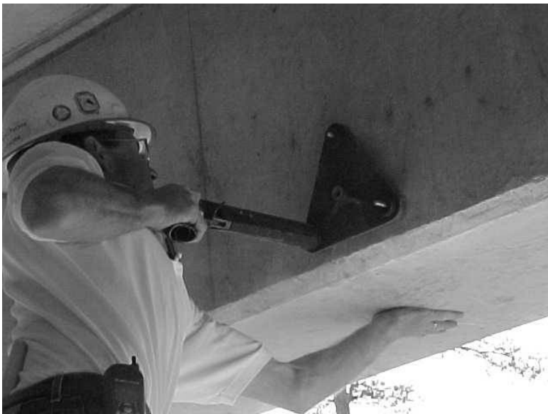
4.10 Windsor Probe™ determination on a beam using the three-probe template.
