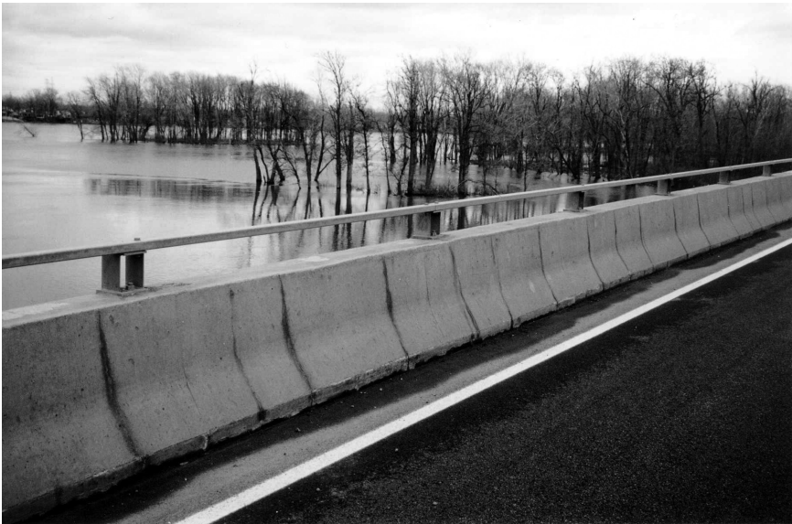
12.12 Barrier wall of Vachon bridge in Laval (Québec), Canada, after reconstruction.
