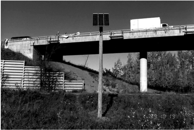
12.8 CNR bridge near Renfrew (Ontario), Canada, during repair and instrumentation.
