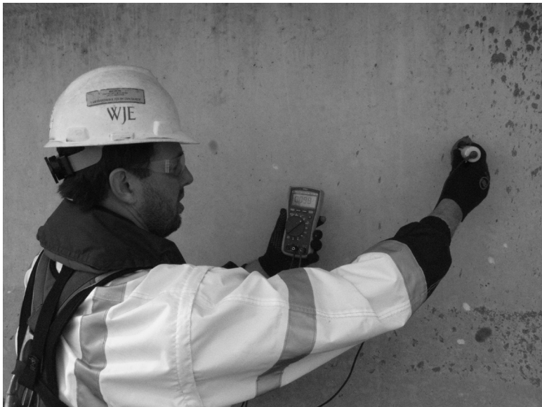
3.10 Copper–copper sulfate half-cell in use; note the sponge to keep the concrete moist and complete the circuit. (Courtesy of WJE)
