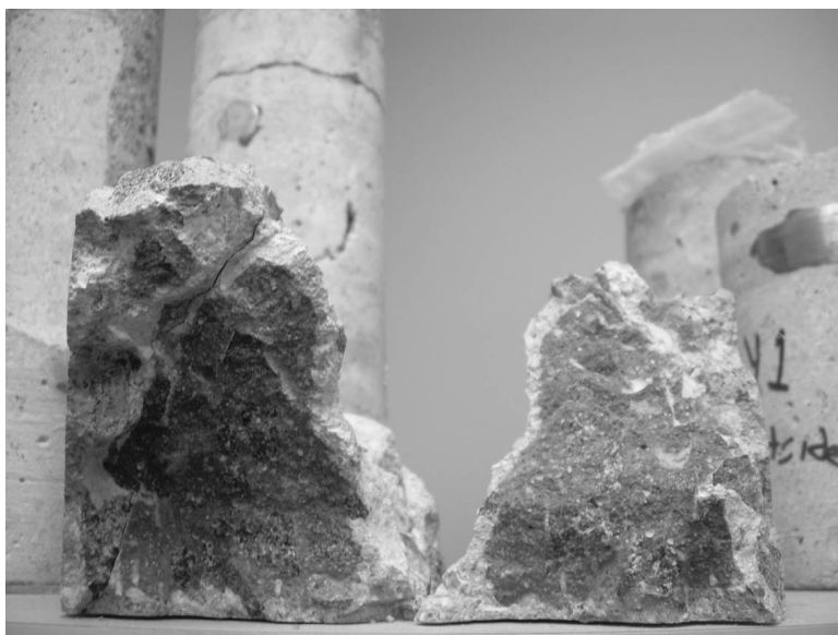
4.16 Carbonation testing on a column corner.
