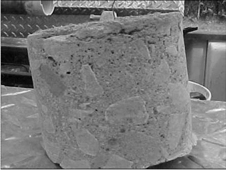
4.1 Delamination in a concrete core removed from a slab.
