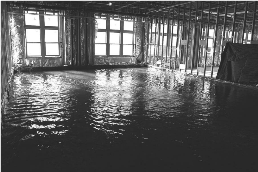
4.37 Use of water as load test material.
