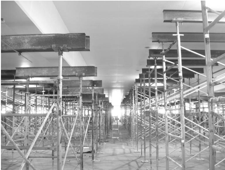
4.32 Shoring installed below structure for load testing.
