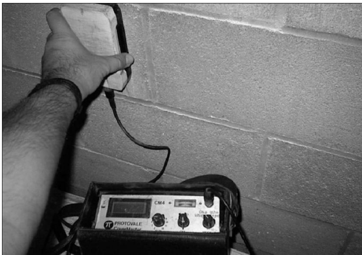
4.20 A covermeter used in locating reinforcing steel in concrete masonry unit.
