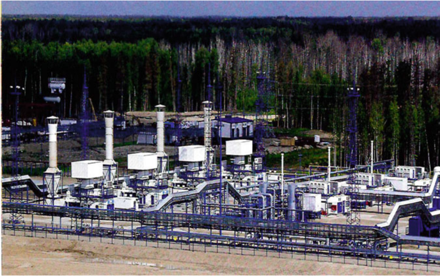
Fig. 4.7 Gas turbine power plant using associated gas (capacity of 24 MW, owned by “Gazpromneft-Vostok”, Russia)
