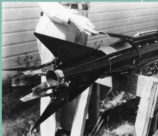
The gyroscope in this 1930s Goddard rocket ( left ) helped keep it on a straight course by operating movable vanes ( right ) in the rocket's exhaust.
