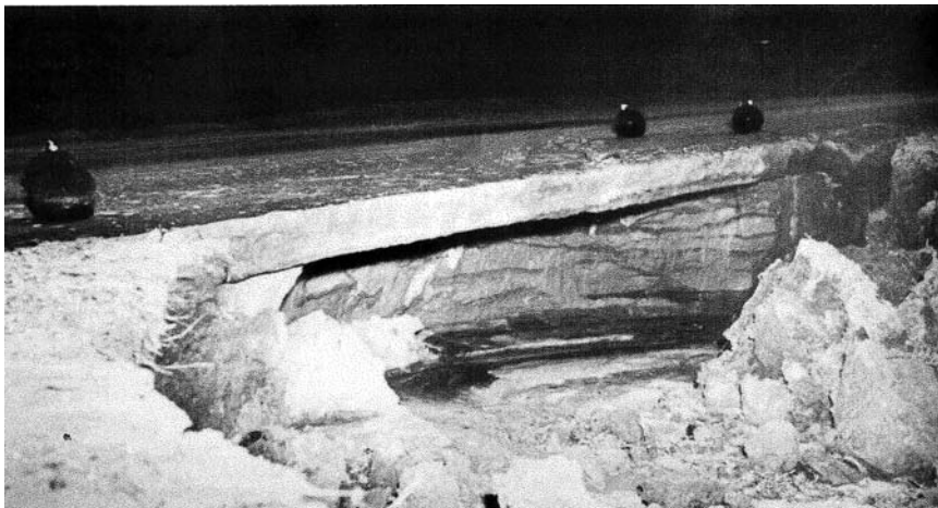
FIGURE 6.1 Bridging action of soil-cement road surface.
