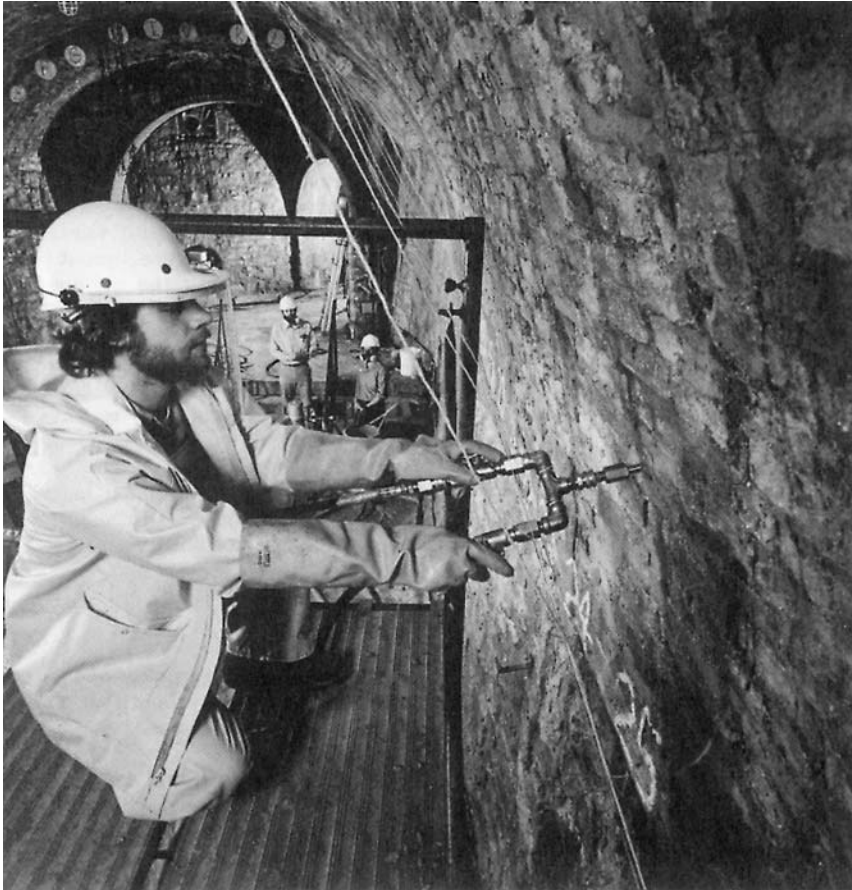
FIGURE 16.9 Grouting from the inside of a tunnel.
