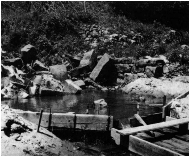
FIGURE 10.1 Weir to measure seepage downstream of power dam.
