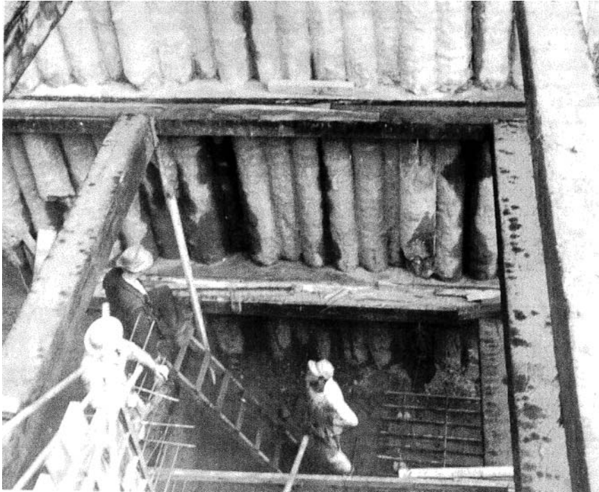
FIGURE 6.2 Earliest field work with deep soil mixing.
