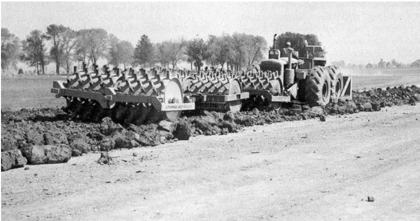
FIGURE 3.3 Sheepsfoot and rubber tired rollers.
