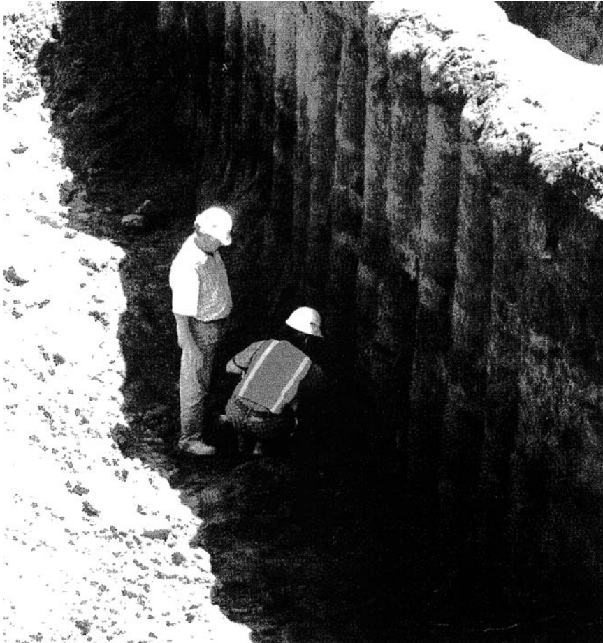
FIGURE 6.3 Barrier wall constructed by deep soil mixing, using a lime-cement slurry. (Courtesy of Underpinning and Foundation, SKANSKA, Maspeth, NY.)
