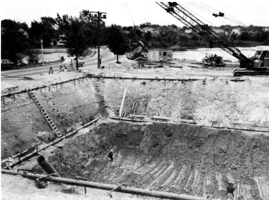
FIGURE 4.8 Wellpoint system in operation.
