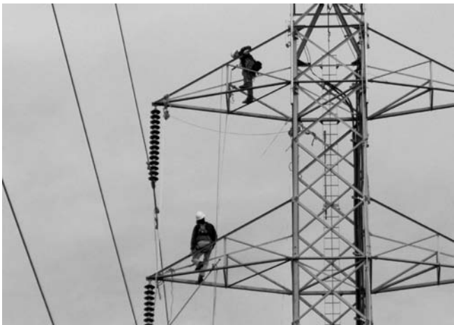
FIGURE 1.4 A transmission line that is being upgraded.
