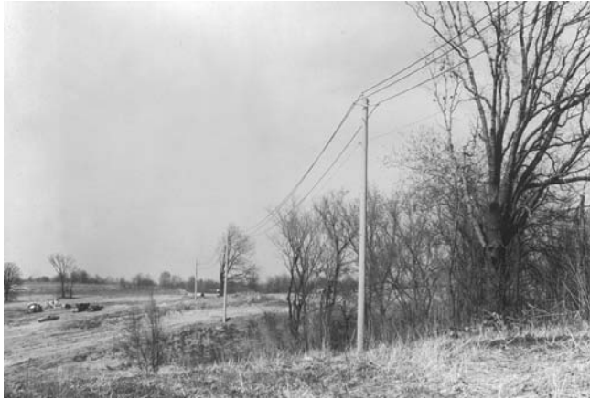
FIGURE 2.23 A typical 12.47-kV line with a single circuit and wood pole. It has a newer type pole top construction. (Union Electric Company.)
