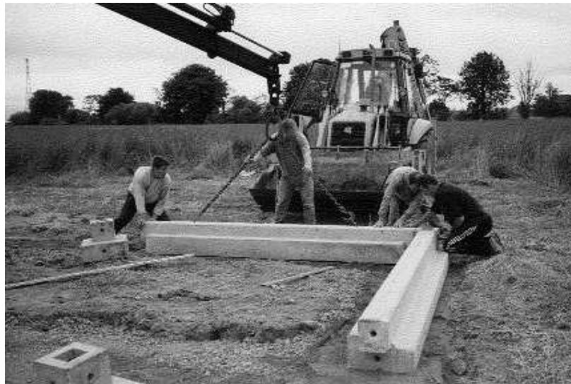
Figure 7 Modular foundation being installed at experimental site
