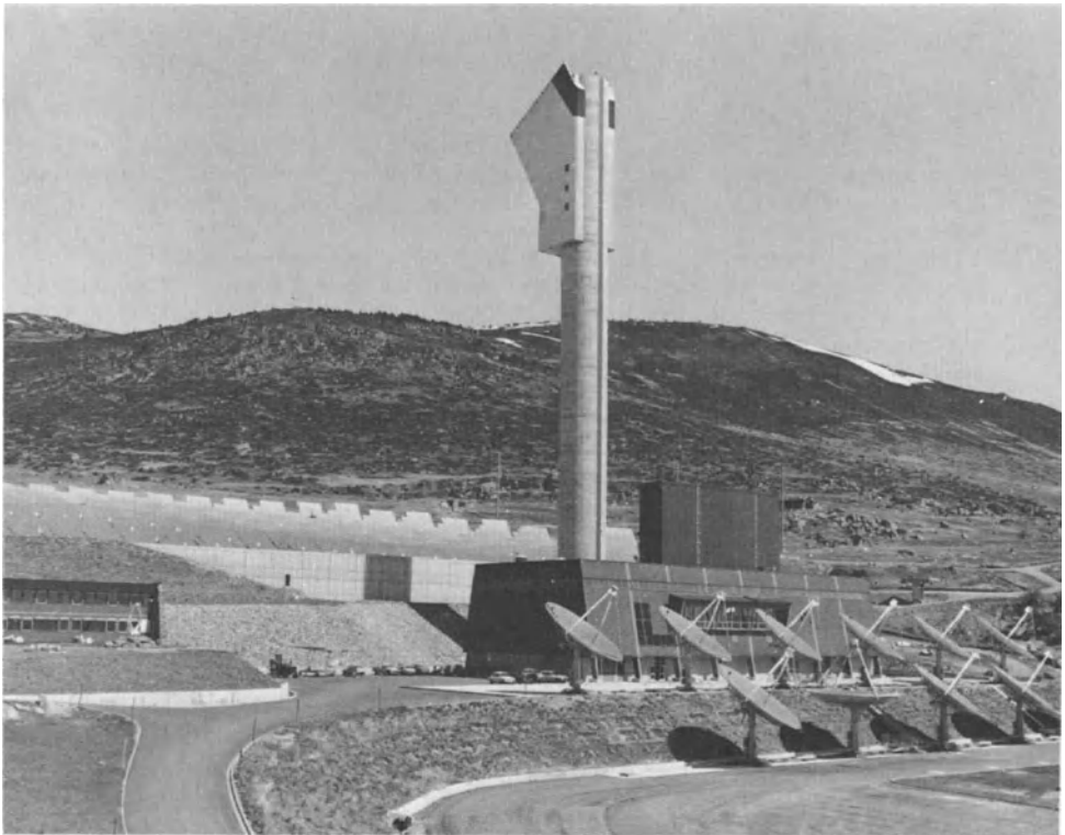
Figure 6 Auxiliary parabolic dishes
