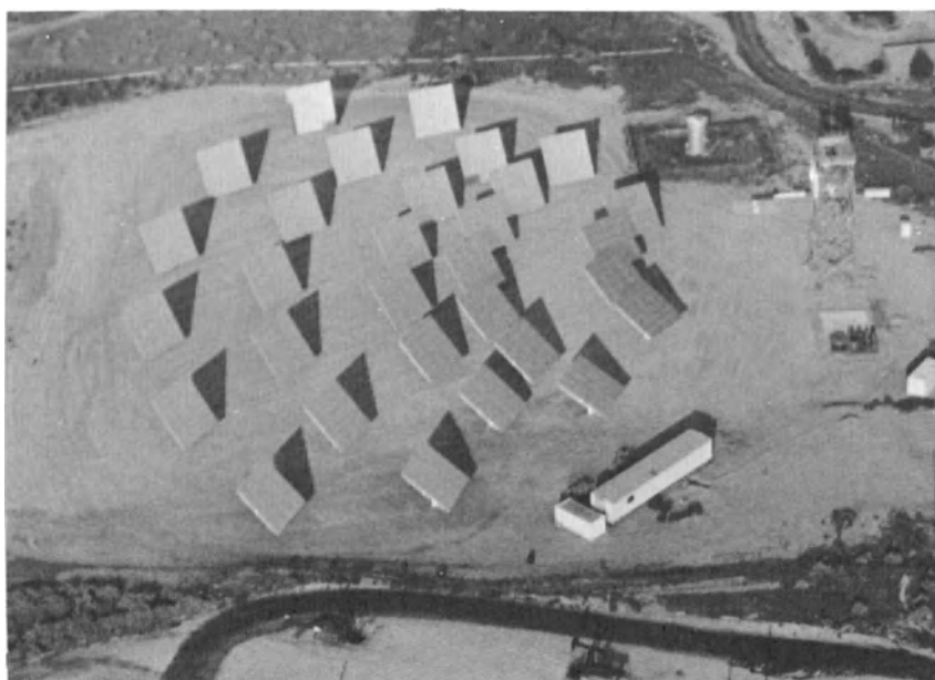
Figure 14. Aerial View of Fairfield Lease Project, July 1982
