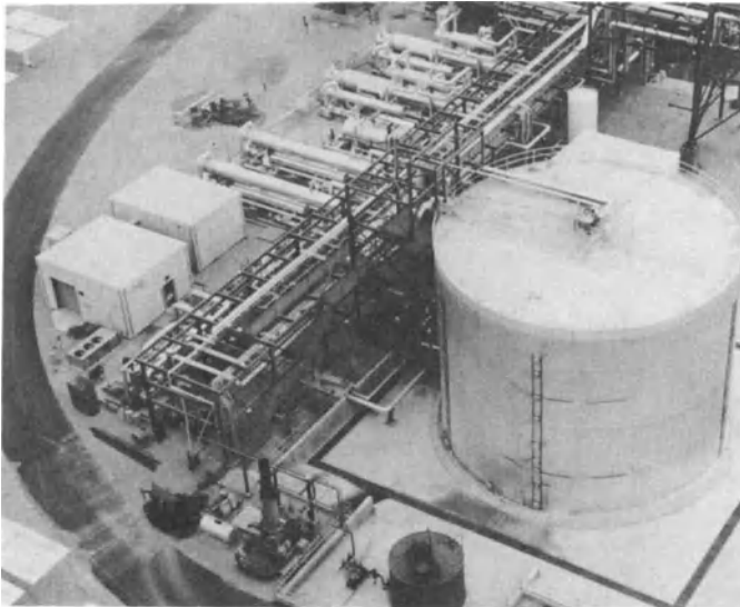
Figure 4. Solar One Storage System
