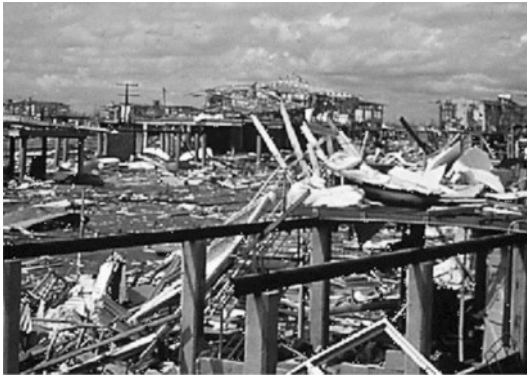
Fig. 1.3: Total suburban destruction during Cyclone Tracy, Darwin, Australia, 1974.
