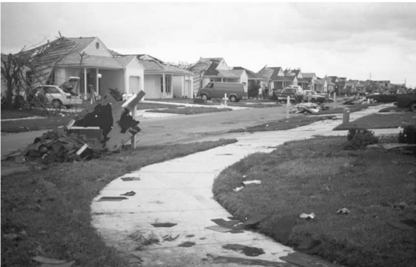
Fig. 1.2: Repeated, gable-roof-end failures on neighboring homes during Hurricane Andrew, Homestead, Florida, 1992.
