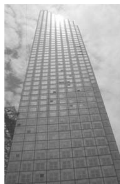
Fig. 1.8: Cladding damage in Miami, Florida after Hurricane Andrew (1992).
