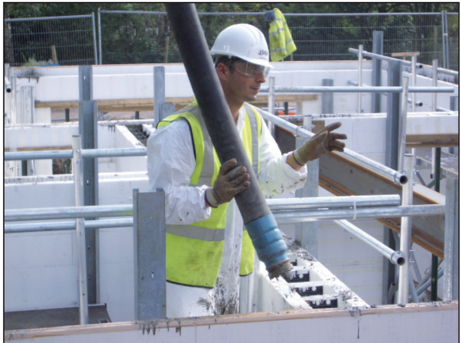
Figure 7.16 ICF filling using boom pump.
