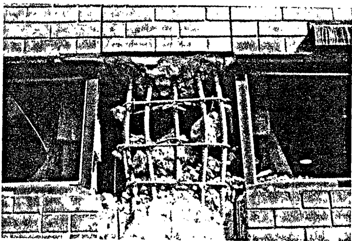
Fig. 1.3 Influence of partial height infill increasing column shear force (1985 Chilean earthquake). (Courtesy of Earthquake Spectra and the Earthquake Engineering Research Institute.)
