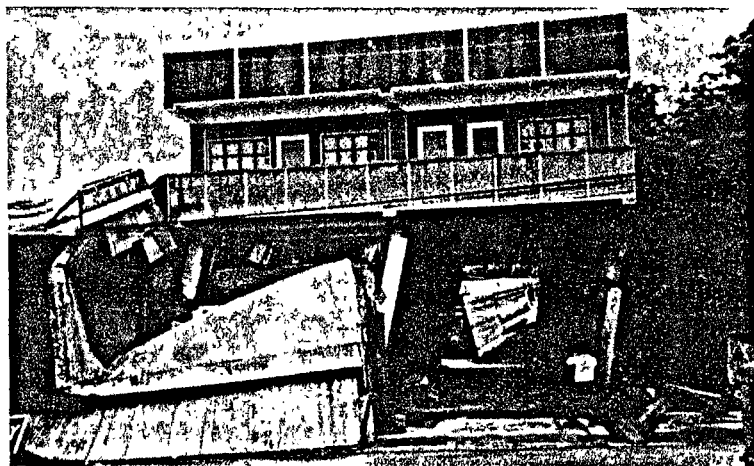
Fig. 1.1 Soft-story sway mechanism, 1990 Philippine earthquake. (Courtesy of EQE Engineering Inc.)
