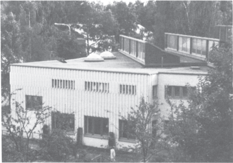
Figure 41 Alvar Aalto Museum, Jyväskylä, Finland: designed by Alvar Aalto. Note the 'reversed fluting' effect of the half-round vertical tiling on the walls.
