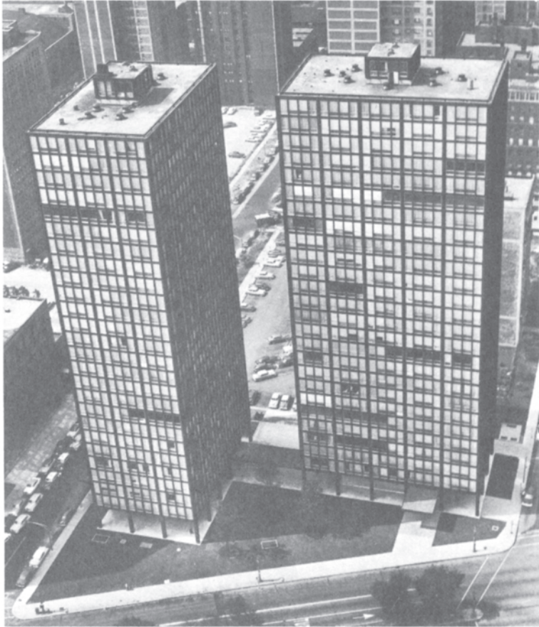
Figure 21 860–880 Lake Shore Drive, Chicago, USA: apartment blocks designed by Mies van der Rohe. Hedrick-Blessing photograph, courtesy Chicago Historical Society.
