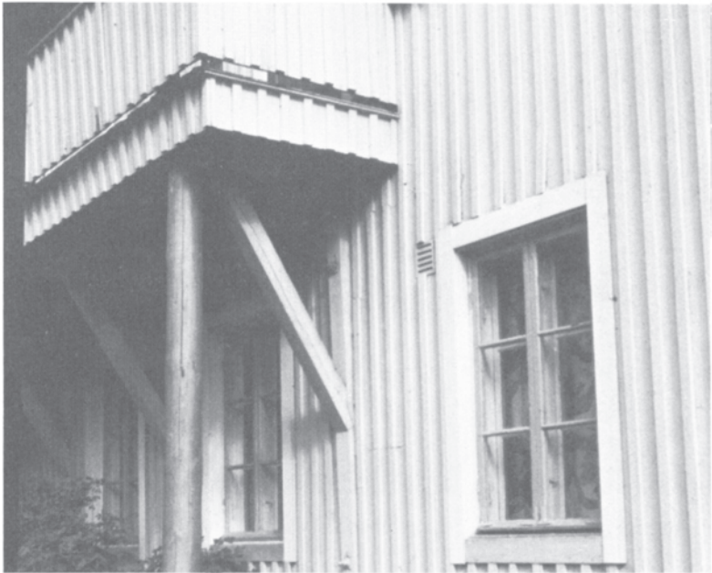
Figure 40 Detail of house (Fig. 39), showing timber battens over vertical butt-joints.
