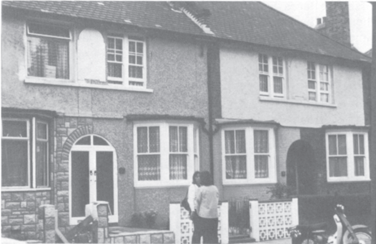
Figure 2 1930s semi-detached(?) house in North London, modified through use.
