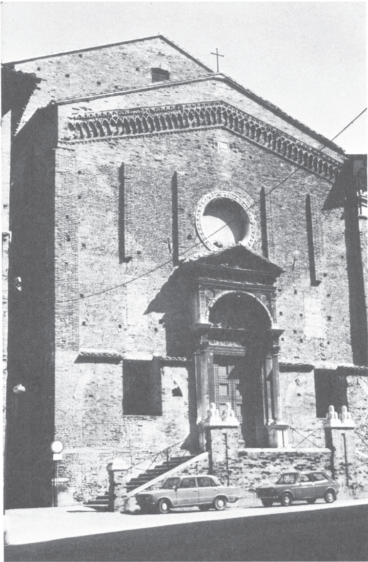
Figure 13 Church front in Urbino, Italy. Note how the construction has been adapted many times as openings and the roof line have changed. The idea that the building design must be fixed at the time of initial design has become much more forceful since the 18th century.
