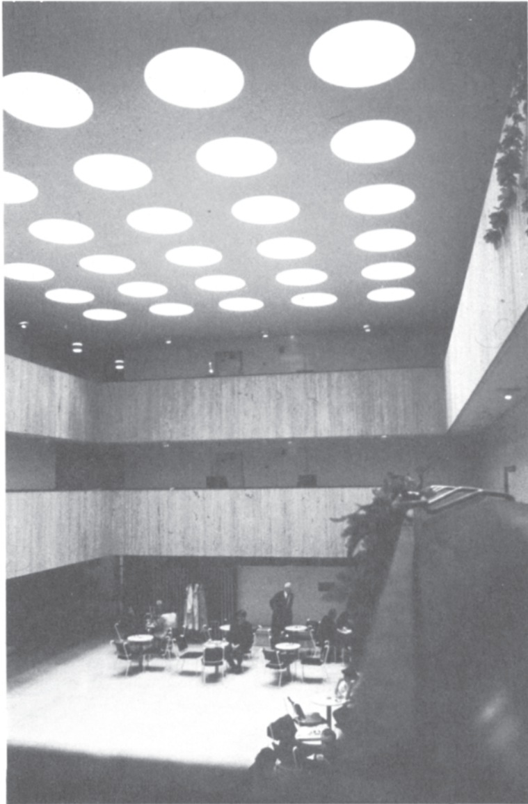
Figure 32 Rautatalo, Helsinki, Finland ('The Iron House'): office building designed by Alvar Aalto. The interior shows the public atrium space. The rooflights admit natural light; they have artificial lights outside, to replace the natural lighting pattern in Winter or at night.
