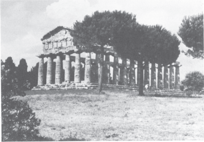
Figure 17 Greek Temple in Paestum, Italy. Note the construction of the columns: the blocks are fluted, which camouflages their assembly sequence of one block placed upon another.
