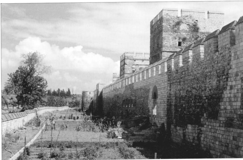
A restored section of the outer wall near the Belgrade Gate, showing the outer walkway, towers and a gateway.
