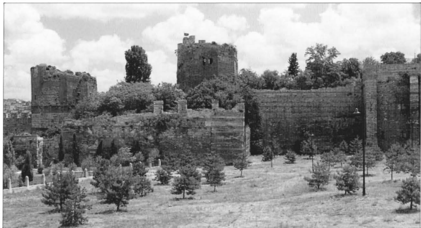
The main section of the walls of Blachernae, showing the wall of Leo and the Prison of Anemas.
