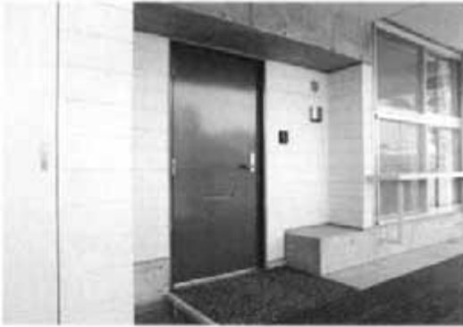
Fig. 4.119 View of the Z-beam at the entry of a dwelling unit. Photograph courtesy of HUDc Research Laboratory.
