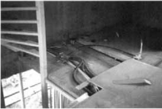
Fig. 7.4 Piping installation under the Interlevel floor. Photograph by Stephen Kendall.
