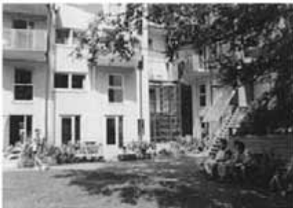
Fig. 4.94 View of the inner courtyard. Photograph courtesy of Joanne de Jager.
