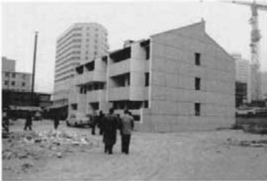
Fig. 4.88 Photograph courtesy of Zhang Qinnan.
