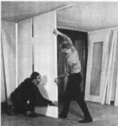
Fig. 4.4 Residents installing an interior partition. Photograph courtesy of Metron Architects.
