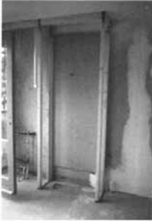
Fig. 7.7 Wall system studs being erected. Photograph by Stephen Kendall.
