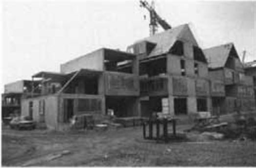
Fig. 6.3 Tunnel-formed Support structure. Photograph by Stephen Kendall.
