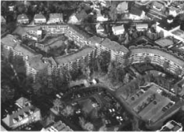
Fig. 4.113 Aerial view of the project in the neighborhood. Photomontage by Michel Hofmeester. Courtesy of AeroCamera BV.
