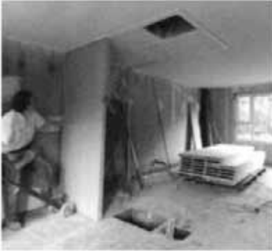
Fig. 7.9 Wall element being installed. Photograph courtesy of Nijhuis BV.
