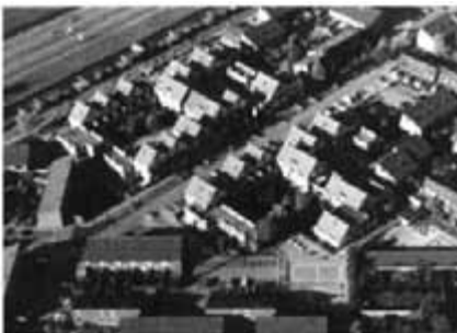
Fig. 4.27 Aerial view of the project. Photograph courtesy of Michel Hofmeester, AeroCamera BV.
