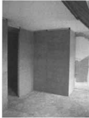
Fig. 7.8 Wall boards installed. Photograph by Stephen Kendall.
