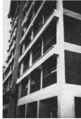
Figure 4: View of installed sunscreens
