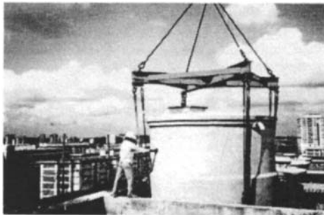
Figure 12: Erection of the completed tank
