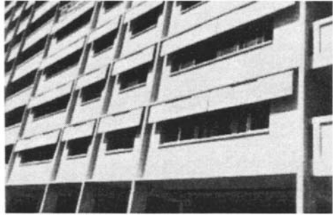
Figure 2: Sunscreens after installation
