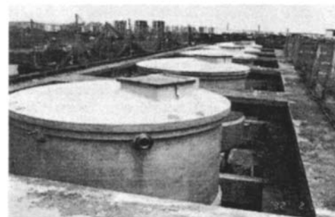
Figure 13: View of the tanks after installation
