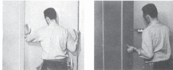
Erecting gypsum panel
