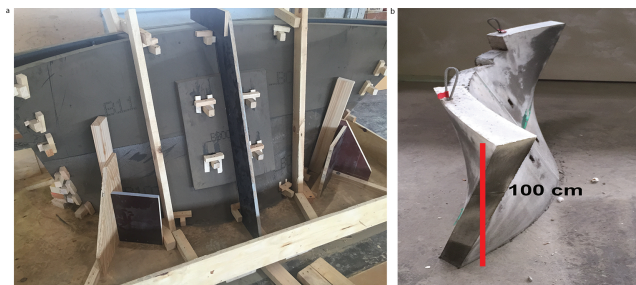
Figure 16. (a) Composite mold from 3D printed formwork elements and (b) resulting large-scale concrete member.
