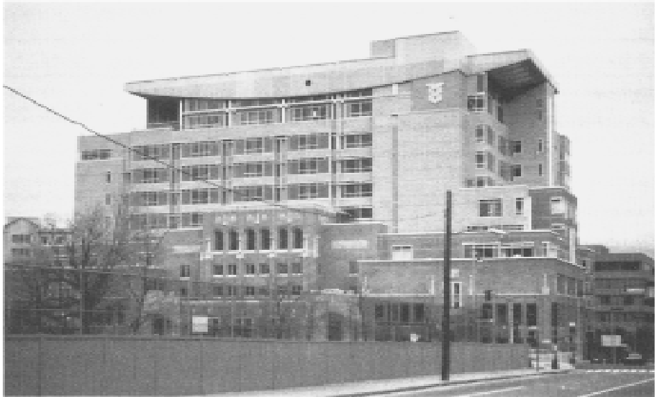
5.8 Clinical Center at Beth Israel Hospital under construction.
