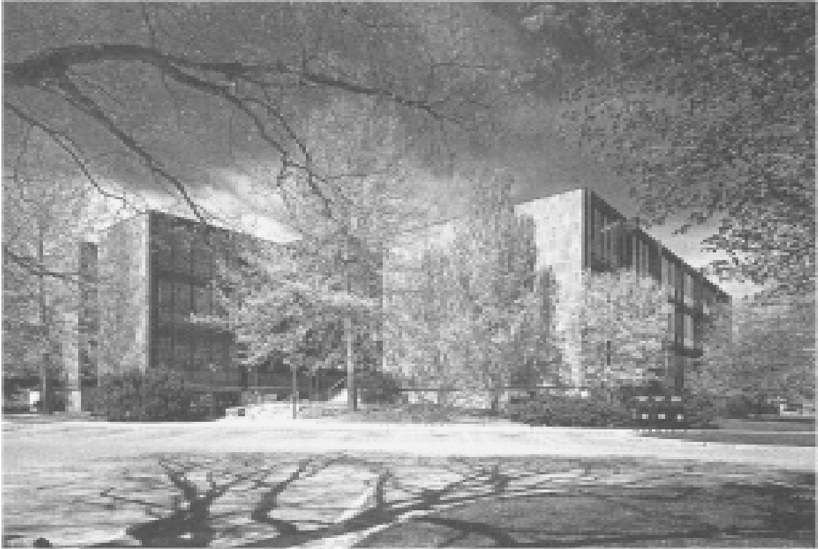
3.3 One of the Wellesley Office Park buildings. (Photo by Steve Rosenthal)
