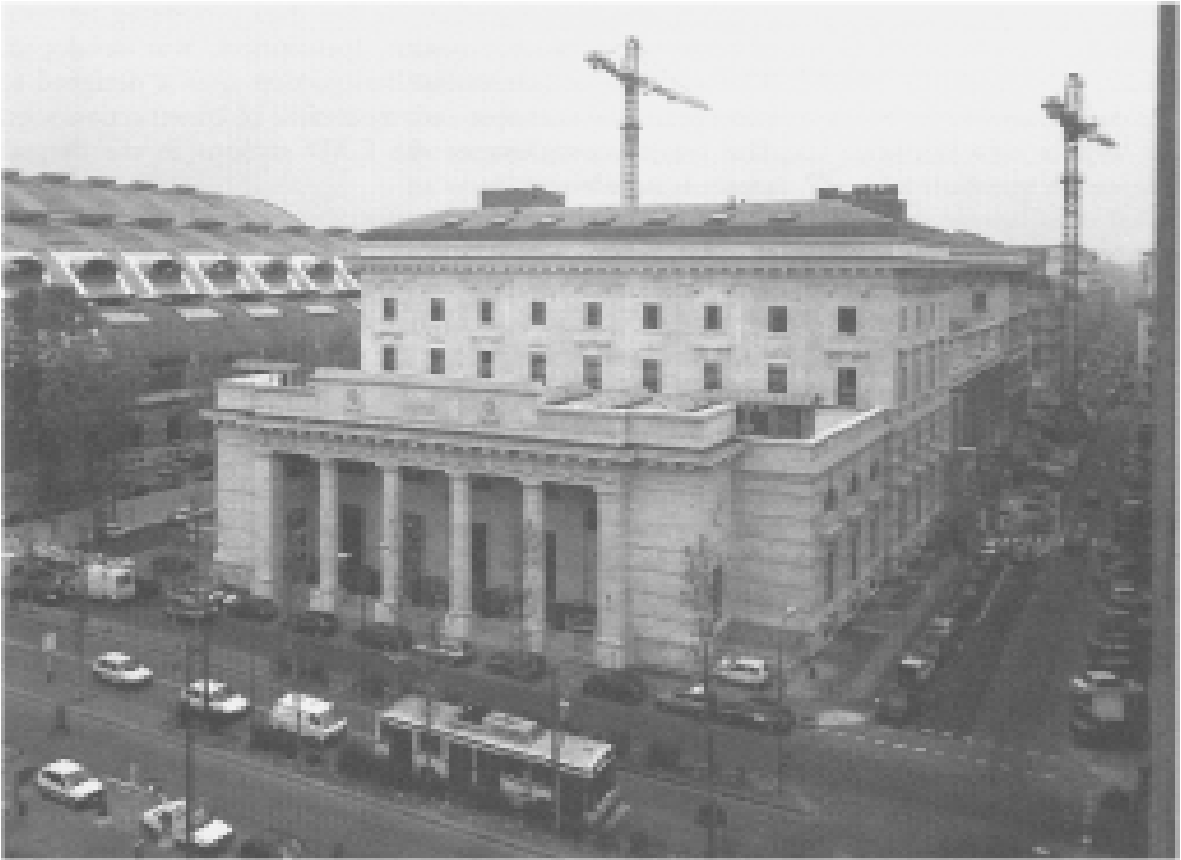
2.12 Post office headquarters under refurbishment in Milan.
