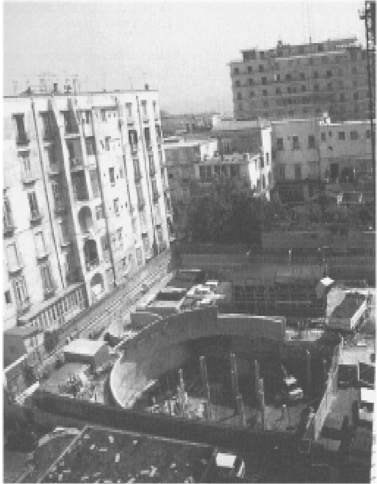
5.6 Site conditions of the SIP underground garage in Naples.
