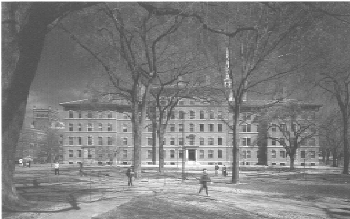
5.9 Refurbished Thayer Hall at Harvard University. (Photo by Steve Rosenthal)
