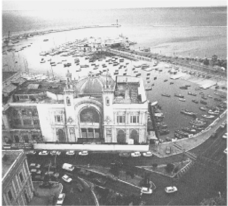
5.4 Aerial view of the Margherita Theater.
