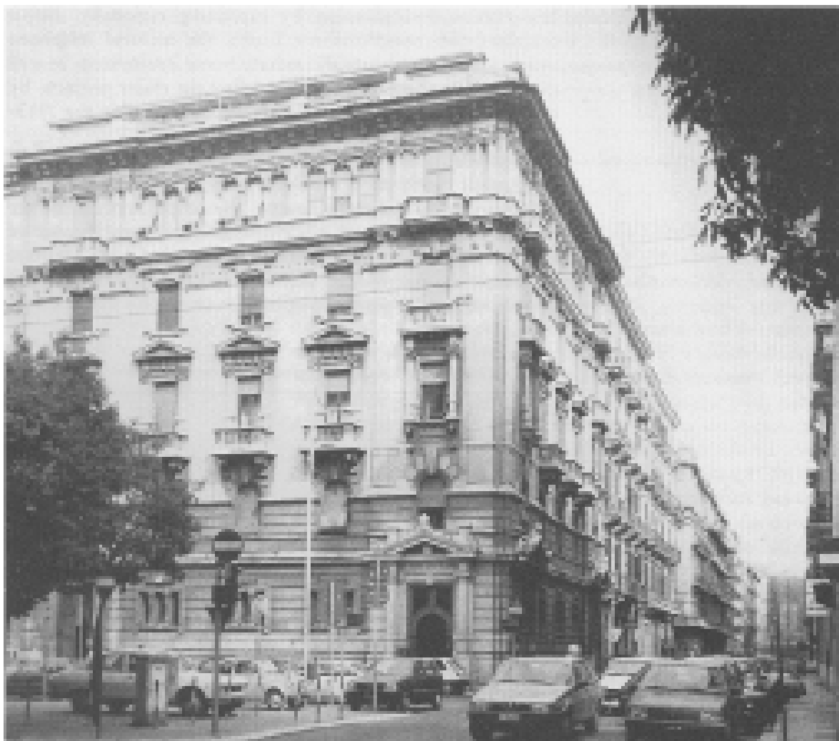
2.1 Residential building in Bari.
