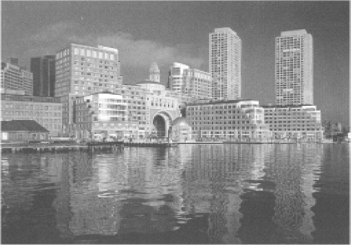
3.7 Rowes Wharf complex. (Photo by Steve Rosenthal)
