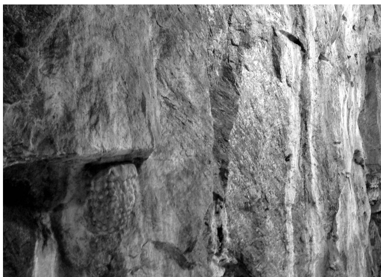
Figure 12.4 A blasted rock wall has a quite ideal diffusion and little sound absorption. (Photo by Mendel Kleiner.)
