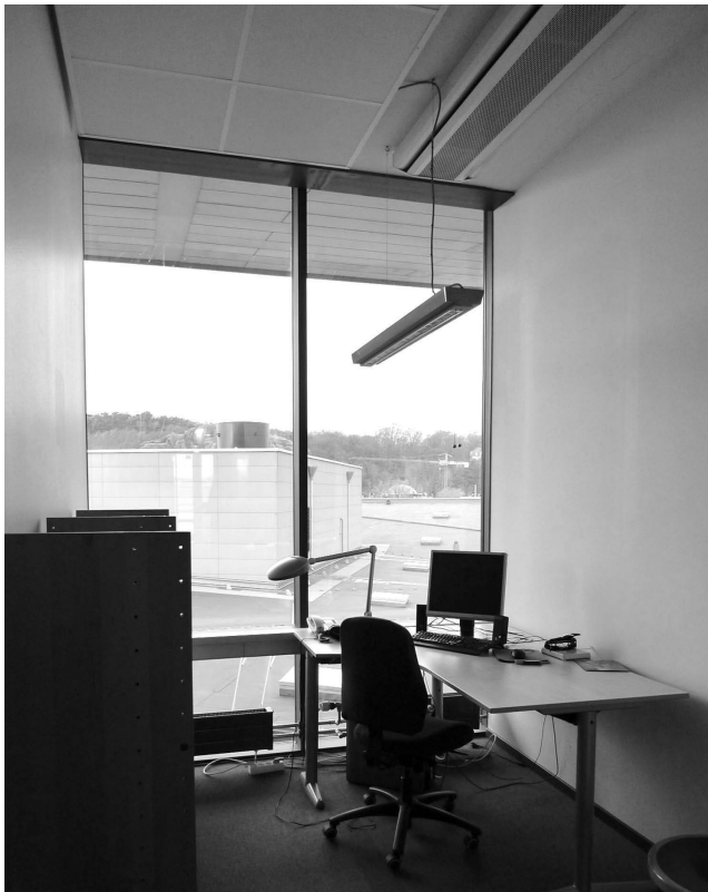
Figure 12.14 This photo shows a room that has a sound absorptive ceiling and carpet along with mirroring plane and parallel side walls, all of which contributes to reflection patterns that result in colored sound and flutter echo. (Photo by Mendel Kleiner.)
