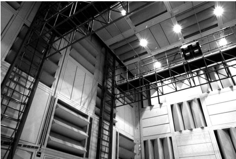
Figure 12.8 Detail of IRCAM's Espace de Projection showing the rotatable wall elements. (Photo by Leif Rydén.)
