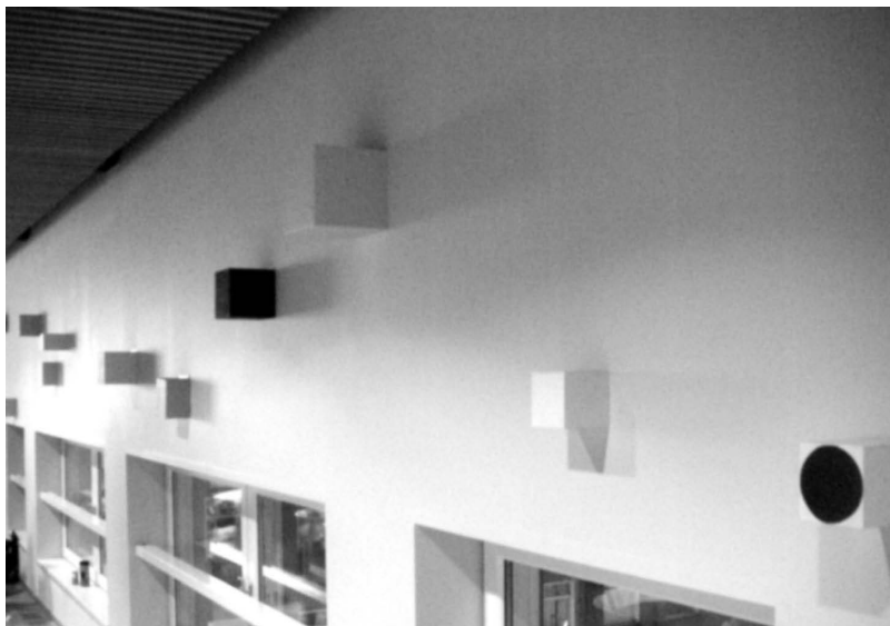
Figure 3.11 Is this to be considered plane wall with mirroring boxes or a diffusing wall with sparse diffusers? (Photo by Mendel Kleiner.)
