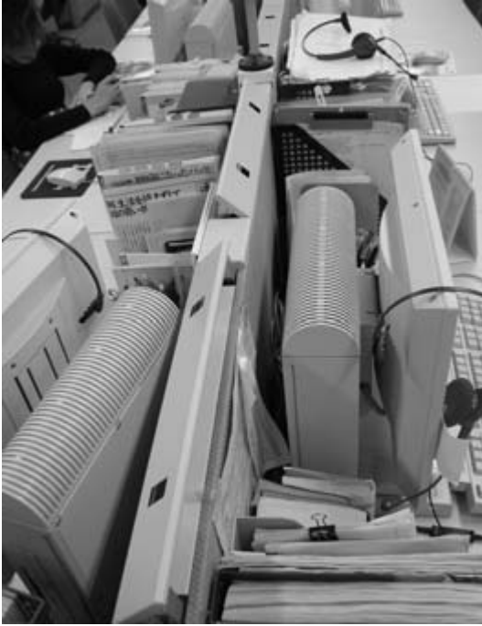
Fig. 5.8 Adjustable ventilation supply in partitions
