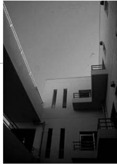
Fig. 19.14d 'Void' for day-lighting and natural ventilation
