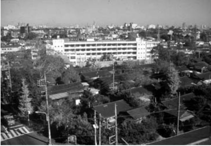
Fig. 19.9 The designated site of the Fukasawa Complex with original wooden public housing (April 1994)
