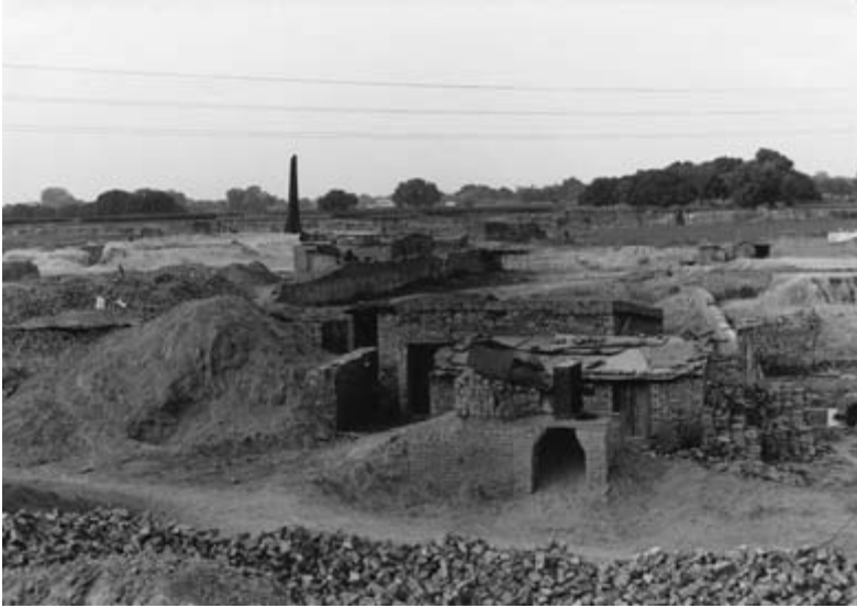
Fig. 15.5 Bull's Trench kilns: The British brought the Bill's Trench kiln system to India. An oval trench, which spans the illustration, permits a continuous building and firing of a kiln. The black iron chimneys are manhandled so as to be above the kiln at all times (Photo: © Paul Oliver)
