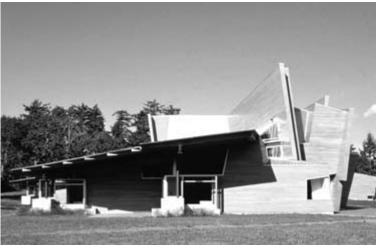
Fig. 5.3 Elimination of traditional finish materials (Strawberry Vale School, Saanich, BC. Patkau Architects, 1996)
