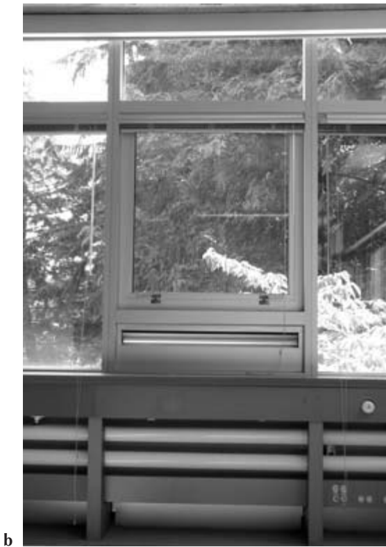
Fig. 5.9 a. Openable window in CK Choi Building. b. Openable window in Lui Centre. c. Detail of window opening in Lui Centre
