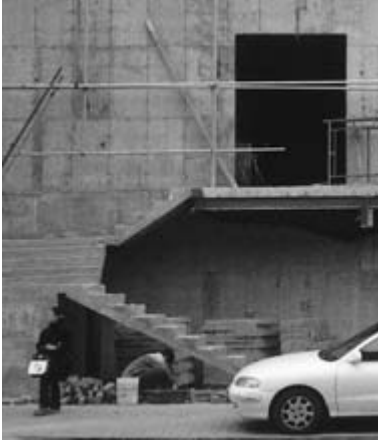
Fig. 3.2 Ulsan Stadium: manual placement of concrete and rubble infill
