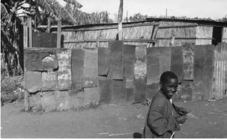
Fig. 15.4 Tin plate: bidons or flattened oil drums and other waste metal sheeting have been used to wall in this compound in Mozambique. Traditional panels of layered palm leaf are used for the walls, but the roof is of galvanised iron sheeting (Photo: © d'Alpoim Guedes)
