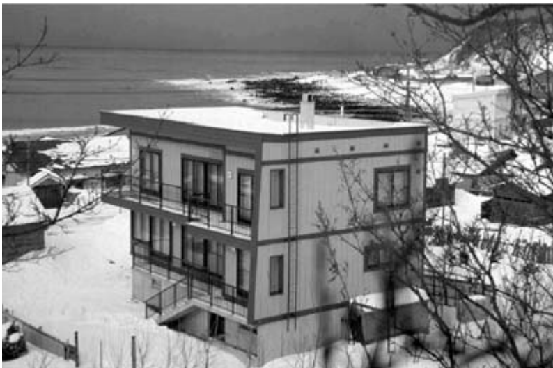
Fig. 18.4 KST house – general view
