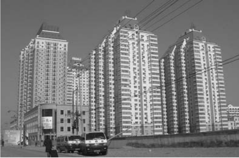
Fig. 17.6 Housing in a northern suburb of Beijing with a density (plot ratio) of about 3.0
