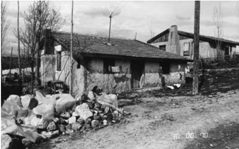
Fig. 15.7 Disaster housing: following the Gediz, Turkey, earthquake, post-disaster housing on a European model was provided. Extensions were built by the occupiers to provide space for their families and to conceal the access to the toilets. These were not earthquake-proof but they were culturally more appropriate (Photo: © ODA Gediz Project)
