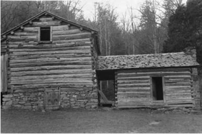
Fig. 15.3 Logging on: Lige Oliver (no relation) built his cabin at Cades Cove, Tennessee, in the nineteenth century. The main building is 'square-notched', but for the kitchen 'half-dovetail' notching was used. Both have been learned from other settlers, for no notching system was ever used in Britain (Photo: © Paul Oliver)
