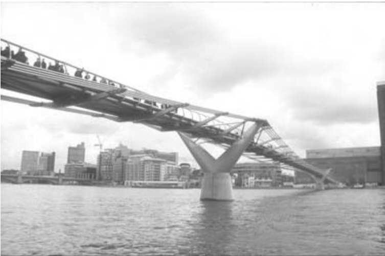
Fig. 4.2 Millennium Bridge, London (Photo: Arup / Thomas Graham)
