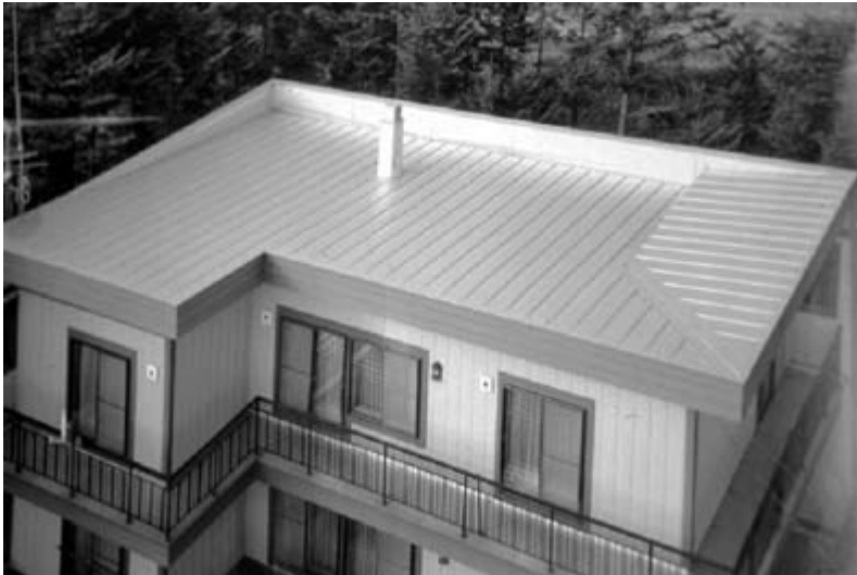
Fig. 18.5 KST house showing inverted roof
