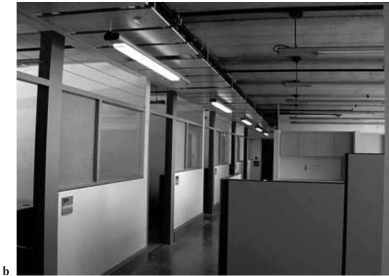
Fig. 5.5 Elimination of finish materials. a. C.K. Choi Centre for Asian Research b. Lui Centre for the Study of Global Issues
