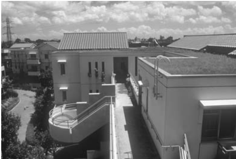
Fig. 19.16 North side of Apartment IV, characterised by grass rooftop and the 'Sky Walk'. Rooftop greening was one of the most outstanding characters of this project. Major objectives were to contribute to regional green networking and to improve the urban thermal condition
