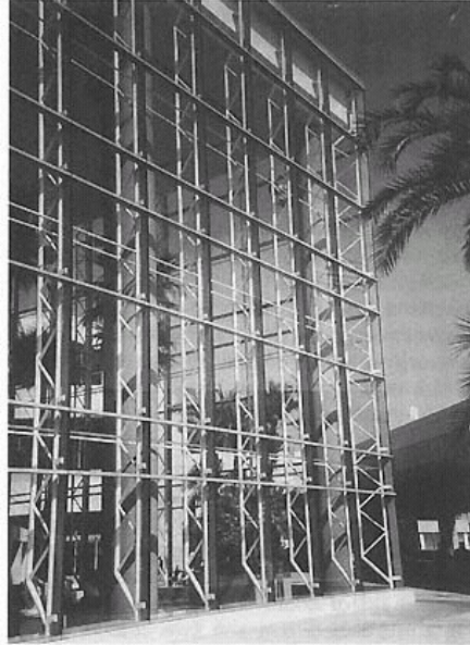
Figure 8-9 Glass cladding wall attached inside aluminum frames. Photograph by author.
