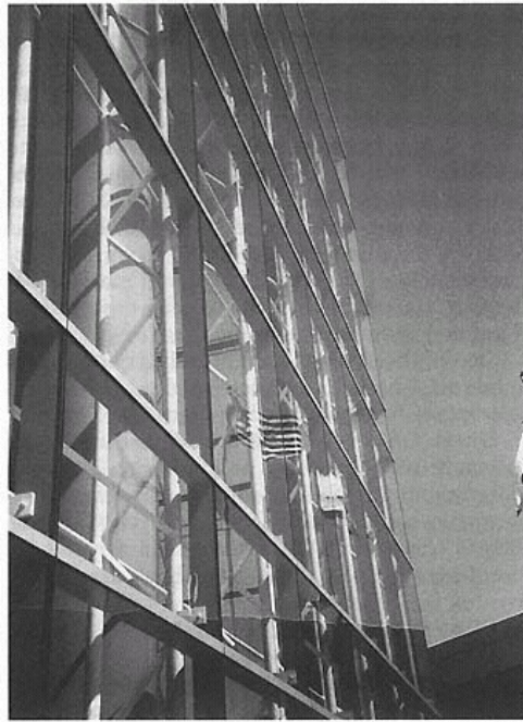
Figure 2-7 Some modern buildings use glass panels set in metal frames for the cladding system. Photo by author.
