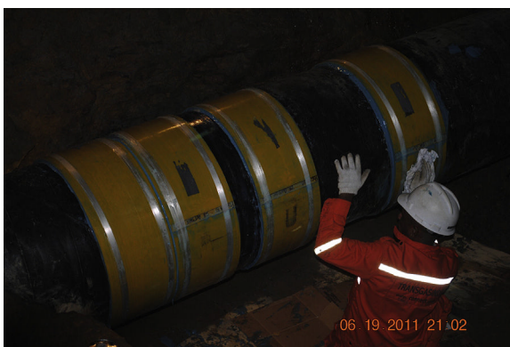
Figure 6.10 Completed 28-in. repair sleeve installation.
