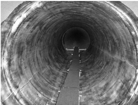
Figure 1.4 Completed CFRP liner.
