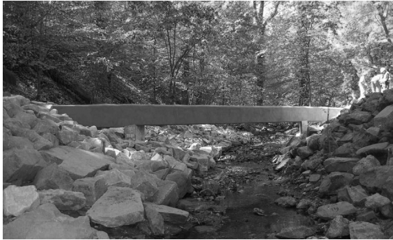
Figure 1.9 Aerial sewer crossing (Bian et al., 2011).
