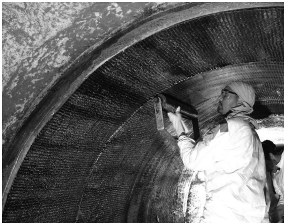
Figure 2.6 Installation of the circumferential layer of CFRP (Gipsov et al., 2012).
