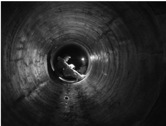
Figure 2.2 Completed CFRP-lined section. Courtesy of Mr Hector Posada of Tucson Water.
