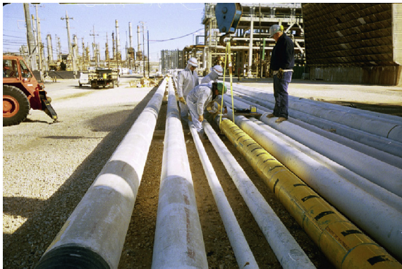
Figure 6.21 Installation of Clock Spring ® at a refinery.
