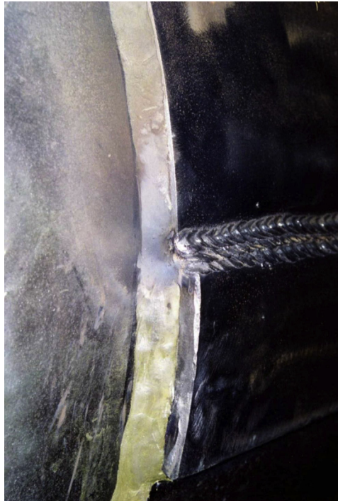
Figure 4.10 Type A sleeve end with hardenable sealant.
