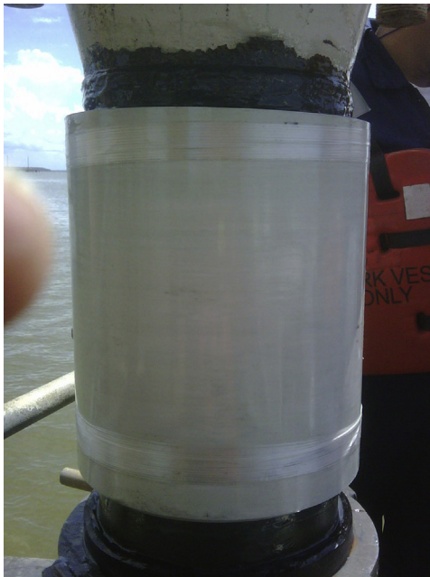
Figure 6.12 Completed high-temperature composite sleeve repair.
