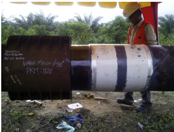
Figure 6.19 Completed high-temperature repair.
