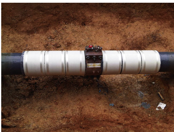
Figure 6.20 Completed crack arrestor repair.
