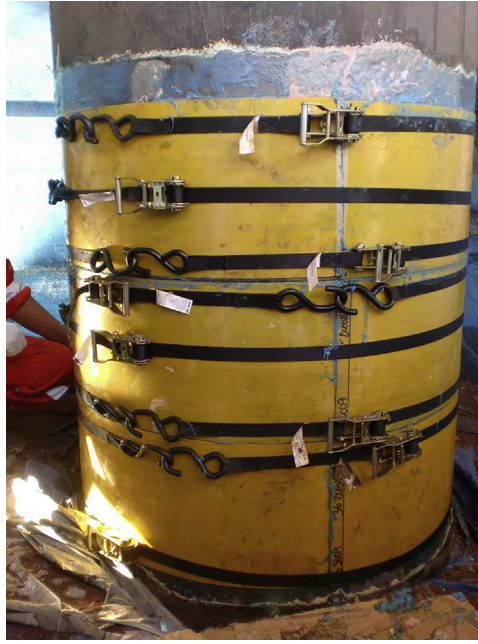
Figure 6.14 Sample of completed sump caisson repair.
