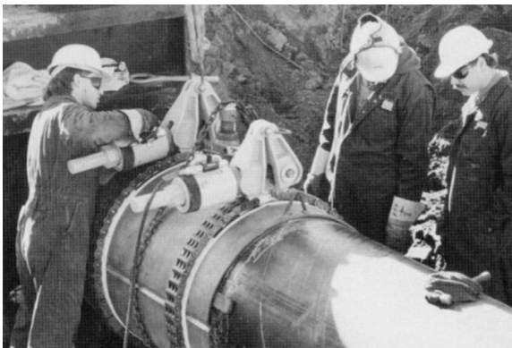
Figure 4.9 Hydraulic clamps being used to preload a steel sleeve during installation.
