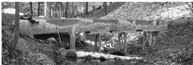
Figure 1.8 Original condition of aerial sewer crossing (Bian et al., 2011).
