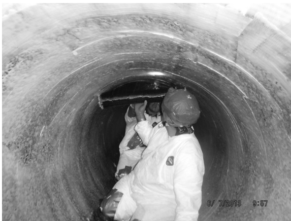
Figure 1.7 Internal application of CFRP.
