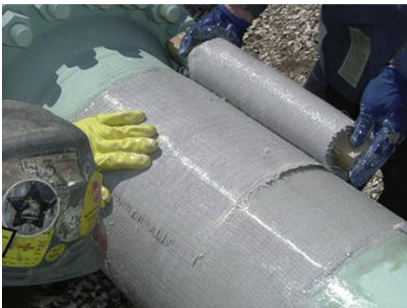
Figure 4.5 Installation of wet lay-up composite wrap (Armor Plate ® pipe wrap).
