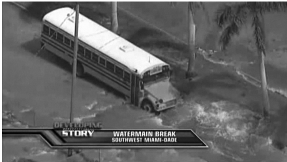
Figure 1.1 Large-diameter water main break.
