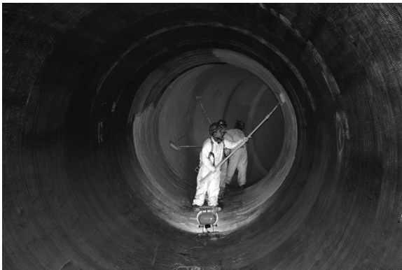
Figure 3.4 Application of top coat to a large-diameter pipe.
