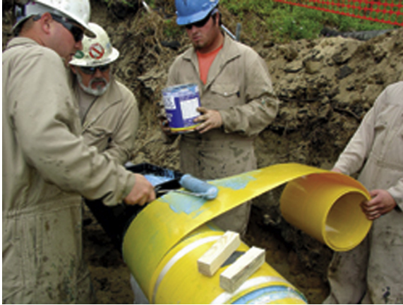
Figure 4.4 Installation of preformed composite sleeve (Clock Spring ® ).
