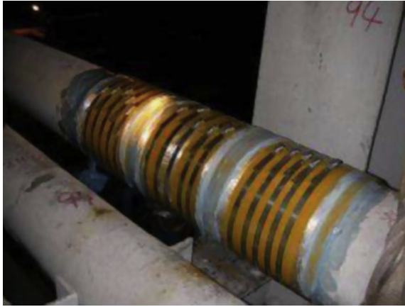
Figure 6.23 Completed installation of Clock Spring®.
