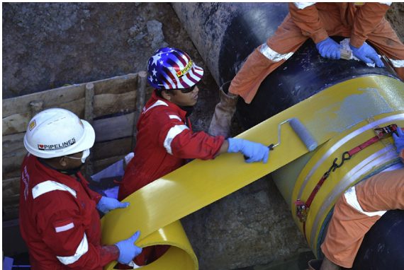
Figure 6.8 Installation of the 32-in. seam sleeve.
