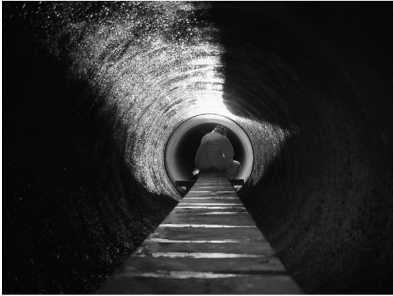
Figure 1.3 Prepared surface on inside of pipeline.
