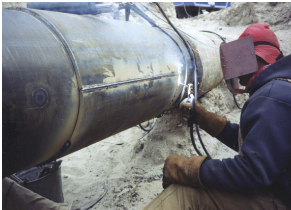
Figure 4.11 Installation of Type B full-encirclement repair sleeve.
