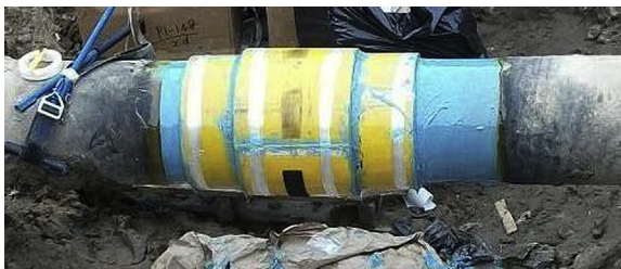
Figure 6.15 Completed girth weld repair.
