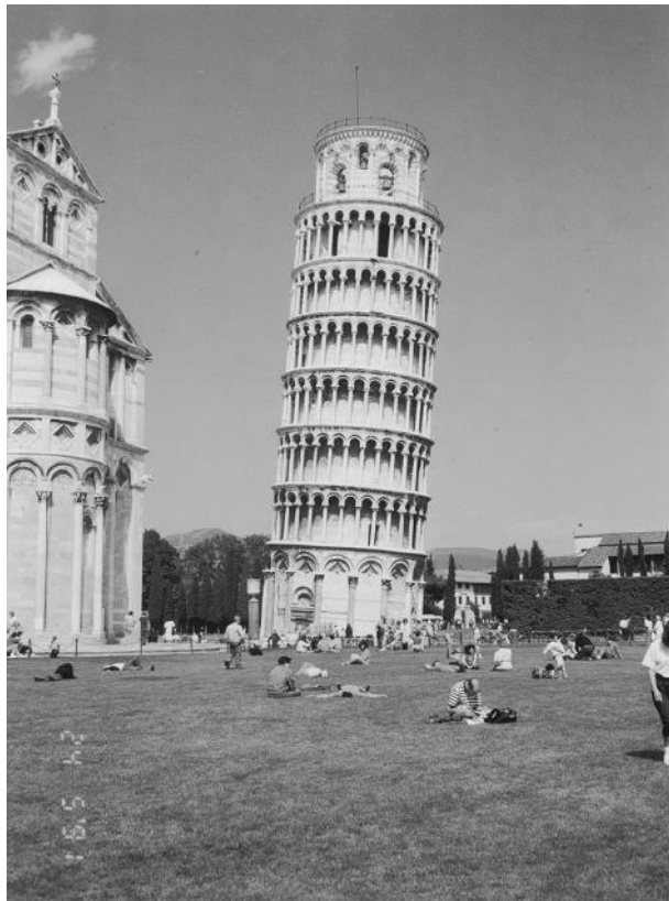
Figure 1.2 A well-known building with an inadequate foundation (Pisa, Italy). (Photograph courtesy of Professor John Burland.)
