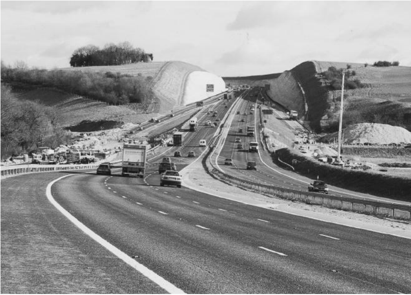
Figure 1.1 A visible and, at the time of its construction controversial, road cutting (the M3 motorway at Twyford Down, near Winchester, Hampshire, England). (Photograph courtesy of Mott MacDonald.)
