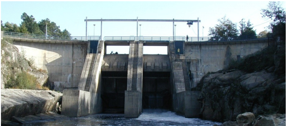
Figure 1. Fagilde dam. Downstream view
