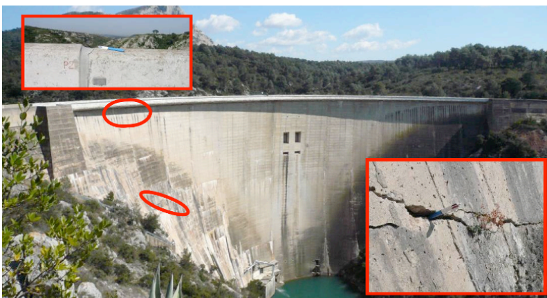
Figure 1. Bimont Arch Dam
