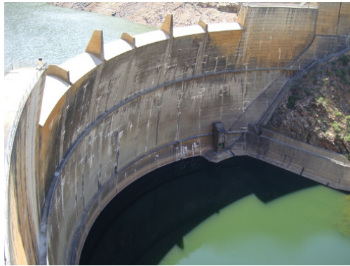
Figure 7. Downstream view of Kouga Dam (previously named Paul Sauer Dam)
