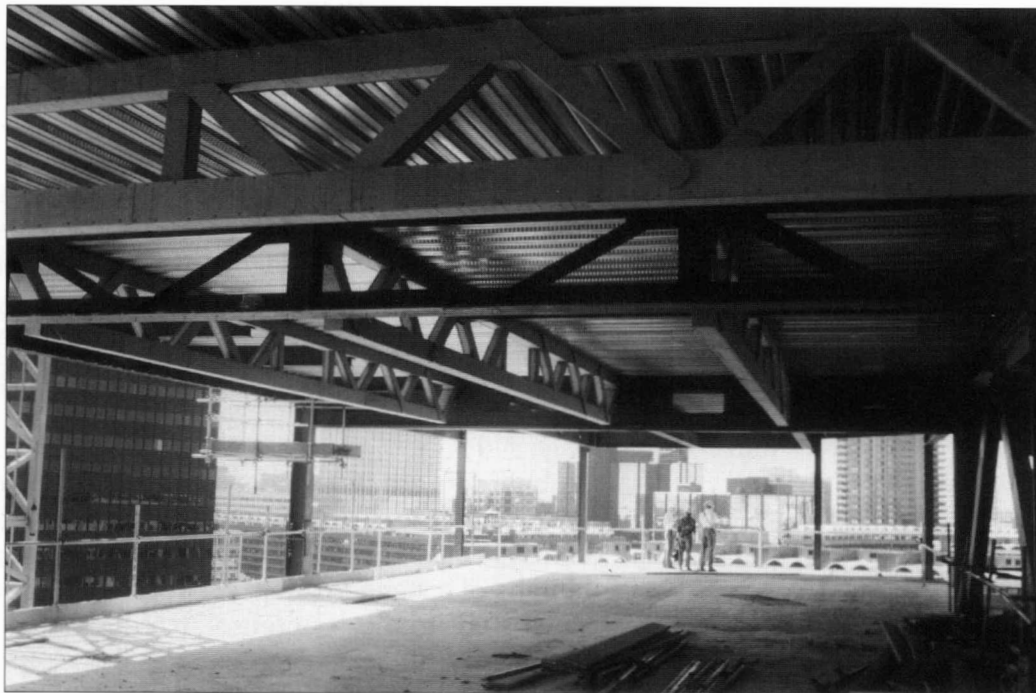
Figure 24 Composite truss showing fire protection
