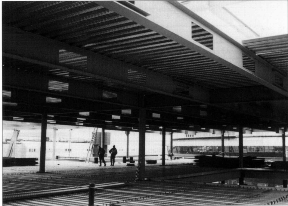
Figure 19 Openings in the webs of composite beams
