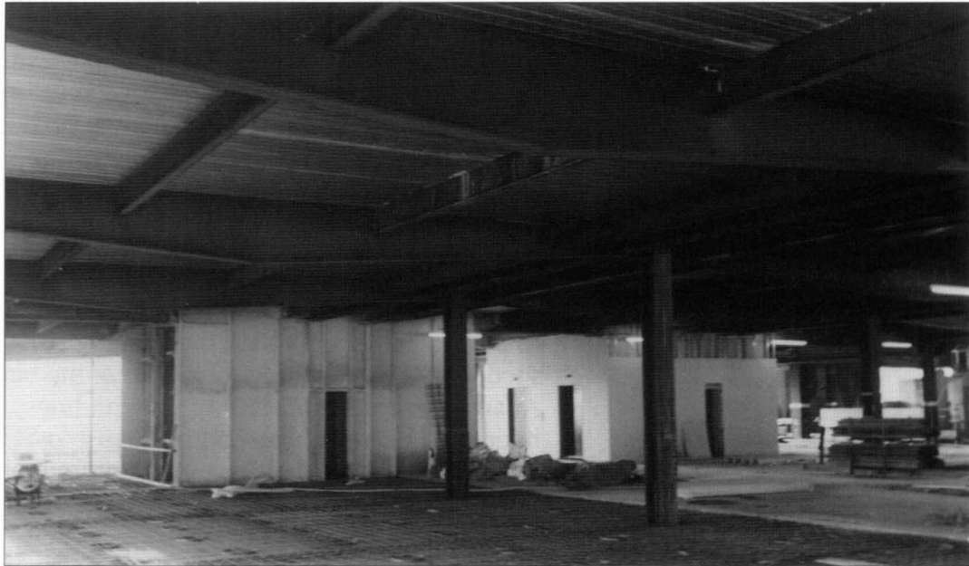
Figure 23 Tapered fabricated beam
