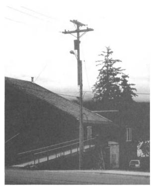
Figure H261A2d-3 Inappropriate side-by-side top pole splice
