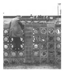
Figure H110A1-6 Supply station enclosure not meeting requirements of either Rule 110A1 requirements for limitation of climbability or Rule 124 for clearance to energized parts
