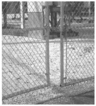
Figure H110A1-7 Supply station fence gate with too large a gap between panels
