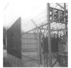
Figure H110A2-4 Solid section prevents contact with close facilities-other areas of fence meet clearances of Rule 110A2
