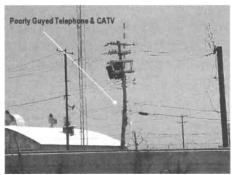
Figure H260-2 Pole overloaded by unguyed communication opposite heavy equipment
