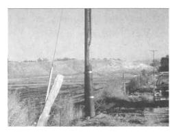
Figure H261A2d-2 Stub pole too short
