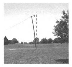
Figure H260-3 Pole deformed by unbalanced service drop tension
