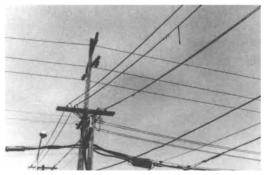
Figure H230-3 Covered conductor with deteriorated covering
