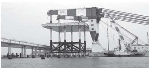
Photo 2. A scene of installation of a jacket unit.
