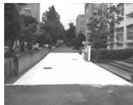
Photograph 5. Water-retentive pavement (F).
