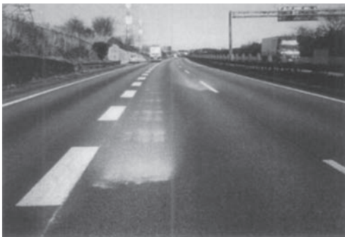
Photo 1. Blow-up of binder mix's particles through surface porosity.
