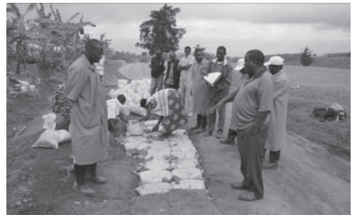
Figure 2. Demonstration of spot improvement using "Do-nou" with the staff of LBT training institute and contractor.
