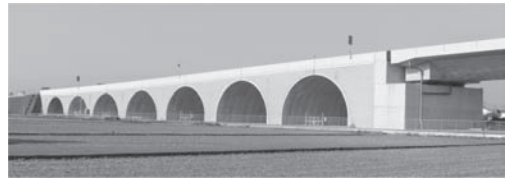
Figure 1. Multi-arch culverts embankment.
