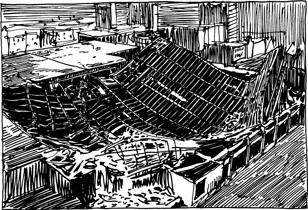
4.10 Hartford Center Roof: after the Collapse
