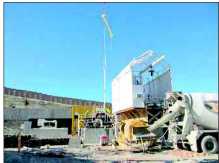
Figure 14. Grouting well casing
