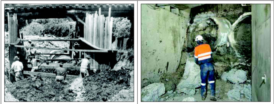
Figure 10. Concrete culverts installed in 1953 and demolition of pipes during jacking operation
