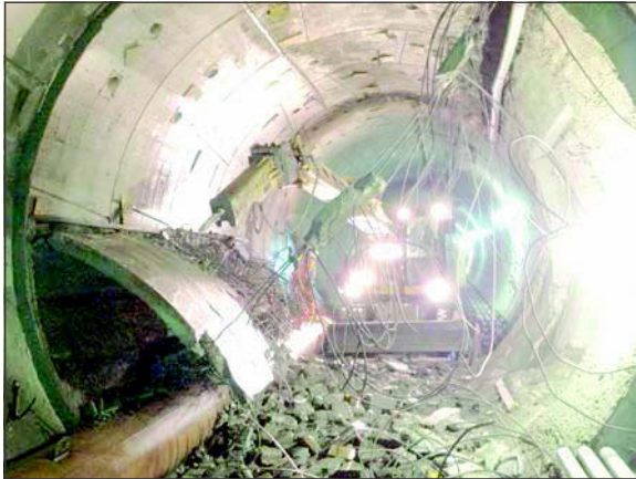
Figure 8. Conveyor side shell removal
