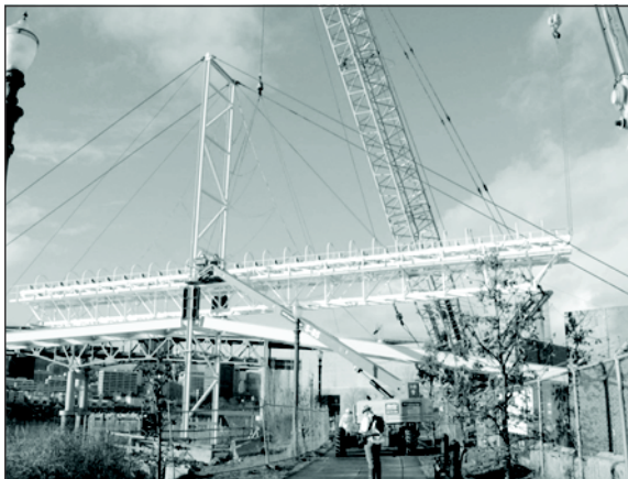
Figure 4. Installation of conveyor for tunnel muck loadout
