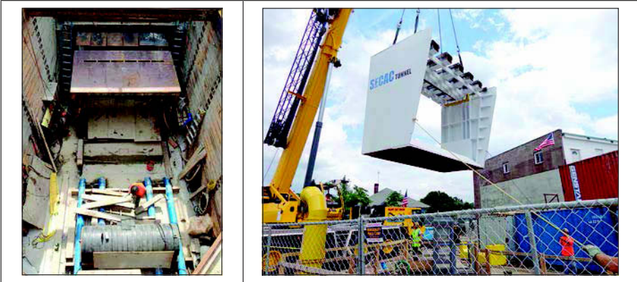
Figure 11. Cutting shield and trailing/steering shield
