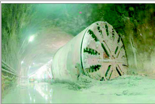
(A) Partial invert excavation
