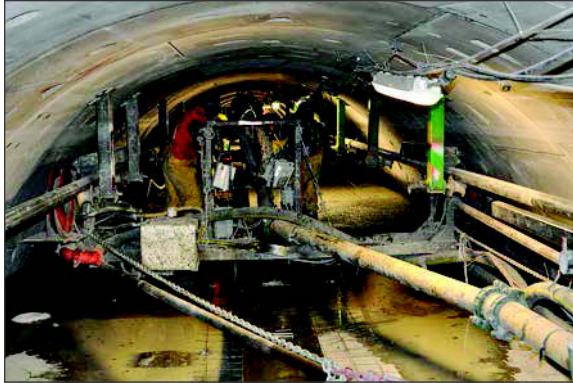
Figure 5. Steel drain forms and concrete distributor
