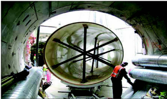
Figure 7. Pipe section at BT3 tunnel eye
