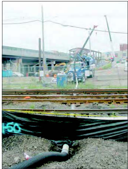
Figure 21. Cross dig with screw sucker and vacuum truck on the other end
