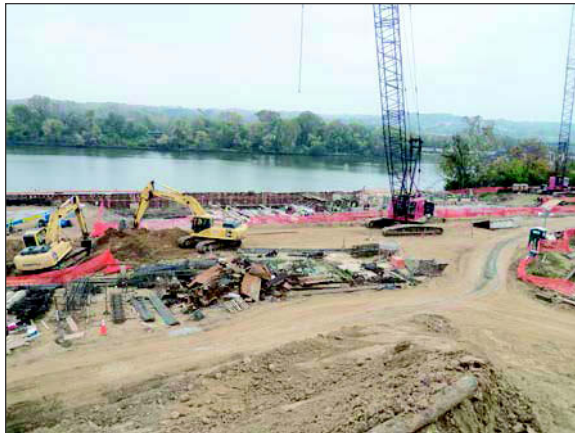
Figure 3. Overflow structure at CSO #19
