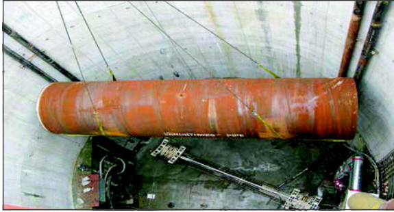
Figure 6. BT3 pipe lowered onto hydraulic turn table
