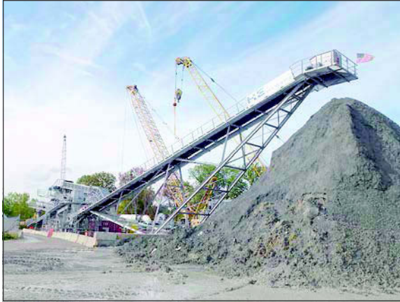
Figure 2. ECT on surface conveyor system
