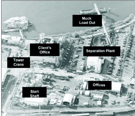
Figure 3. Main construction site—Opera shaft
