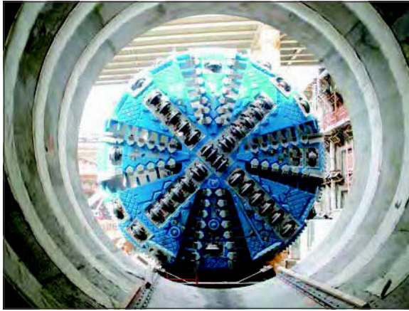
Figure 10. Bullflex bags in the launch block for the A Tunnel
