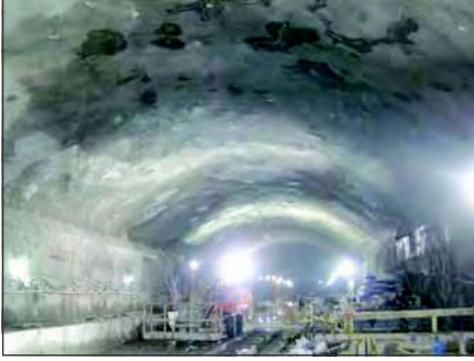
Figure 8. Separated arch header excavation
