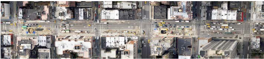
Figure 14. Aerial view along 2nd Avenue as the shaft sinking work started in late 2010 at 69th and 72nd Streets. Four lanes of traffic had to be maintained except for specific periods of the day—Monday to Friday.
