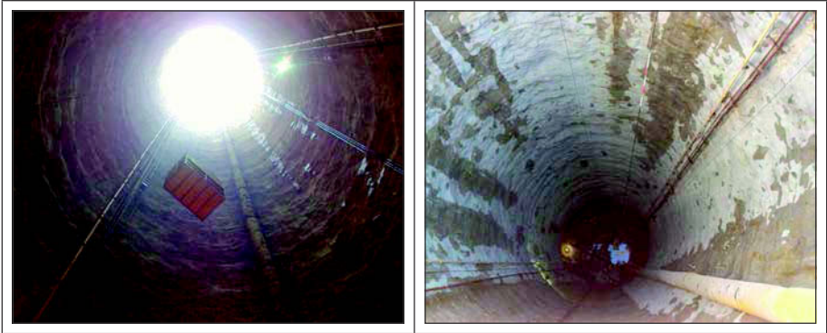
Figure 9. The excavated shaft with minimal ground water infiltration
