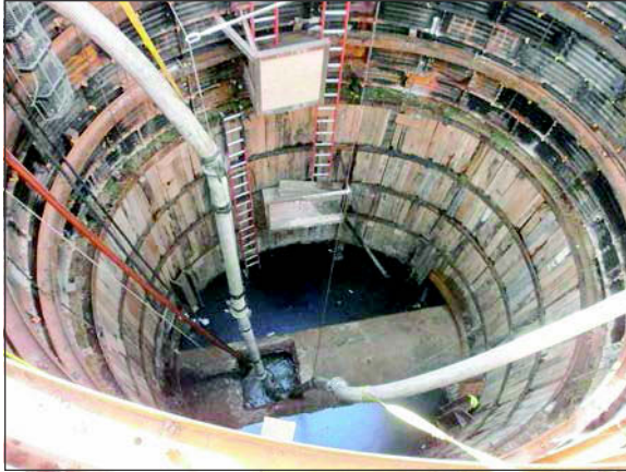
Figure 5. Typical access shaft on M Street during ESI rehabilitation work
