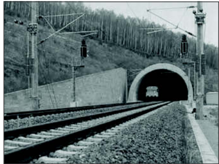
Figure 4. Sinnberg Portal at oblique angle (Courtesy of ILF Consulting, USA)
