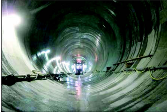
Figure 6. Finished concrete liner
