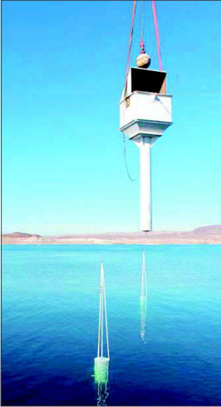
Figure 4. Sealed bucket used to place concrete underwater
