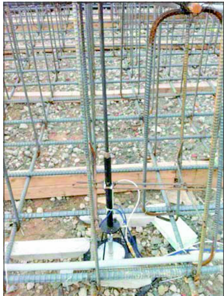
Figure 8. Total stress cells mounted on rebar for diaphragm wall panel
