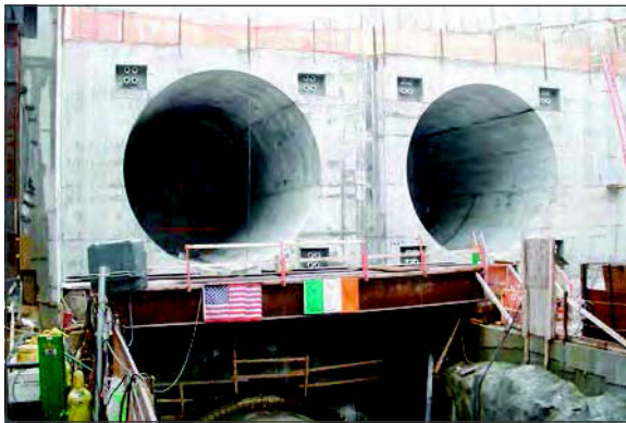
Figure 3. Launch blocks—during construction
