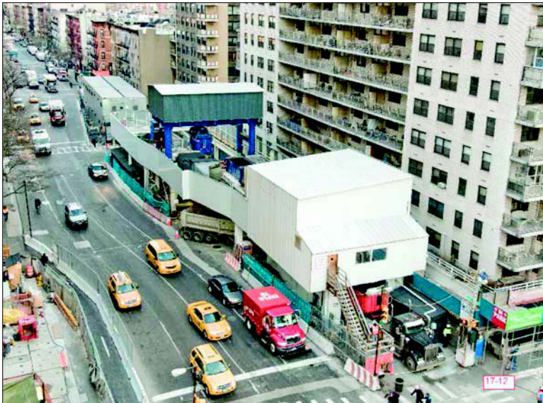
Figure 4. Photograph of completed north shaft muck conveyance system
