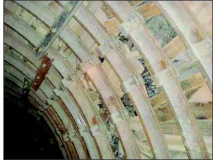
Figure 6. TH profiles installed in coal mine
