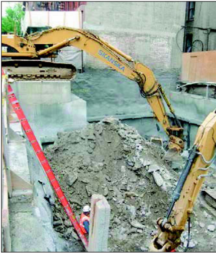
Figure 9. Mucking with 345
