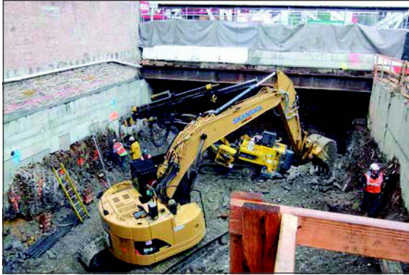
Figure 5. Excavating down to Elevation 130
