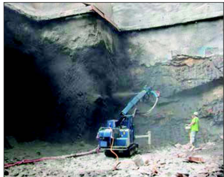
Figure 11. Shotcreting with Oruga
