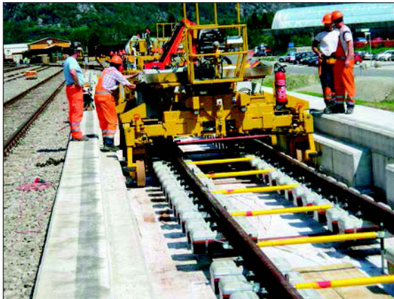
Figure 7. Special machines for attaching LVT sleepers to the rails (Source: ABH, 2010)
