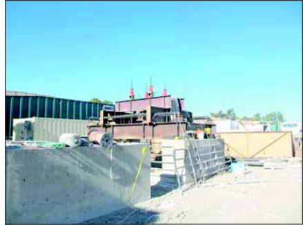
Figure 12. Well casing support frame
