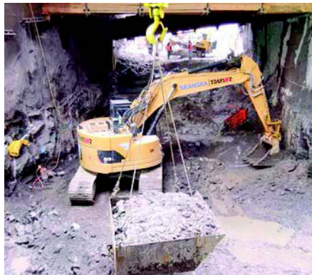
Figure 8. Mucking with 321 and 45t crane
