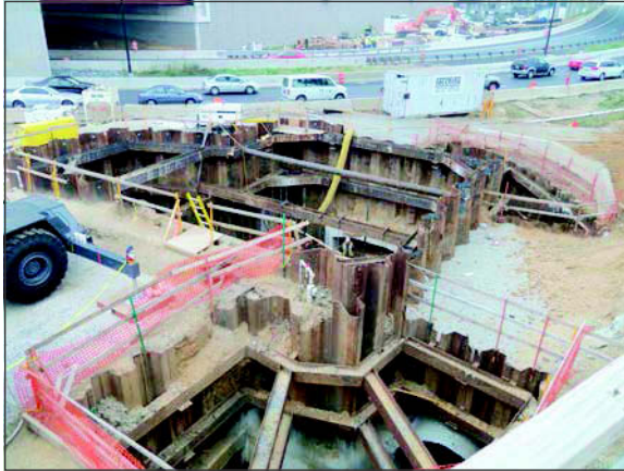
Figure 6. Diversion structure at CSO #7, Division G
