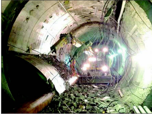
Figure 13. Conveyor side shell demolition
