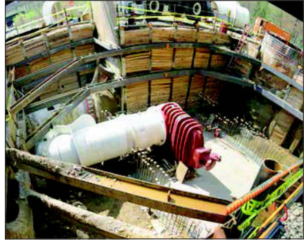
Figure 7. 1,829 mm diameter (72 in.) pipe tie-in and valve installation at S-4
