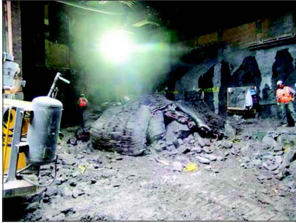
Figure 6. Matting during blast
