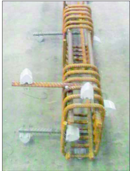
Figure 6. Radial joint reinforcing steel
