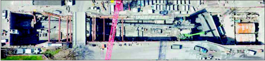
Figure 6. CHS site during the SB tunnel drive
