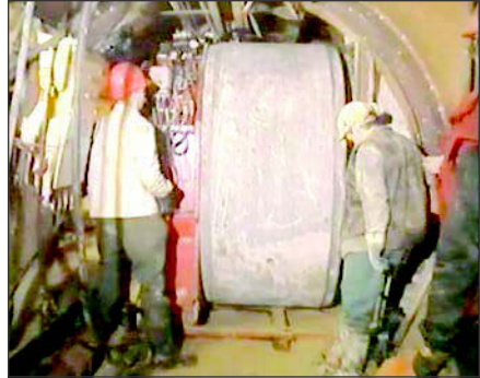
Figure 7. Driving transverse tubes
