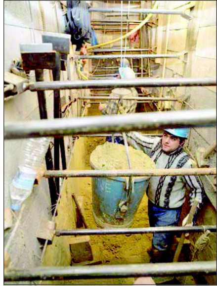
Figure 5. Manual diaphragm wall excavation
