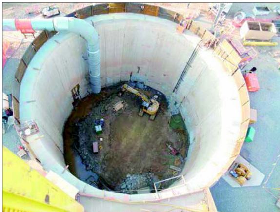
Figure 16. Blue Plains shaft BPT-SS 76' diameter—slurry walls exposed
