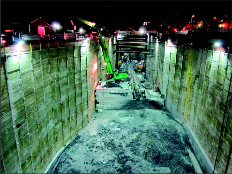
Figure 4. Muck pit and truck loading on the NB Drive
