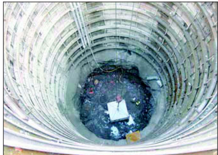
Figure 3. Excavation of main working shaft
