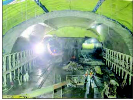
Figure 9. Cast segment of the separated arch final lining
