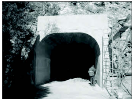
Figure 6. Brow repaired with mass concrete (Mexico)
