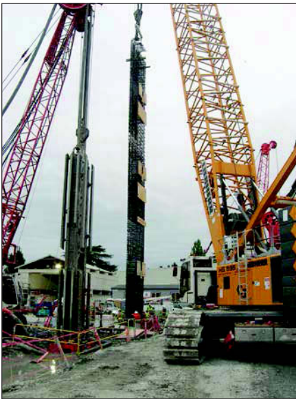
Figure 4. Typical reinforcing steel cage installation
