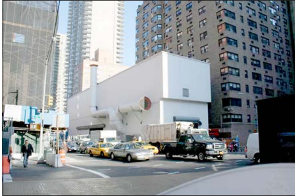
Figure 9. Muck enclosure at the 72nd Street shaft
