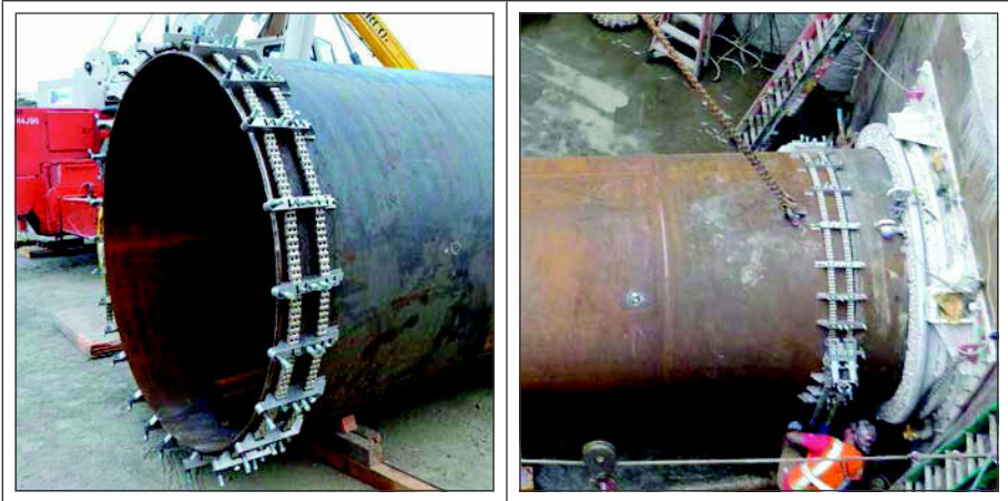
Figure 6. YLS casing fit-up using a double chain clamp
