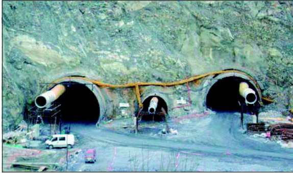
Figure 12. Pilot and evacuation gallery in Dos Valires (Andorra)
