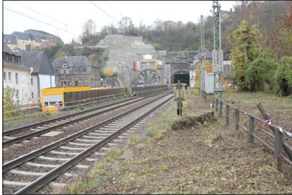
Figure 7. View of the New Kaiser Wilhelm Tunnel at Cochem portal (Source: ABT, 2011)
