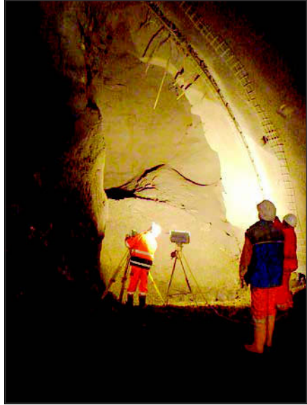
Figure 7. Surveying the void at TM 580.01 (Source: ABT, 2010b)
