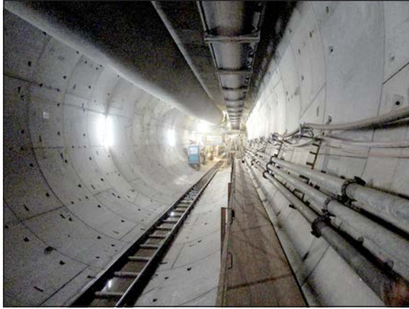
Figure 10. View into the tunnel showing the TBM back-up (Source: ABT, 2011)
