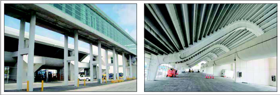
Figure 3: Pedestrian Bridge (left) and Shed #2 (right) on Dodge Island
