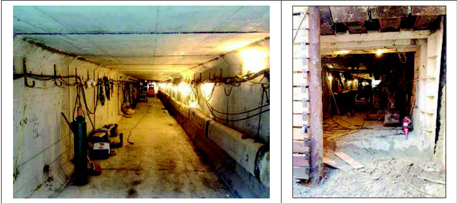
Figure 12. Completed culvert and break-through
