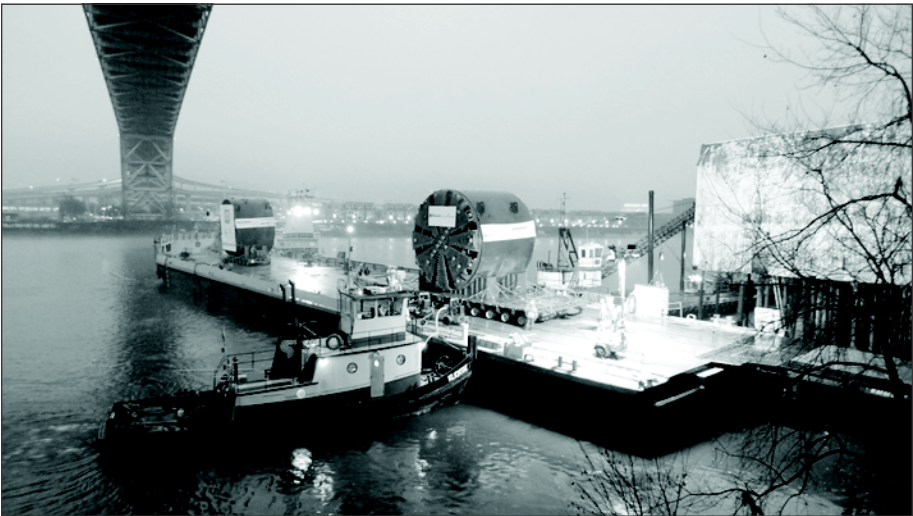
Figure 19. Barge loaded with the TBM and tailshield at the roll-on site
