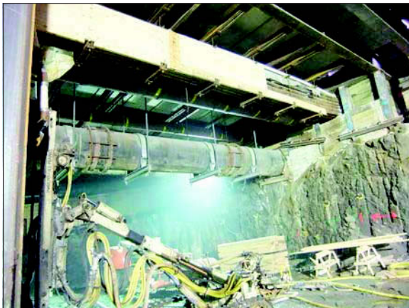
Figure 4. South shaft utilities being protected
