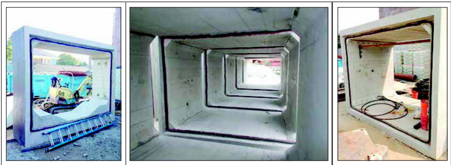
Figure 8. Box culvert [Type B]
