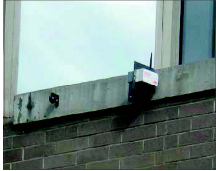
Figure 10. Combination prism and tilt meter on No. 7 Line project
