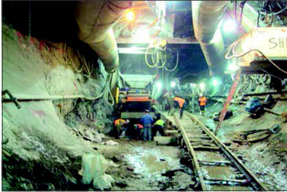
Figure 2. Crusher plant installation in a 3.5-ft deep pit
