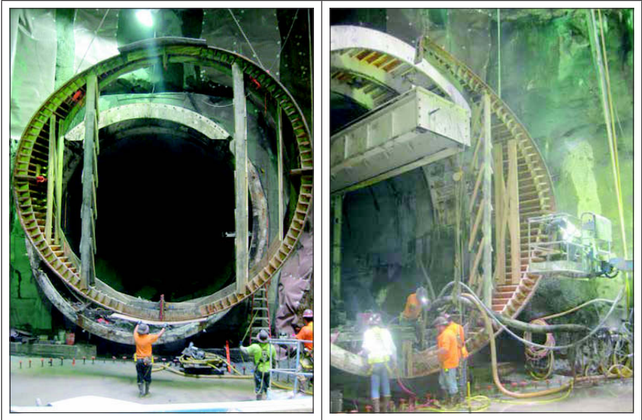
Figure 9. Junction form erection
