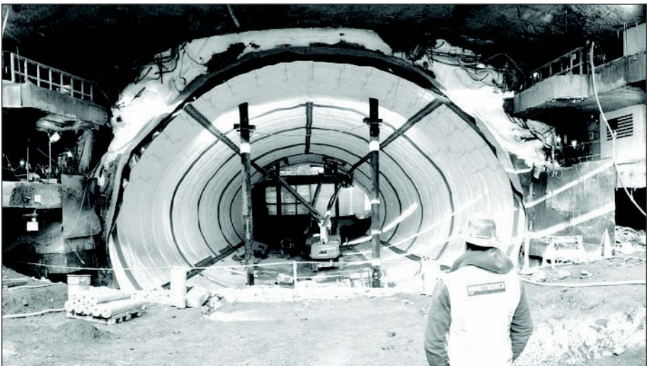
Figure 9. Completed tunnel with waterproofing installed. Note freeze visible around the edge.
