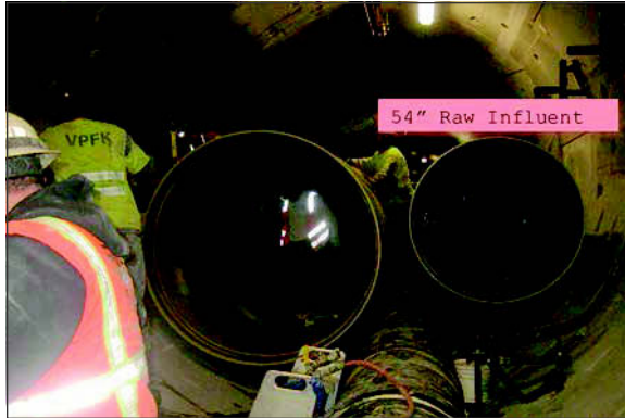
Figure 3. BT2 pipe install
