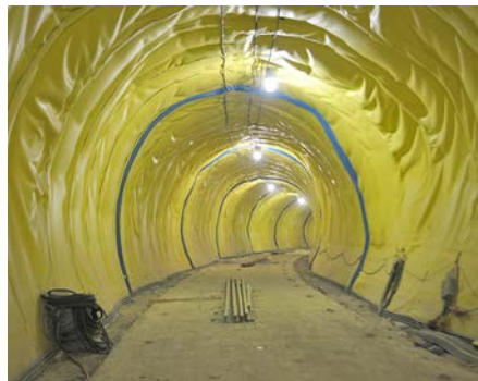
Figure 44. Completed waterproofing materials in the Horseshoe Tunnel, complete with water-barrier
