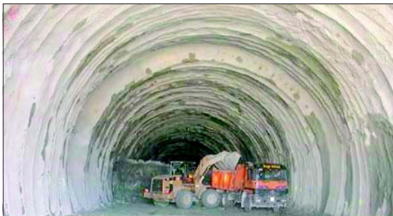
Figure 4. Bench excavation in road tunnel
