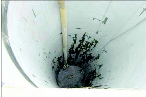
Figure 9. Looking down the completed South Shaft
