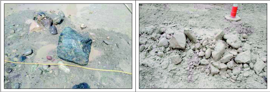
Figure 2. Cobbles and boulders encountered in panel excavation
