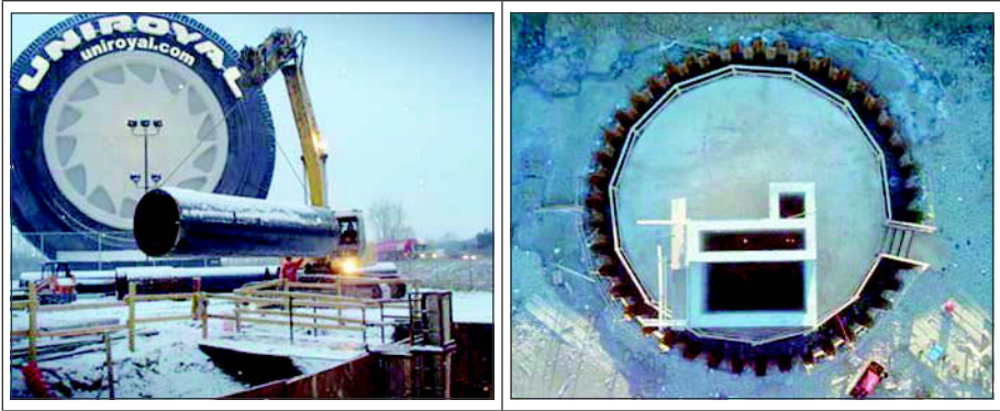
Figure 4. Each shaft location presents unique challenges
