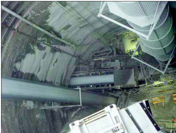
Figure 3. Conveyor installation in the shaft
