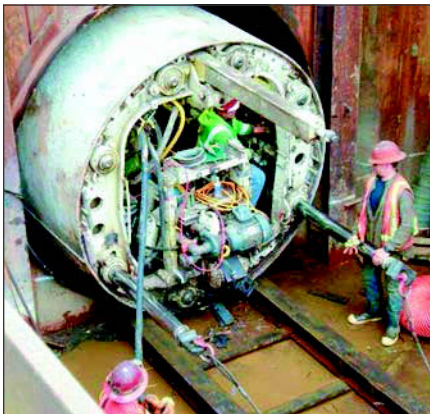
Figure 13. TBM after extraction from casing
