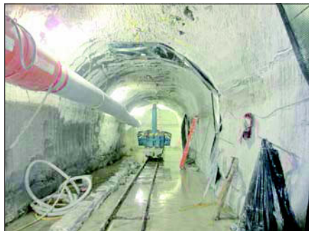
Figure 7. Reamer in suction chamber
