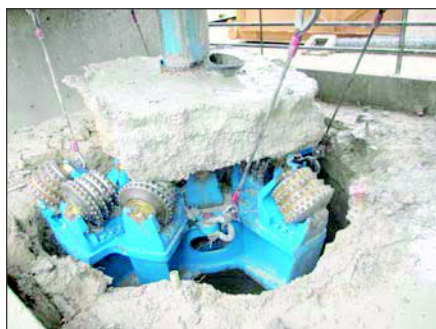
Figure 9. Reamer at ground level
