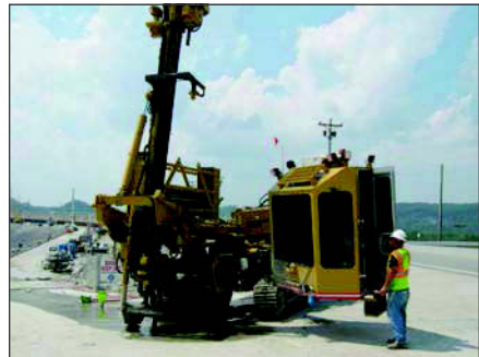
Figure 5. State-of-the-art drill rig used on the Thornton Shaft Grouting project
