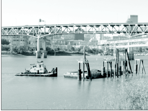
Figure 5. River barge for tunnel muck loadout
