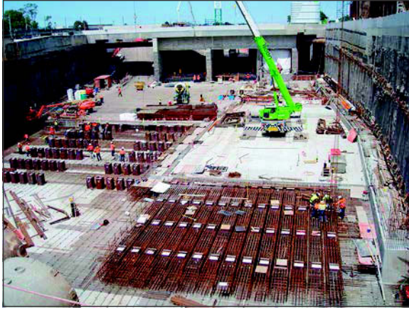
Figure 5. Jacking raft during construction showing shear pin recesses
