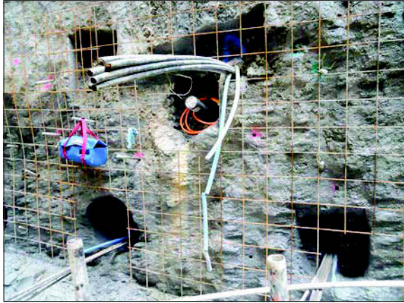
Figure 8. Horizontal extensometer on the East Side Access project
