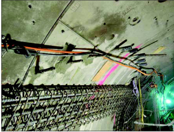
Figure 6. CP 19 pre support spiles above lintel cage
