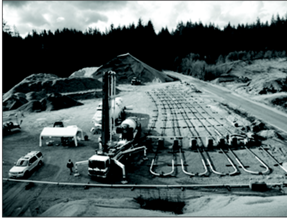
Figure 1. 700m long pumping test circuit using 5 inch dia. pumpline
