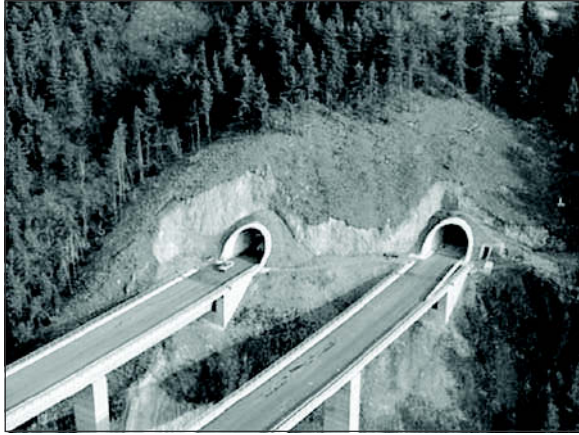
Figure 8. West portals of Donnersbergtunnel (Austria) (Courtesy of ILF Consulting, USA)
