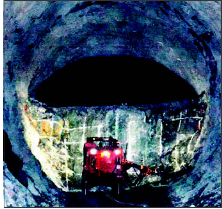
Figure 3. Top heading and bottom bench excavation
