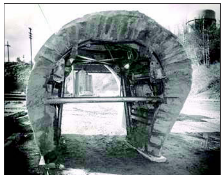
Figure 5. Portsmouth Tunnel open-face pneumatic shield (front view) in 1967 photograph
