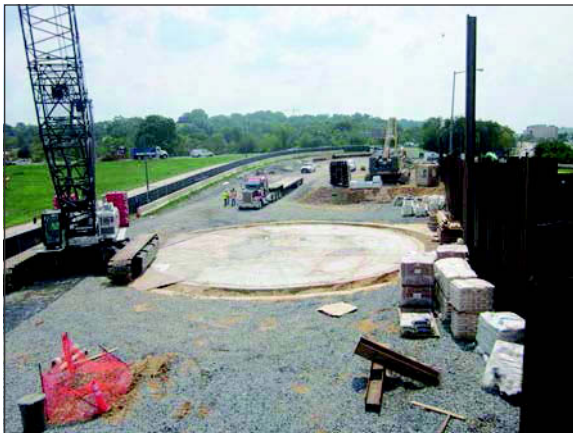
Figure 7. Poplar Point Junction shaft location, Fall 2012
