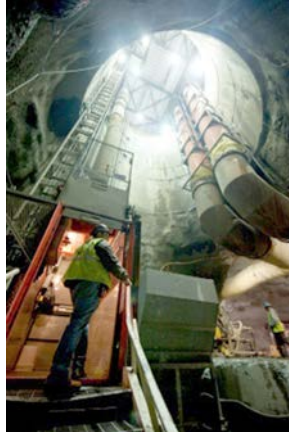
Figure 17. Looking up inside one of two construction shafts at the site
