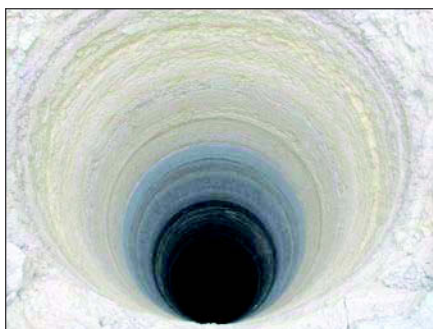
Figure 10. Completed well shaft
