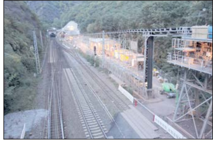
Figure 3. Site installation at the Ediger-Eller portal (Source: ABT, 2011)
