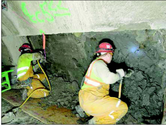
Figure 12. Hand excavation at cross passage 20
