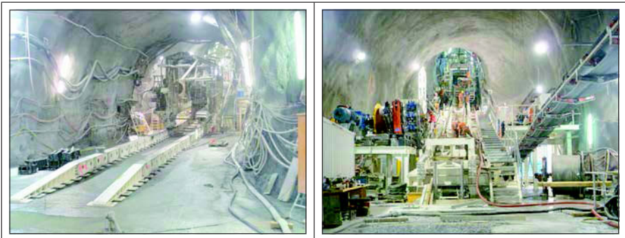
Figure 4. Ramp of 25° inclination—launch position for Gripper TBM
