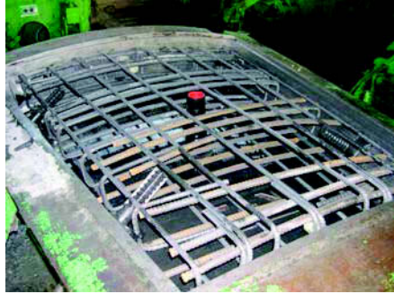
Figure 8. Reinforced steel cage for precast concrete segment
