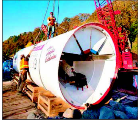
Figure 14. Herrenknecht open face digger shield with excavator arm
