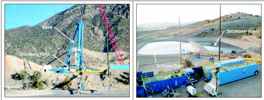
Figure 3. Blind drilling site
