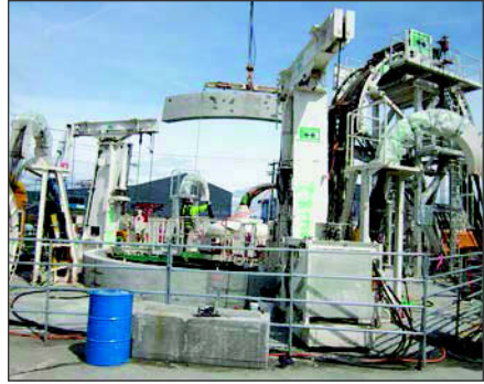
Figure 6. VSM excavation assembly winch (1 of 3)
