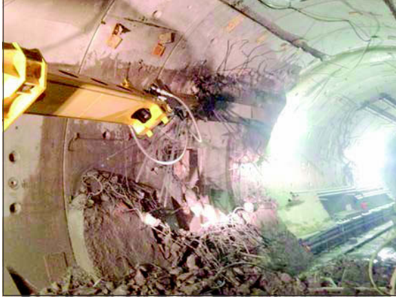
Figure 7. Lintel beam removal
