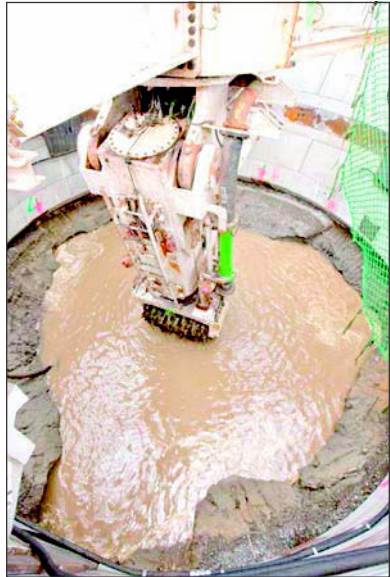
Figure 8. VSM excavation arm during calibration
