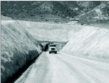
Figure 5. Box cut supported with shotcrete (Mexico)
