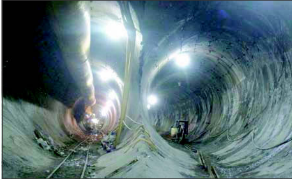
Figure 2. Narrow pillar on East Side Access (New York, NY)
