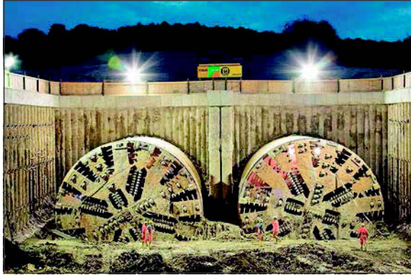
Figure 3. Katzenberg Tunnel, machines after breakthrough
