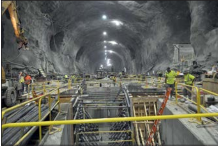
Figure 4. Main station cavern construction
