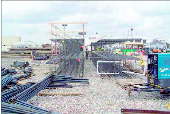
Figure 15. Rebar cage constructed
