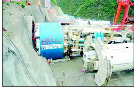
Figure 3. TBM launch
