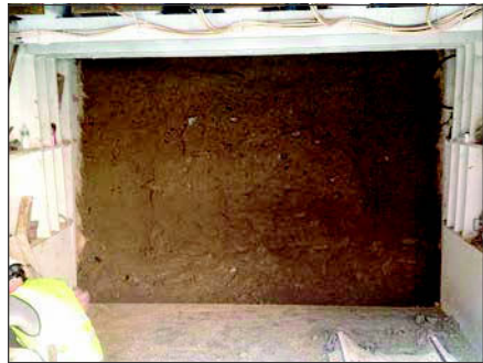
Figure 5. Typical ground type during mining
