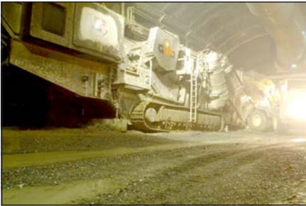
Figure 13. RPHT—Jaw crusher in the top heading area (Courtesy of Rowa, www.rowa-ag.ch )
