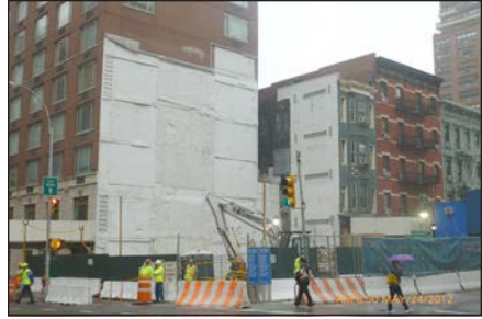
Figure 7. Tie-backs at Entrance 3
