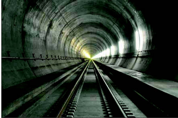
Figure 8. Completed tunnel Bodio-Faido West (Source: ABH, 2012)
