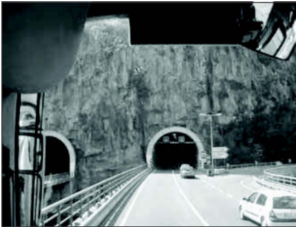
Figure 3. Rock blocks held with bolts (Madeira)
