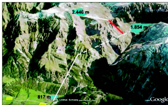
Figure 1. Aerial view of project area and 40° inclined pressure shafts marked in red
