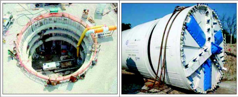
Figure 5. Secant pile shaft and TBM prior to insertion
