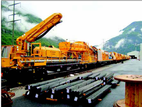
Figure 4. Concreting train (Source: ABH, 2010)
