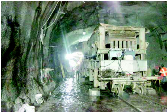
Figure 6. Fully assembled crusher plant on transporter frames and rail dollies
