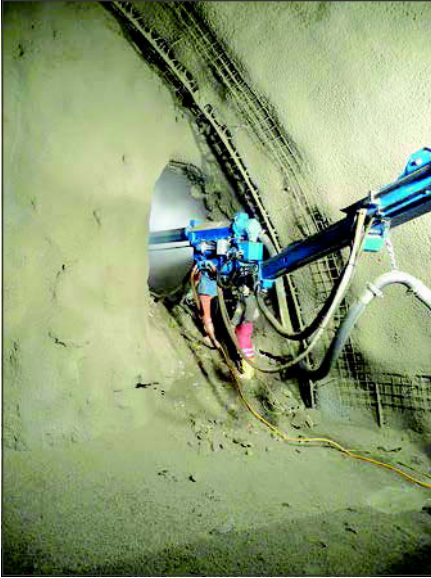
Figure 6. Sealing the opening and the void at TM 580.01 (Source: ABT, 2010b)
