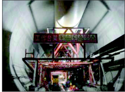
Figure 6. Continuous pour concreting behind the TBMs
