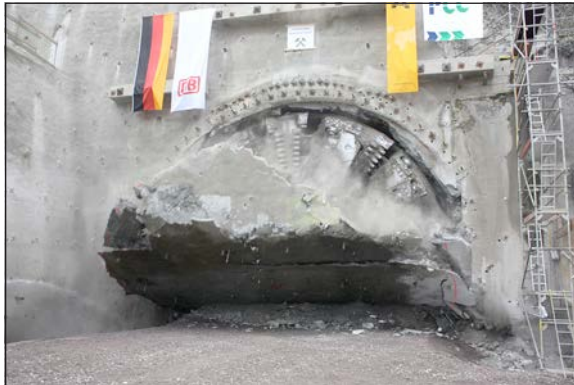
Figure 6. TBM breakthrough at the Cochem portal (Source: ABT, 2011)
