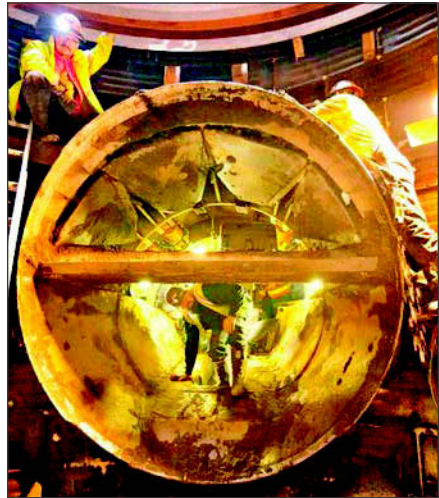
Figure 15. Digger shield after hole through at North Shaft
