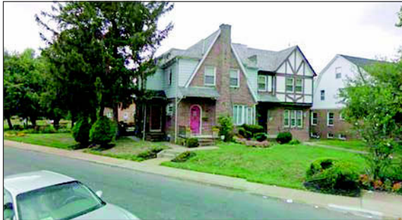
Figure 3. Alignment passes under residence in mixed-face conditions
