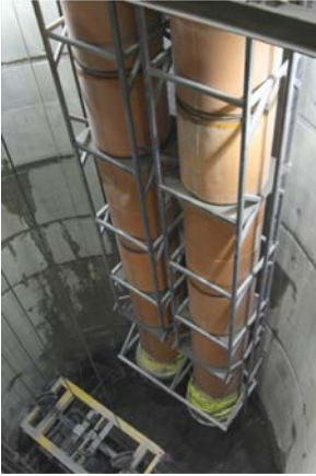
Figure 16. Interior view inside one of two construction shafts at the site
