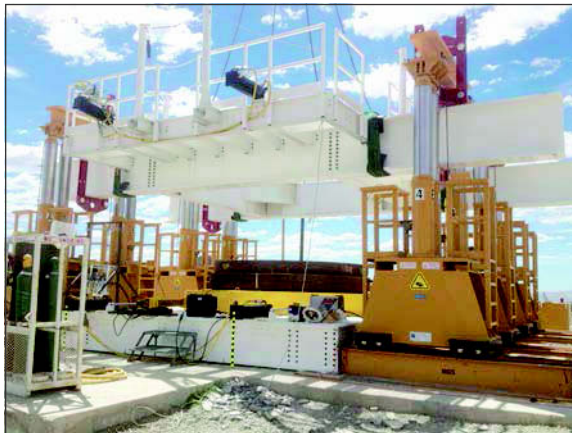
Figure 8. Liner installation system
