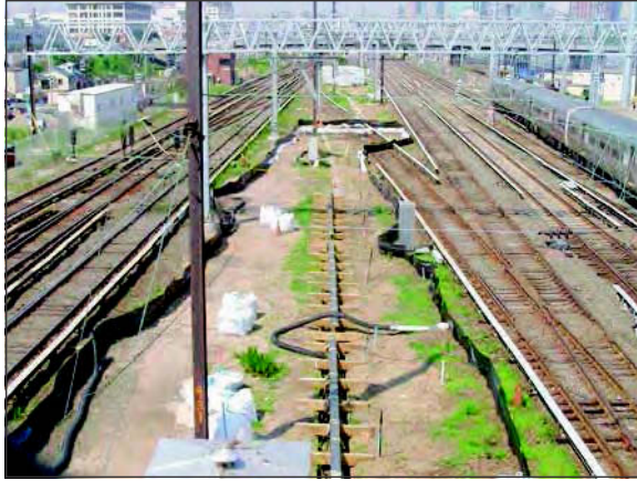
Figure 20. View of surface clean-up system and suspended cable trough
