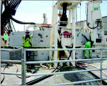
Figure 5. VSM hydraulic caisson jack (1 of 4)
