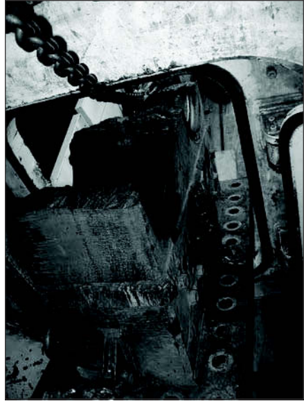
Figure 13. Moving the yoke through the manlock
