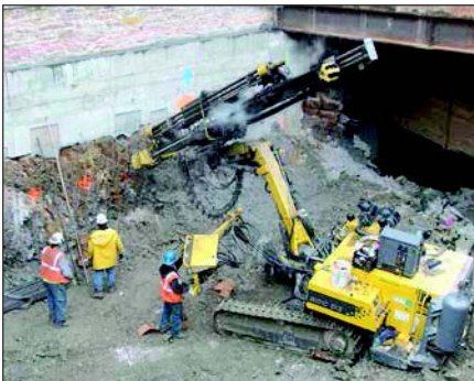
Figure 10. Rock bolting with D3
