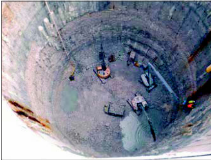
Figure 5. Main gate shaft during excavation
