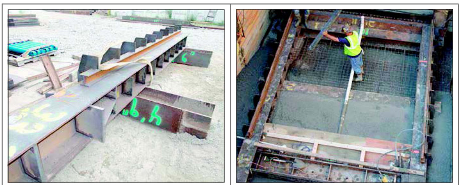
Figure 10. Thrust block fabrication and installation
