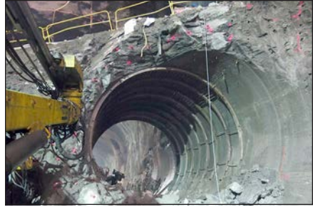
Figure 5. Excavation of the TBM tunnel as part of cavern construction
