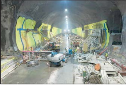
Figure 10. Main station cavern— waterproofing and concrete lining work
