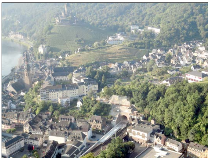
Figure 1. View of the portal of the New Kaiser Wilhelm Tunnel in Cochem (Source: ABT, 2012b)
