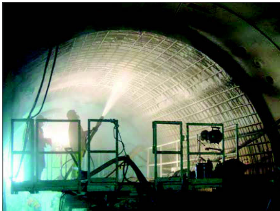
Figure 5. Placing dry mix shotcrete in crown
