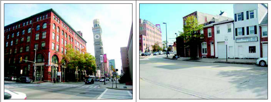
Figure 5. Narrow right-of-ways with adjacent historic sensitive structures
