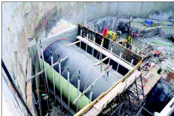
Figure 9. Construction of launch blocks showing vertical and horizontal tie rods
