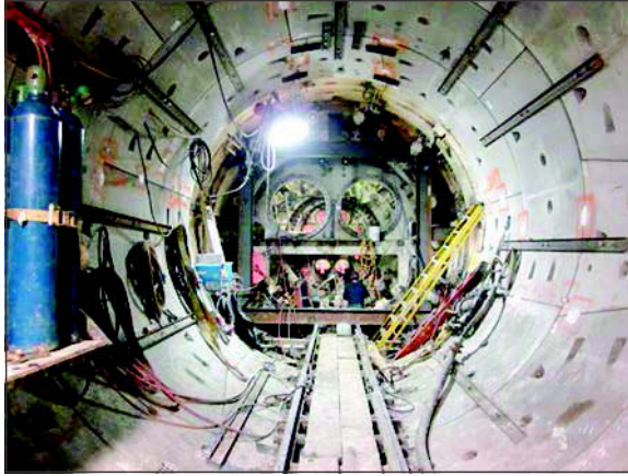
Figure 5. Temporary bracing installed
