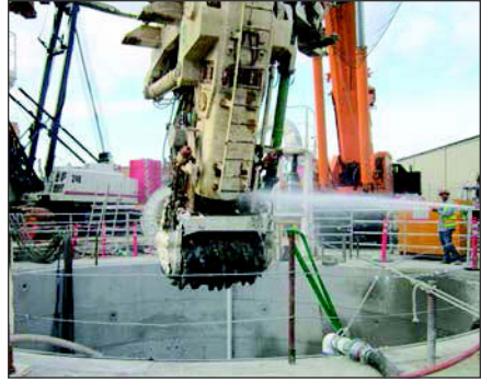
Figure 4. VSM excavation cutterhead
