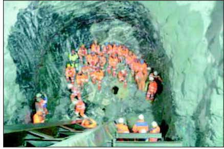
Figure 8. Breakthrough after first drive
