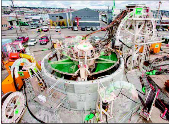
Figure 2. Herrenknecht VSM machine at the BSRP South Shaft
