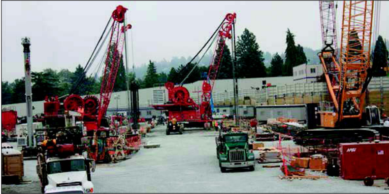
Figure 3. Fully mobilized site in action
