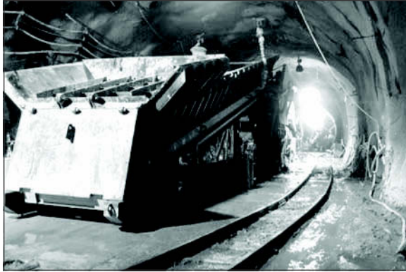
Figure 8. Final muck conveyance system at flight conveyor feed point
