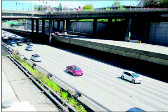
Figure 1. I-5 Freeway at undercrossing (looking North-Northeast)
