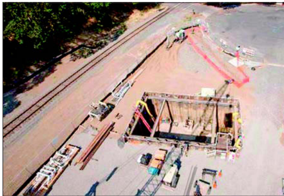
Figure 2. Aerial view of south portal shaft and railroad crossing
