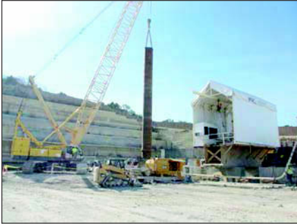
Figure 11. Well casing installation
