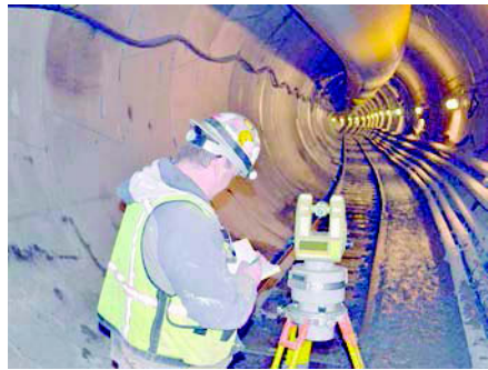
Figure 10. Gyro-theodolite observations in the BT-3 Tunnel using the DMT Gyromat 2000
