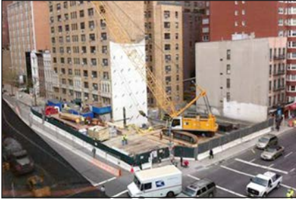
Figure 6. Tie-backs at Ancillary 2
