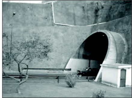
Figure 2. Concrete canopy, bolts, and shotcrete (Madeira)
