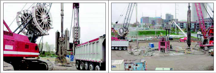
Figure 3. Diaphragm wall panel excavation
