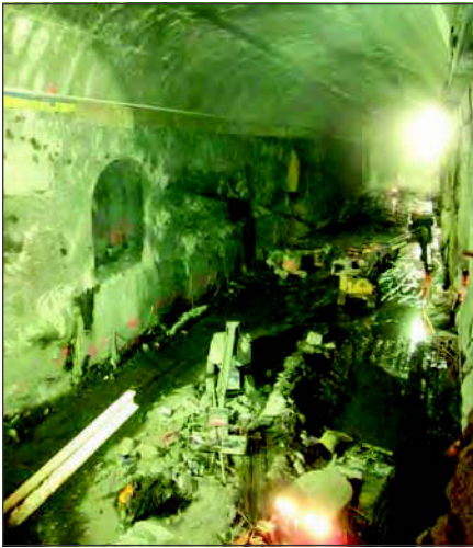
Figure 10. Benching down to full cavern depth
