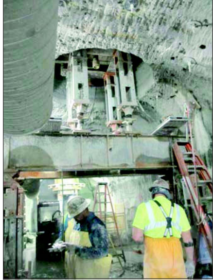
Figure 15. Lower falsework in suction chamber
