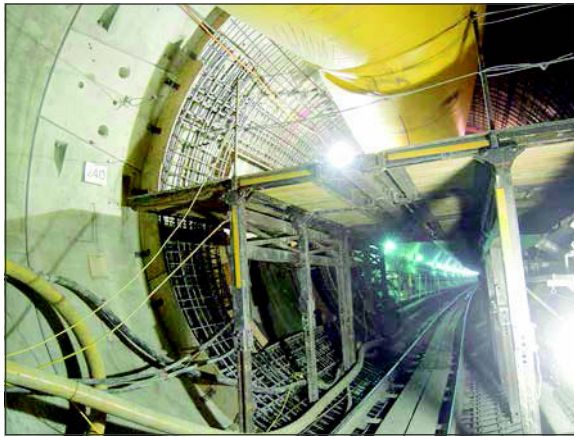
Figure 11. Completed propping reinforcing and formwork with work deck in place
