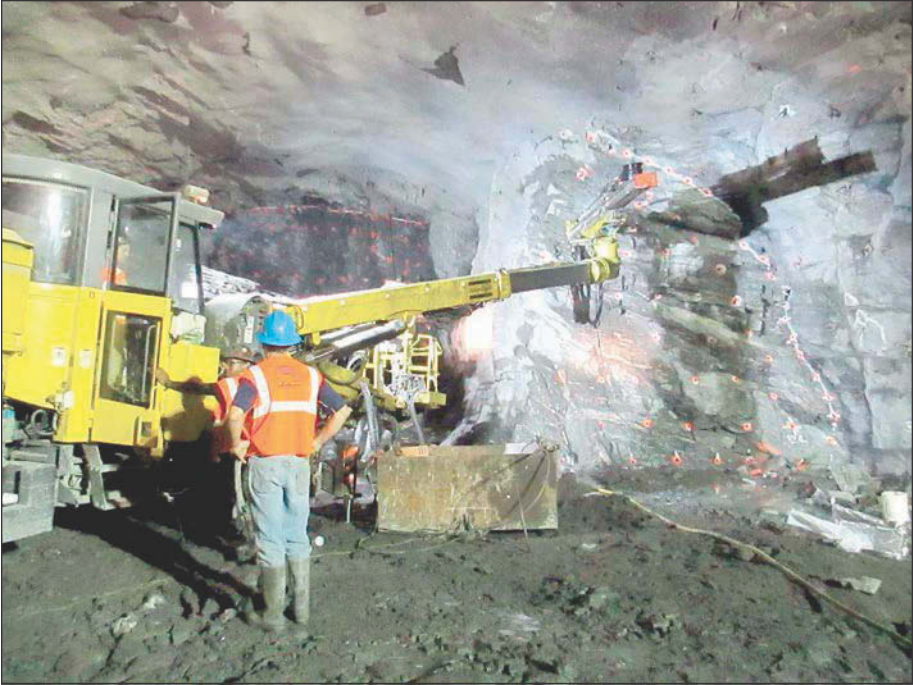
Figure 4. Drill-and-blast excavation of cavern top heading
