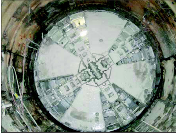
Figure 12. Breakthrough of the BT3C TBM inside the larger-diameter BT3 shield
