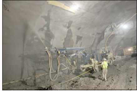
Figure 11. Shotcrete initial support
