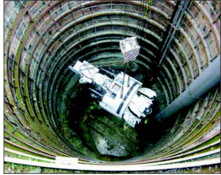
Figure 6. TBM cutterhead and support lowered into shaft
