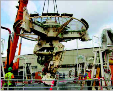
Figure 3. VSM excavation assembly
