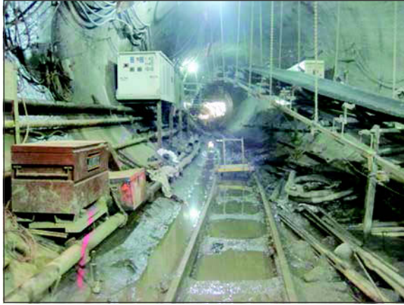
Figure 5. Crusher branch belt existing crusher pit on a twelve-degree incline
