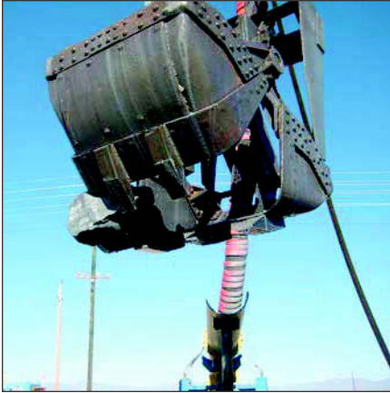
Figure 6. Clamshell used to remove broken cutter
