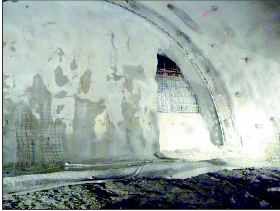
Figure 9. Closing the void at TM 580.01 (Source: ABT, 2010b)
