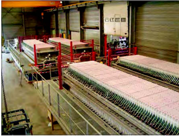
Figure 14. MS STP filter presses
