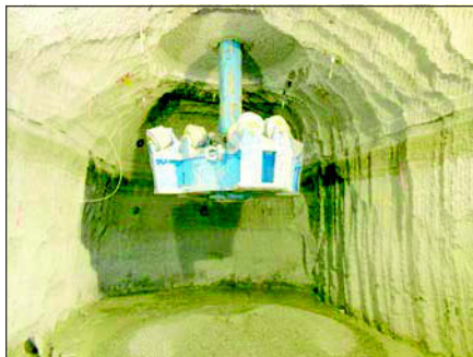
Figure 8. Starting reaming operations
