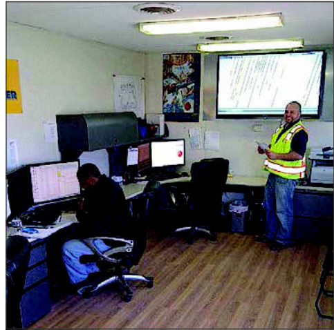
Figure 7. On-site iGrout monitoring station
