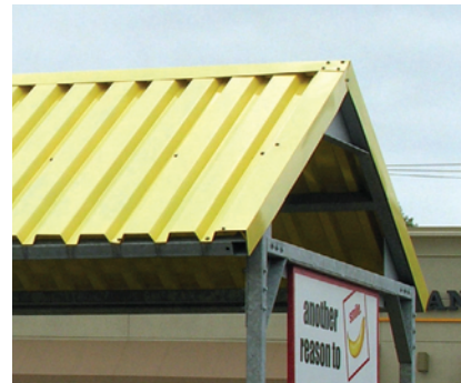
CORRUGATIONS in nature (top) and in everyday objects (bottom) are smart examples of structures that would otherwise require more material for support.
