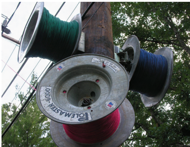
TENSION ROPE DRUM. Ropes for pulling high-wattage conductor cables are made from strong nylon.
