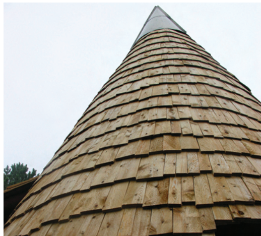
ROOF SHINGLES. Most wood-shingled roofs are made from western red cedar. Wood shingles provide air circulation and weather resistance.
