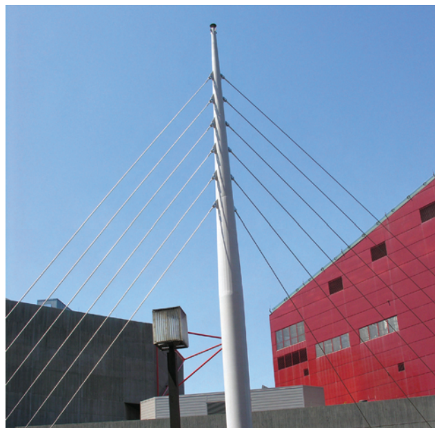
CABLE BRIDGE. Tension structures are strong and light.
