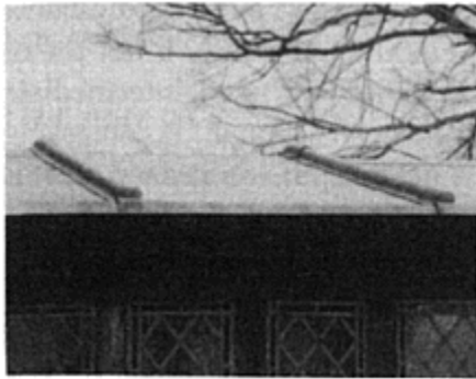
Fig. 2.4 A sheet lead roof covering showing how the sloping long edges of the units are connected and weatherproofed by being lapped over wooden rolls.
