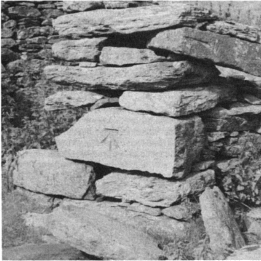
Fig. 3.8 An Ordnance Survey Bench Mark (OSBM) cut into the wall of a derelict shieling to the west of Ben Lawers in the Grampian Mountains in Scotland. Its altitude is 505.24 m above the mean sea level at Newlyn, some 500 miles away.
