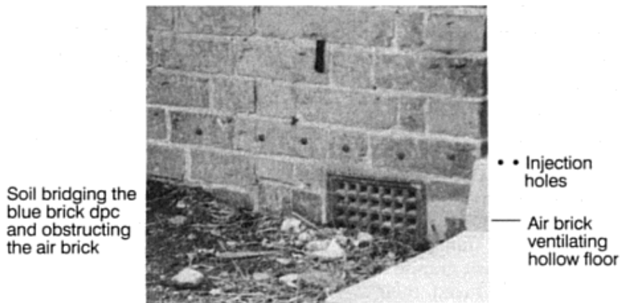
Fig. 2.7 Visible evidence of an injected chemical dpc in an external wall. Also, a ventilation inlet to a hollow floor, and a soil-bridged blue brick dpc.
