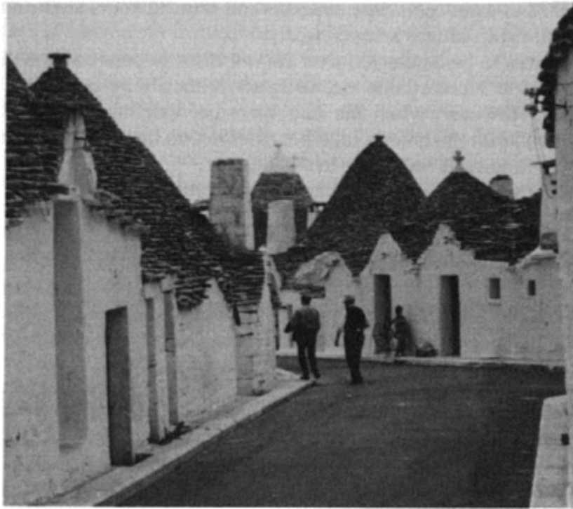
Fig. 3.2 A street in Alberobello, Italy, showing trulli constructed of small pieces of limestone bedded in mortar. rafters . In a floor or ceiling they are called joists , and in a wall or partition, they are called studs . Although made mainly of wood, metal sections may be used. The members are connected to form a frame by either:
