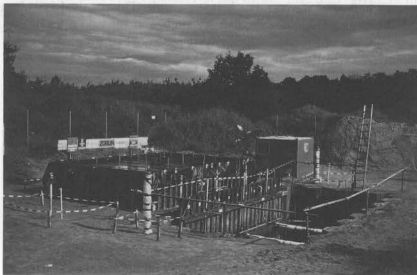
Figure 6.26 The construction excavation at the test site
