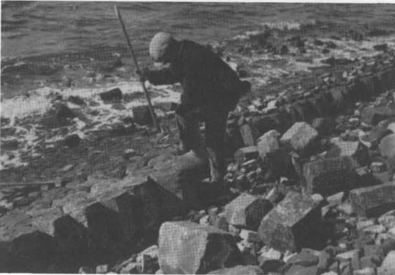
Figure 5.2 Construction of a block revetment on the Afsluitdijk, near Kornwerderzand (1927), © municipality of Wieringen
